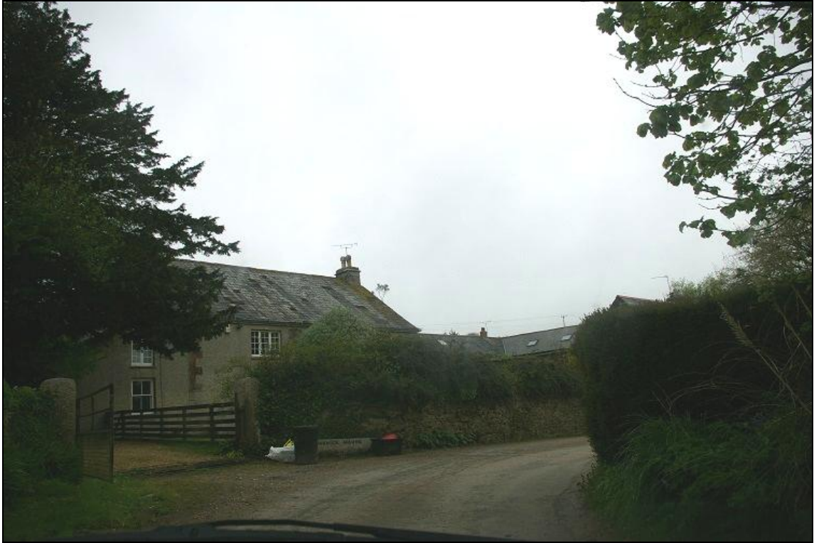
View of Gwarnick Manor, which lies 1km south-east of the proposed turbine. The turbine will appear to the north-west, behind the house. There is also blocking from the topography, hedge-banks and outbuildings; viewed from the south-east.
