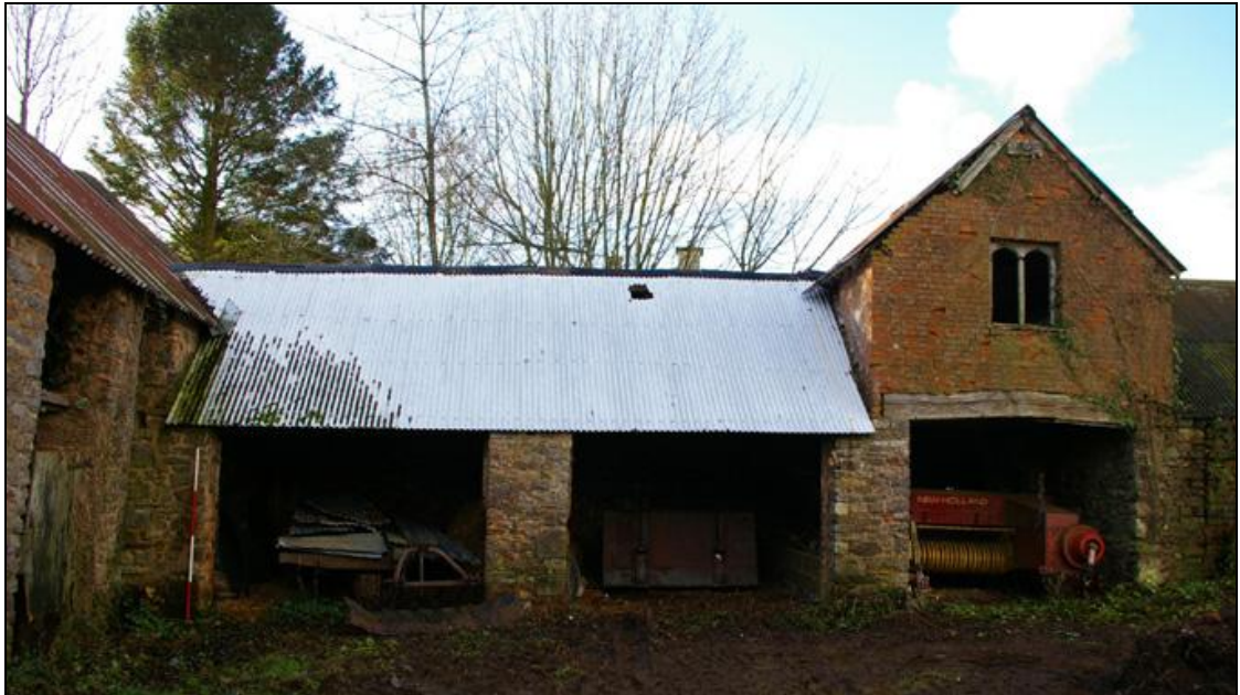
Figure 20: The east elevation of Buildings 7 & 8, viewed from the east (2m scale).
