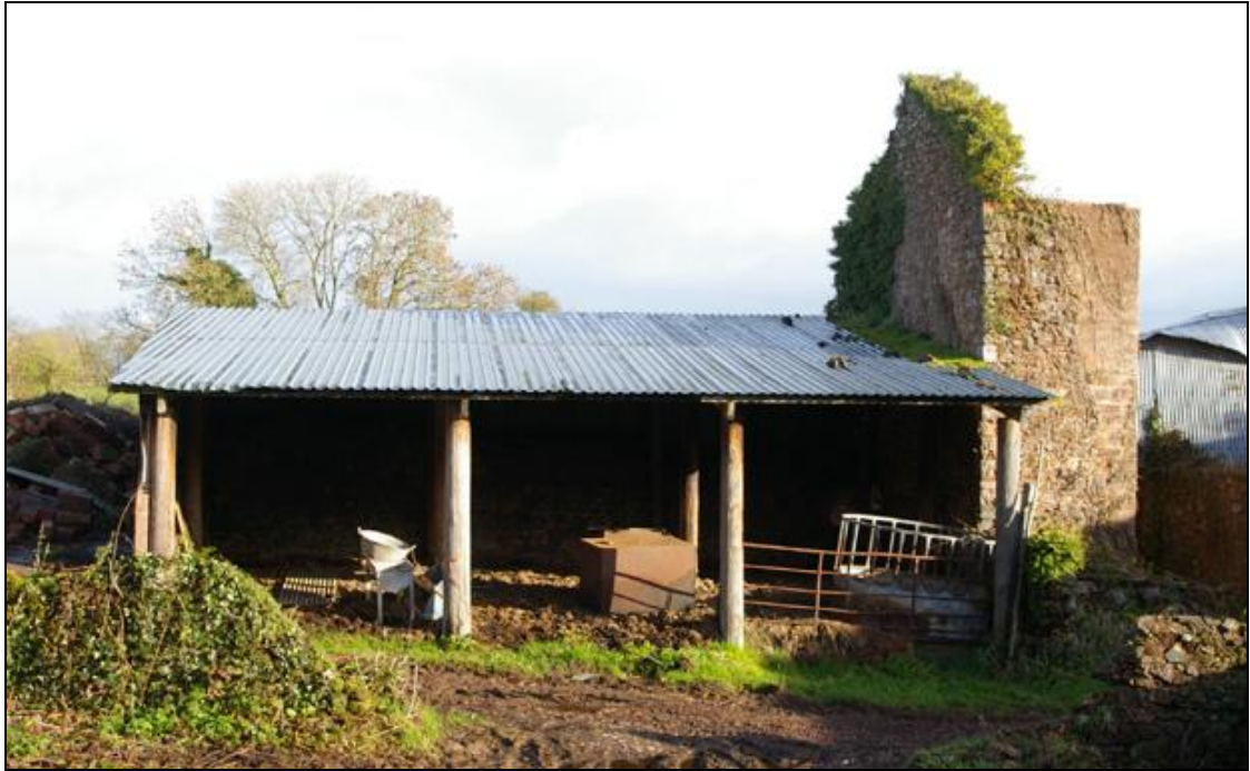
Figure 10: The west elevation of Building 4, abutting Building 5 to the south, viewed from the west.
