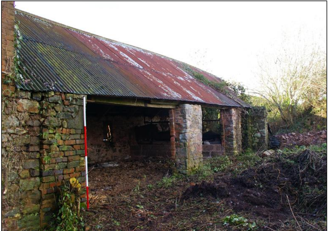
Figure 21: East elevation of Building 9, viewed from the southeast (2m scale).
