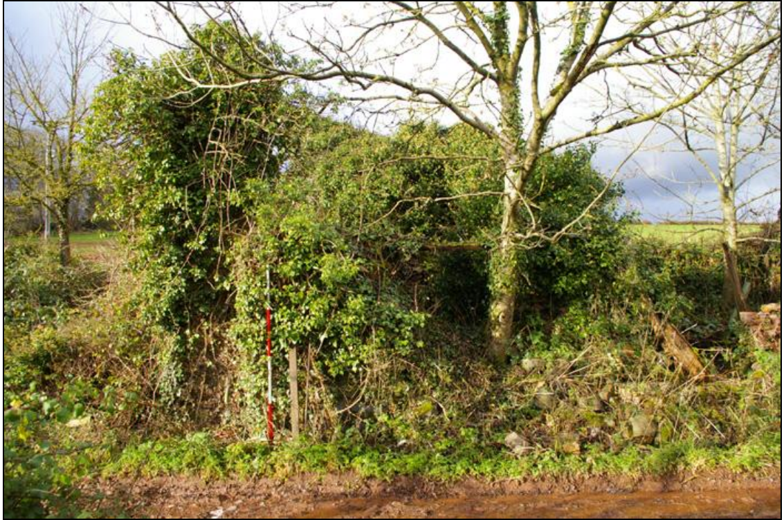
Figure 9: The south elevation of Building 3, viewed from the south (2m scale).
