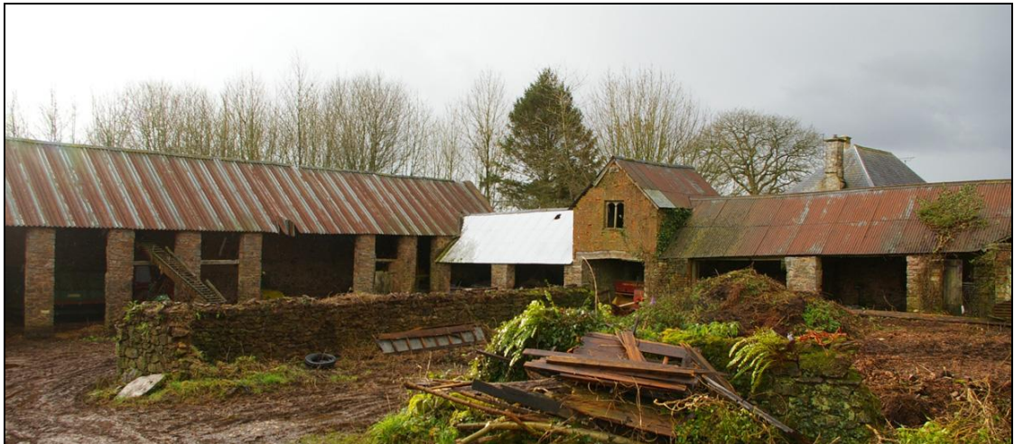
Figure 6: Buildings to the south-west of the courtyard, viewed from the north-east.
