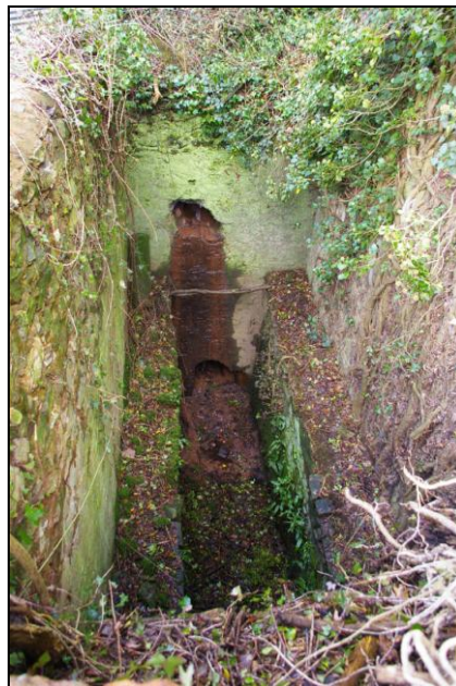
Figure 15: The view into the wheel pit.
