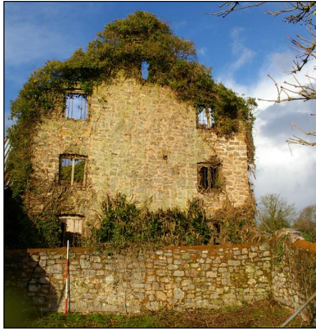
Figure 14: The south elevation of Building 5, with wheel pit, viewed from the south (2m scale).
