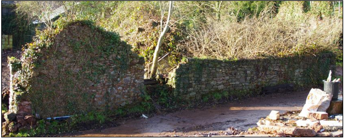
Figure 22: Ruins of Building 10, viewed from the east.
