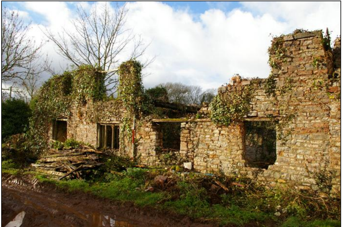
Figure 8: The south elevation of Buildings 2 & 3, viewed from the south-east (2m scale).
