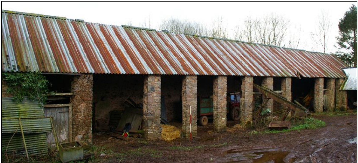
Figure 16: The eastern end of Building 6, viewed from the north-east (2m scale).
