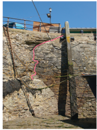
The later wall appears to overlap the highlighted area suggesting that this represents an extension to the older pier end.
