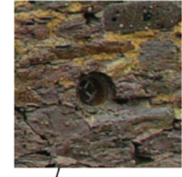
The weepholes used to reduce the consequences of tidal pressure on the outer harbour-side wall.
