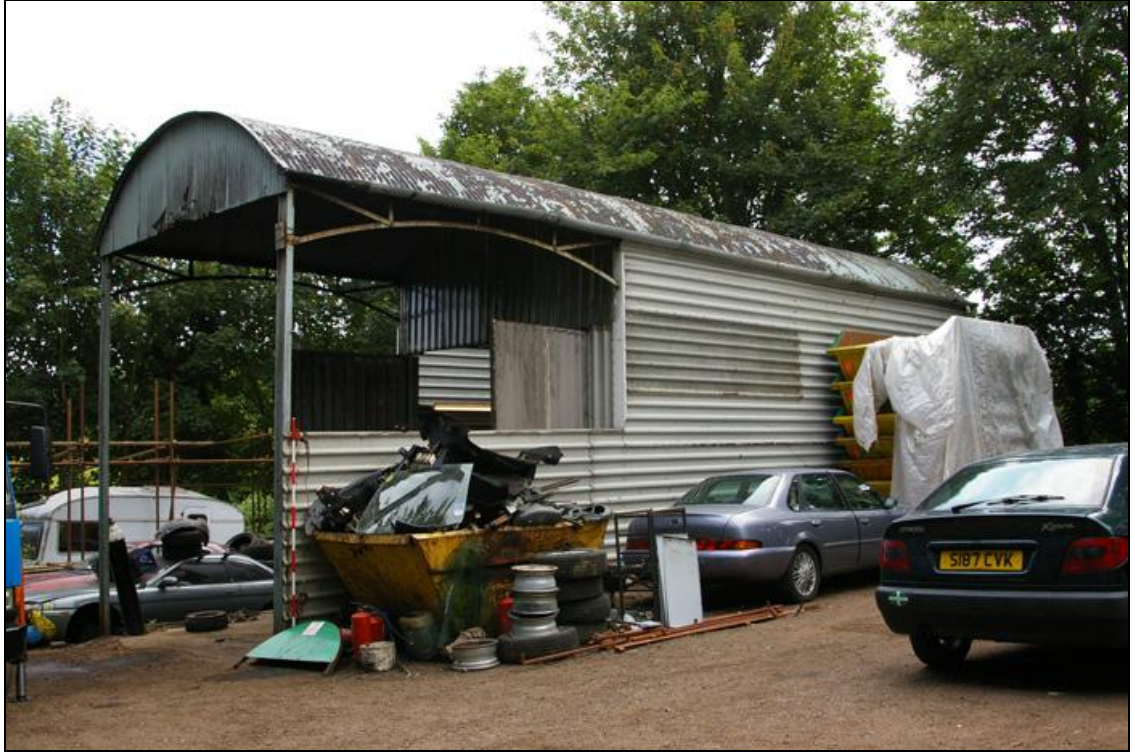
Figure 28: Building 8, viewed from the north-east (2m scale).
