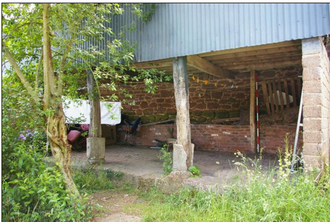
Figure 16: The north front of Building 3a – Linhay, viewed from the north-west (2m scale).
