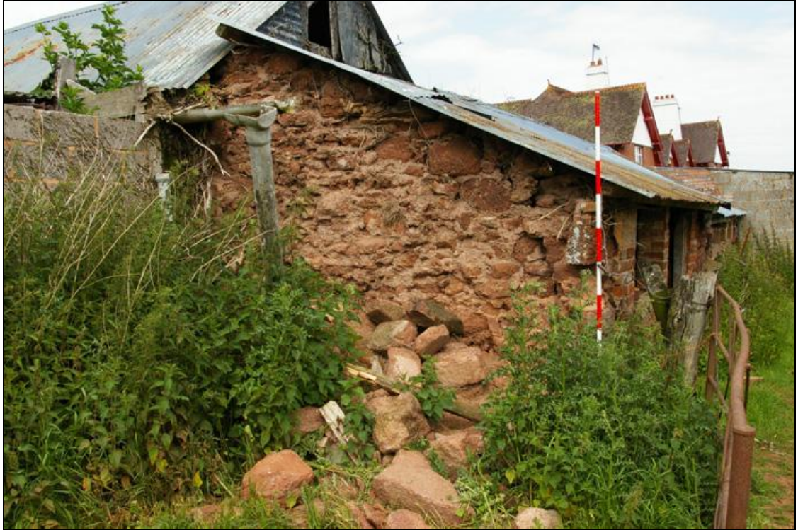
Figure 22: Exterior south wall of B5, viewed from the south (2m scale).
