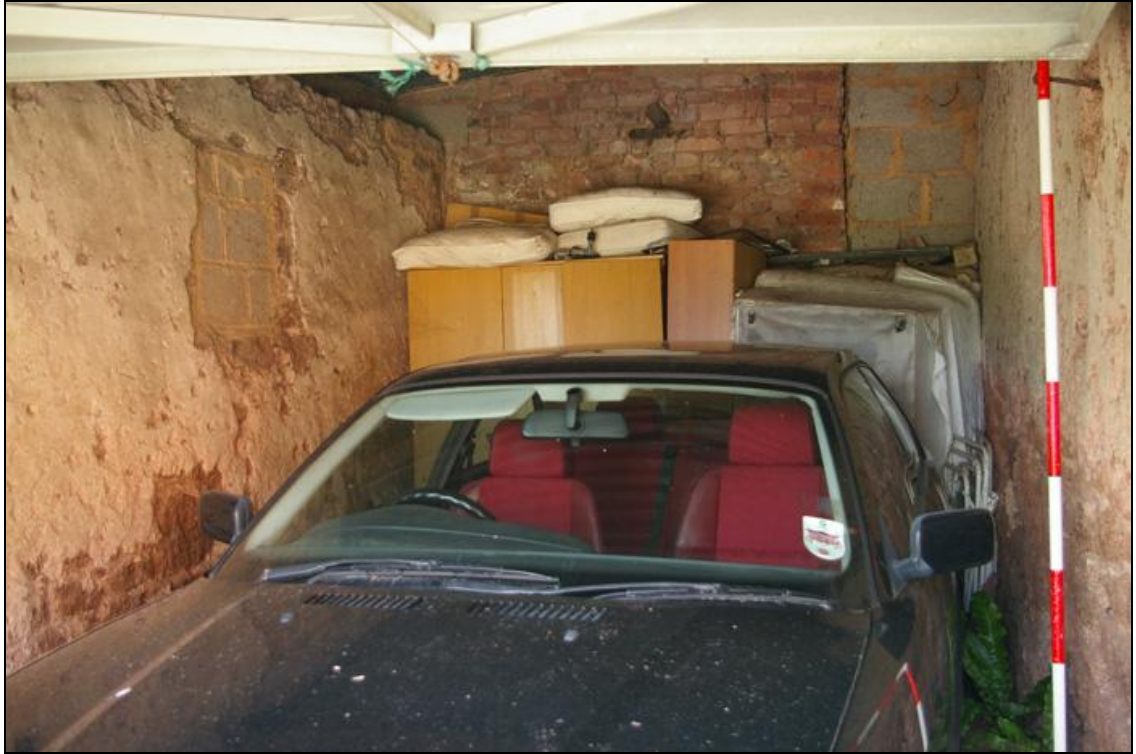
Figure 25: The interior of B6; the north-western garage compartment, viewed from the north (2m scale).
