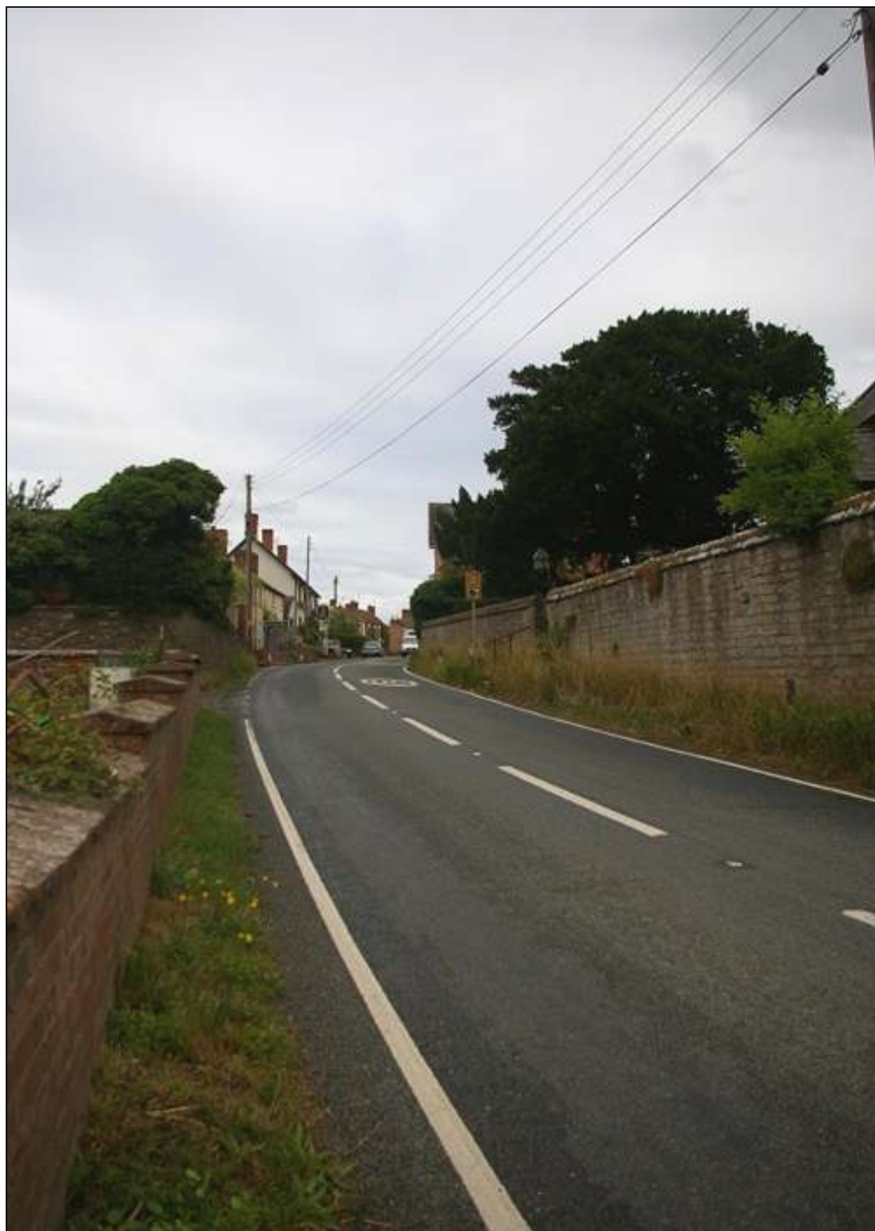
View along the main road in Lyng, showing houses and buildings, which provided some local blocking to the church; from the west.
