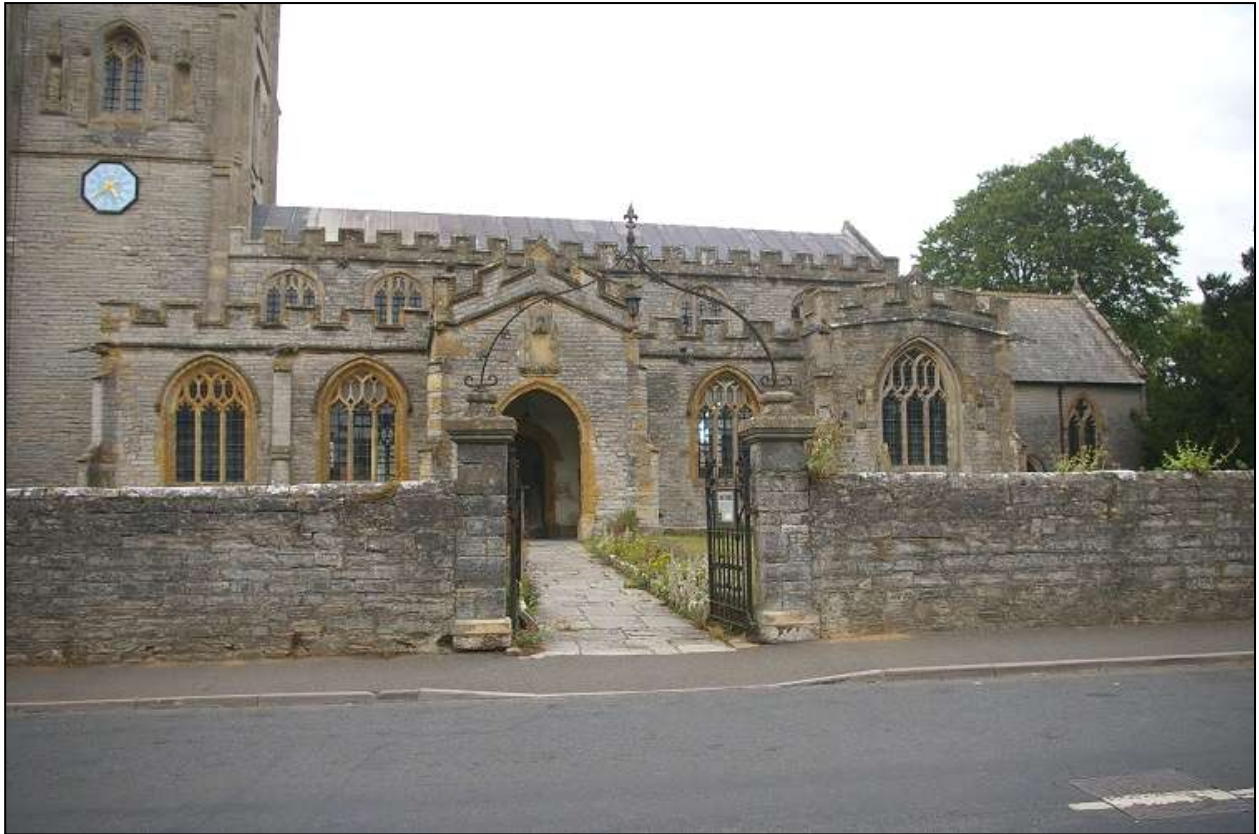
View of the Listed churchyard wall and gates into St Mary the Virgin, Westonzoyland; from the south-west.
