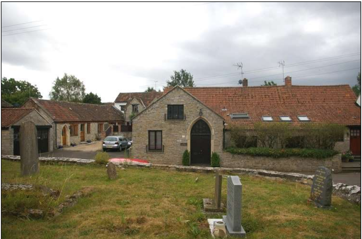
Local blocking which affects Stawell Church; from the north.
