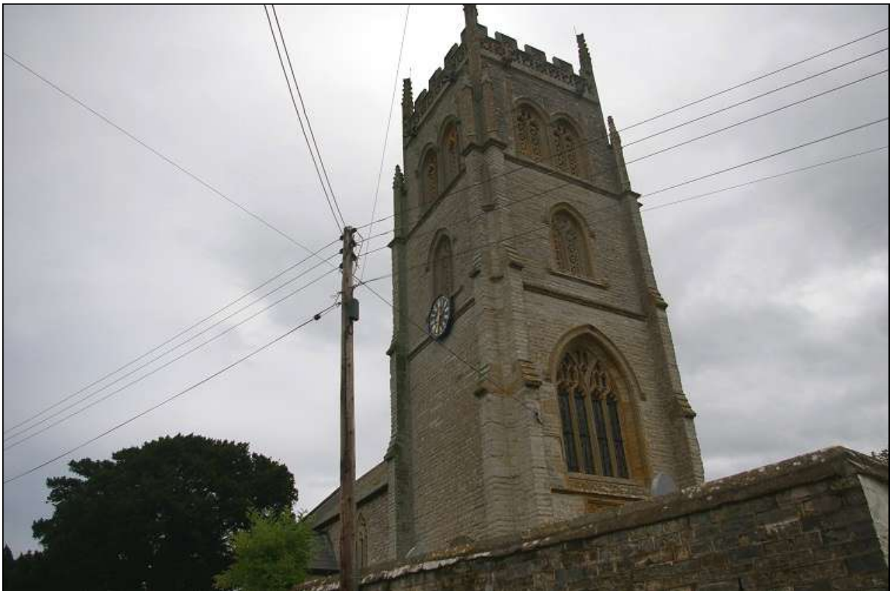
St Bartholomew's Church in Lyng, with its tall church tower giving some views north; from the north-west.
