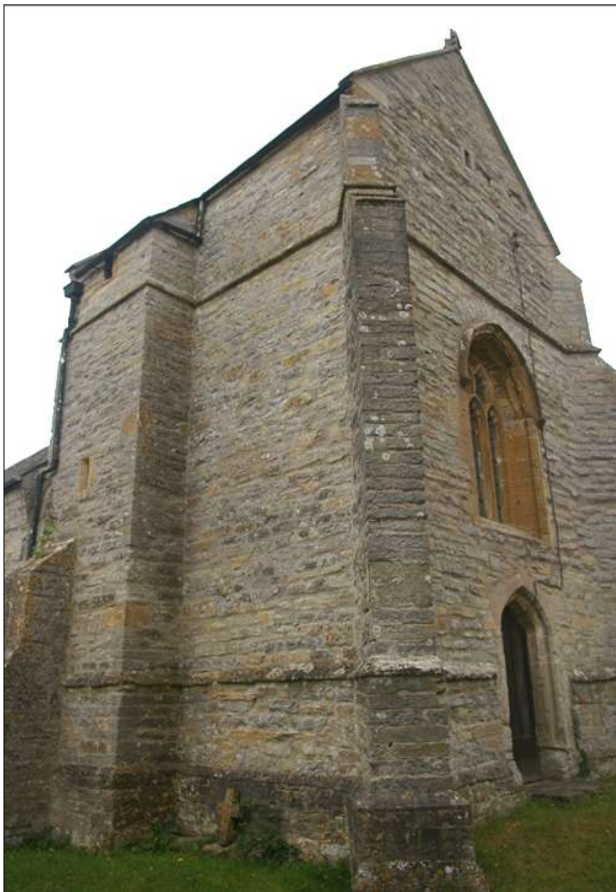
Stawell Church with its small squat tower; from the north-west.
