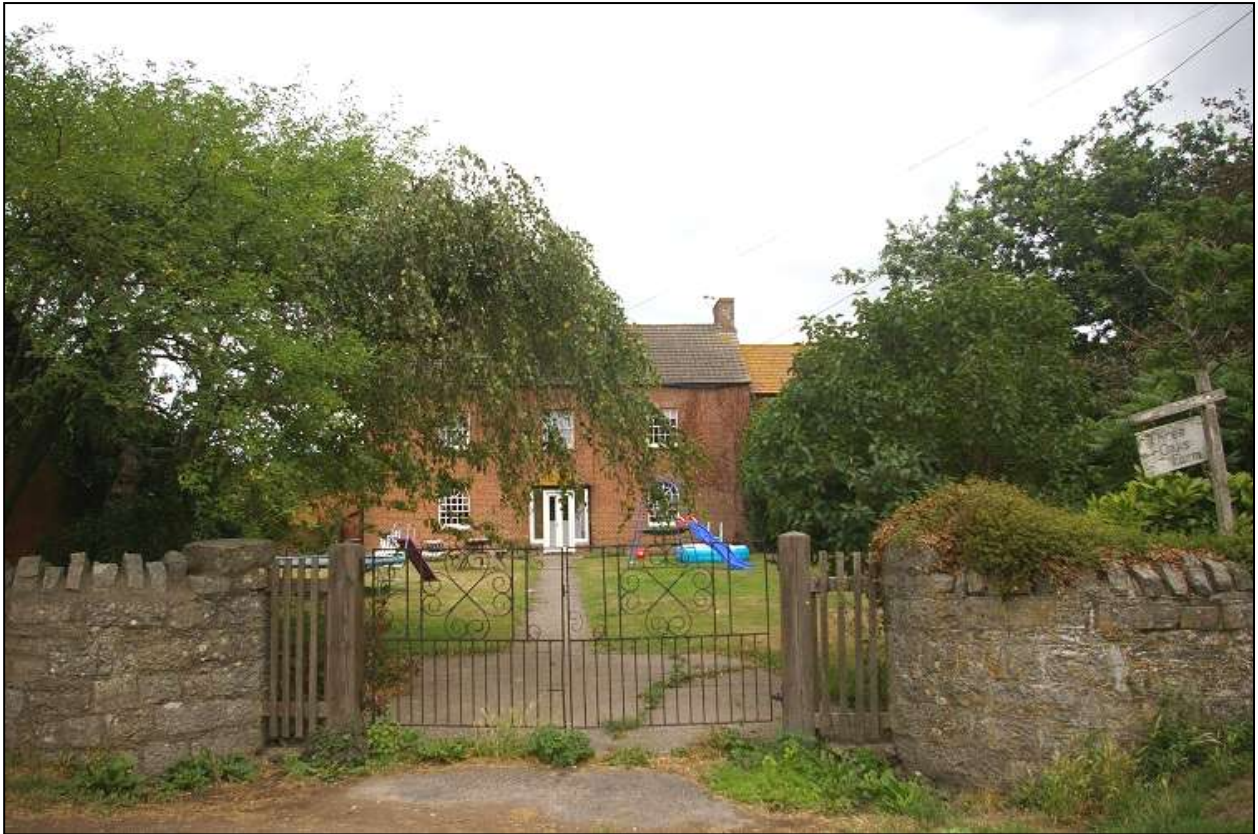
View of the frontage of Three Oaks Farmhouse, showing how the views are restricted by the surrounding barns; from the west.
