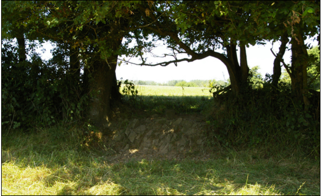
Figure 7: A section of stone revetment within the eastern boundary of F1 (western boundary of F2), viewed from the west.
