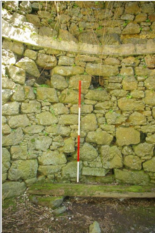
Figure 7: The cavities in the east wall, viewed from the west (2m scale).
