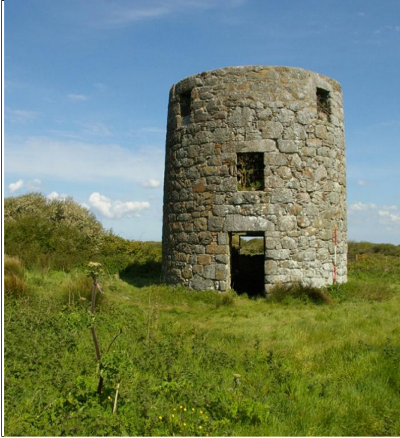
Figure 2. The windmill viewed from the south, showing the opposing door openings and south, east and west window openings (2m scale).
