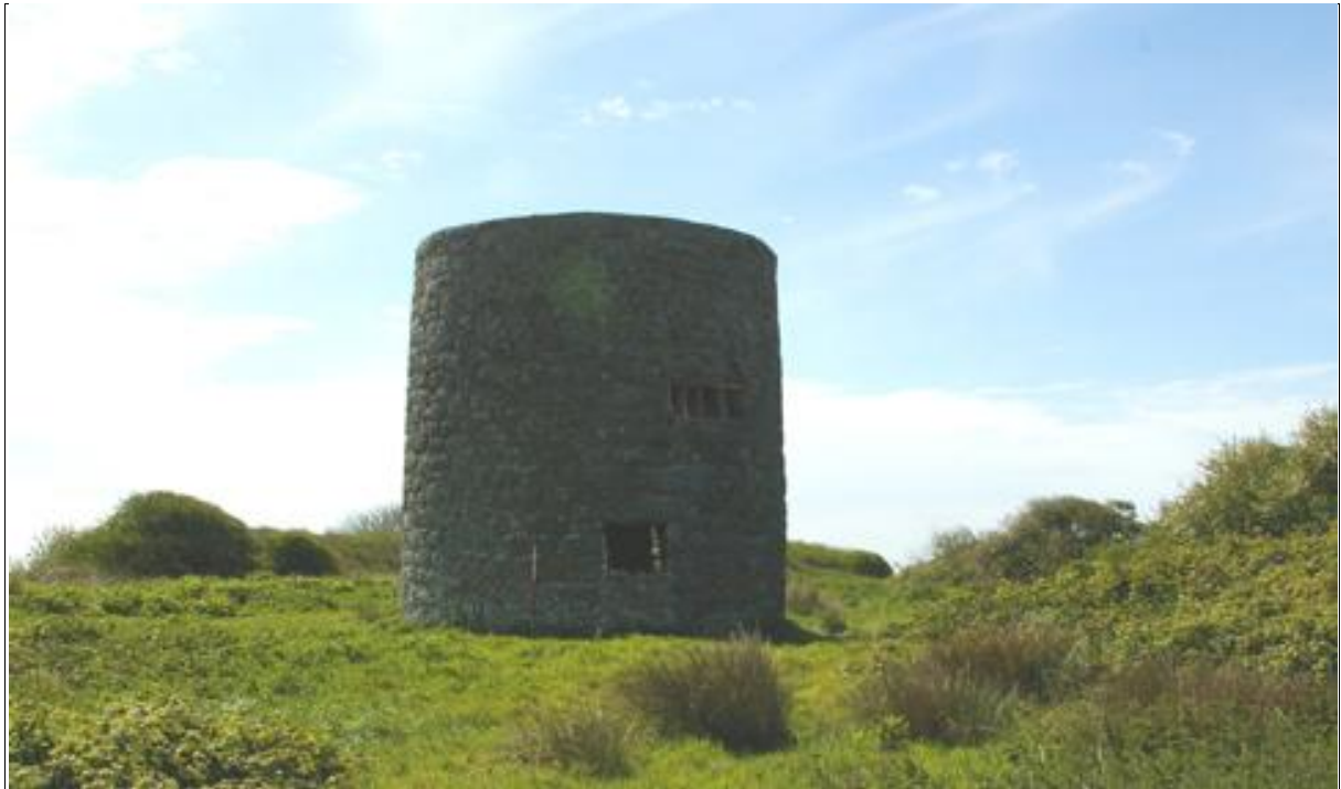
Figure 12: The windmill, viewed from the north (2m scale).
