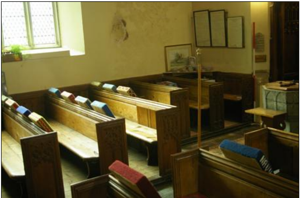
Figure 6: The south-west corner of the nave (south aisle), showing the pews to be removed under the current proposals, viewed from the north-east.
