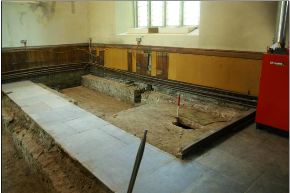
Figure 11: The raised arch of the vault below the seating areas within 'Martha's Corner', viewed from the south-east (2metre scale).
