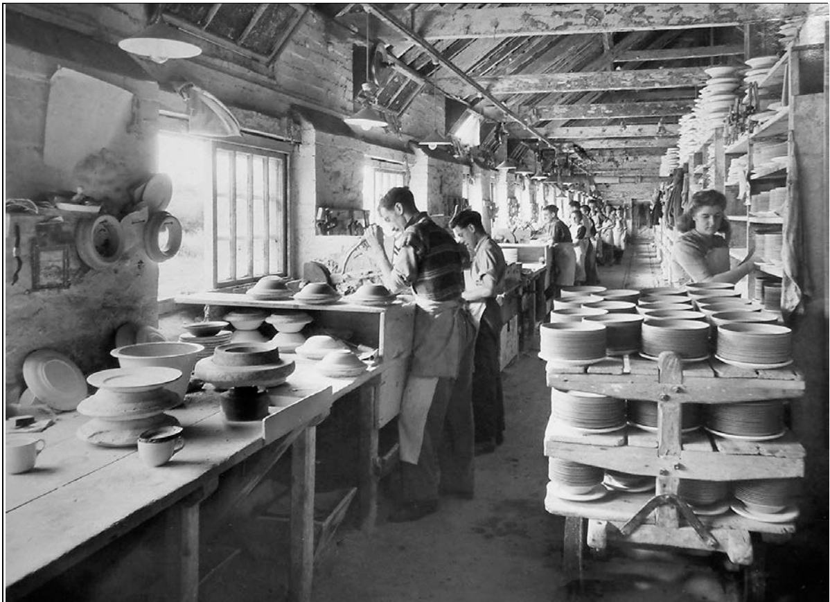
Figure 2: The Steam Shop (Flat) (Building 1) in 1947, viewed from the south (courtesy B. Adams).
