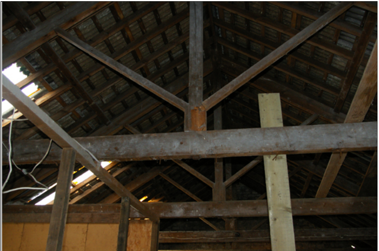
Figure 34: King post roof structure over B2, viewed from the east.
