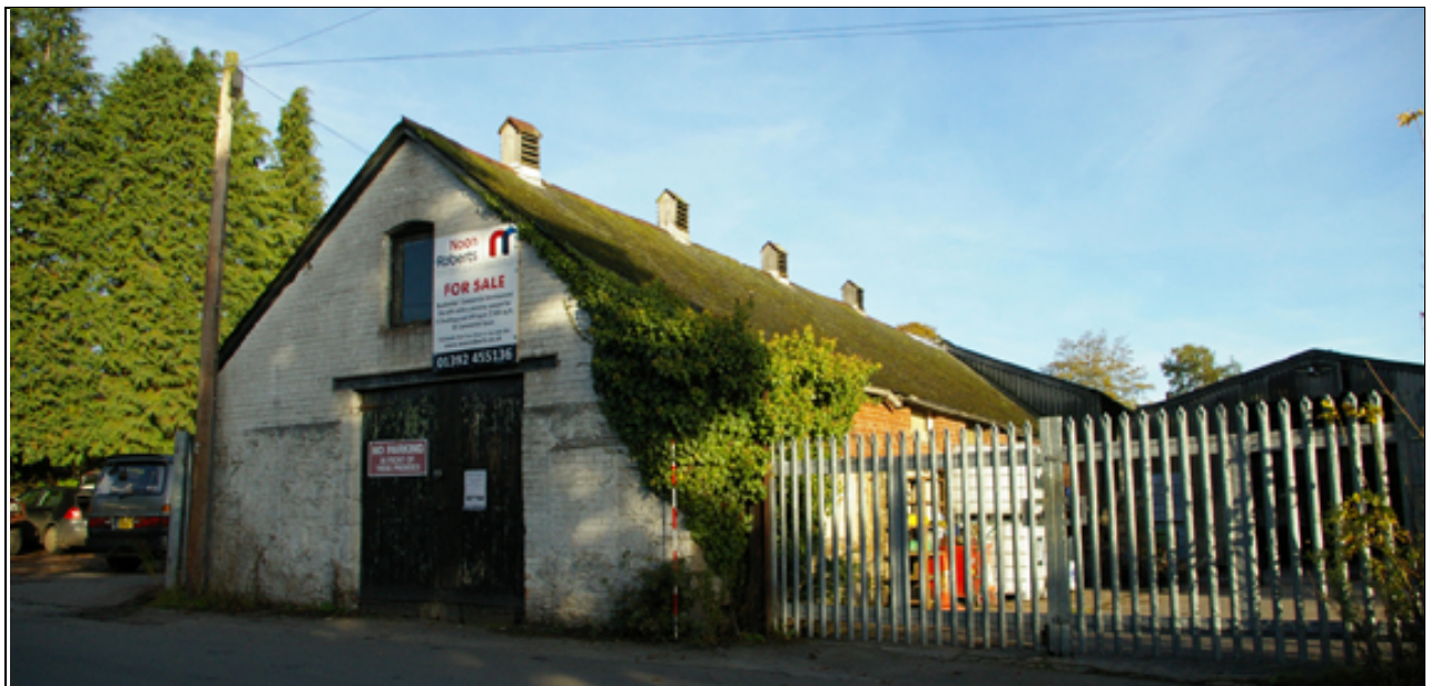
Figure 10: B1, viewed from the south-east.
