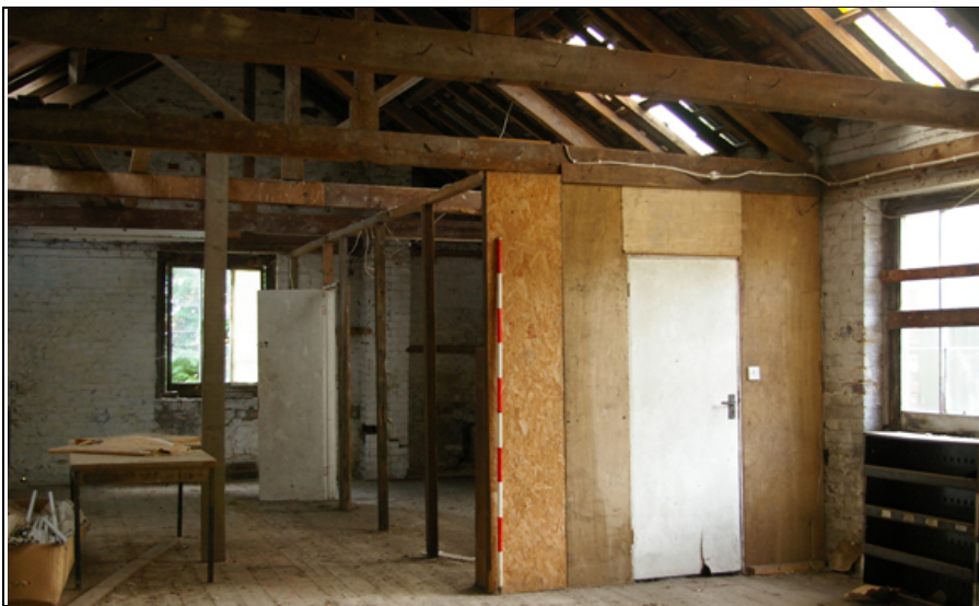
Figure 37: First floor interior of B2 (south), viewed from the north-west.
