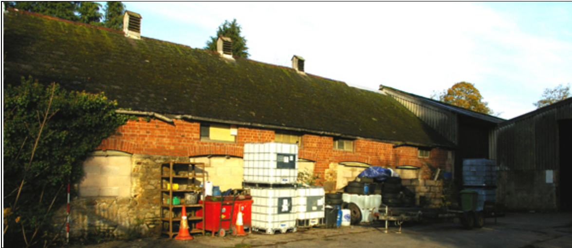
Figure 18: The east elevation of the southern portion of B1, viewed from the south-east.
