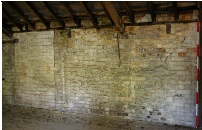
Figure 39: As Figure 35, viewed from the north.
