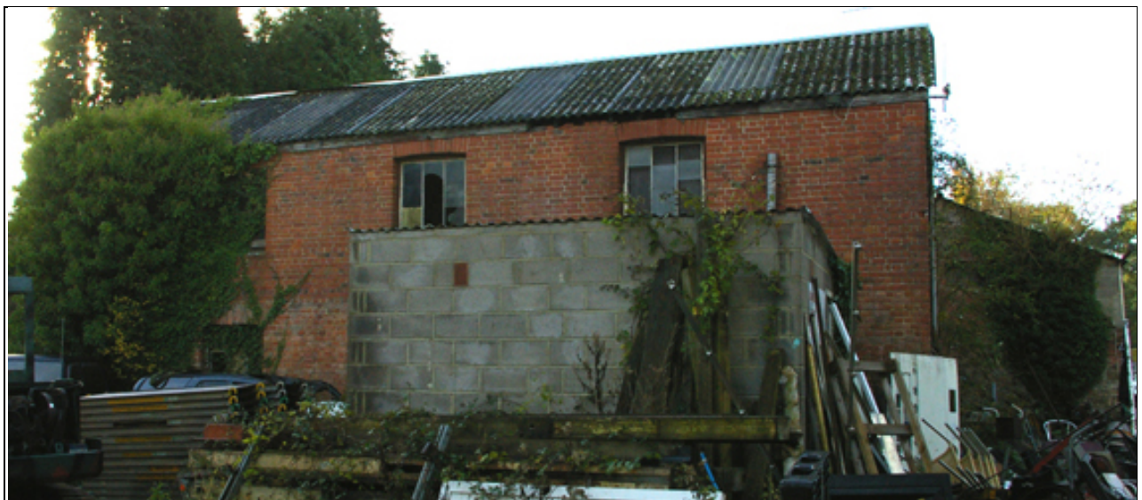
Figure 24: The north elevation of B2, viewed from the north.
