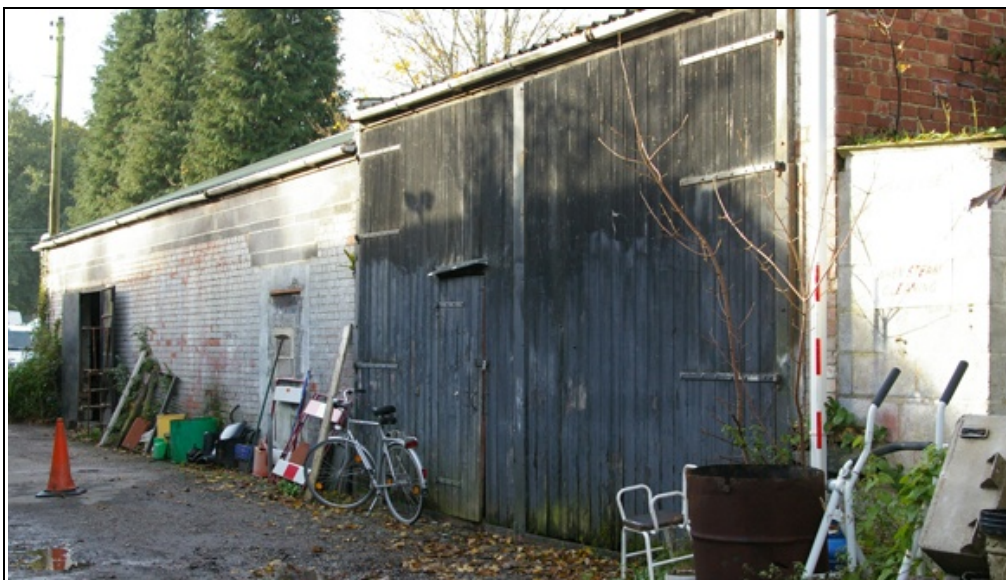
Figure 28: The east elevation of B3, viewed from the north-east.
