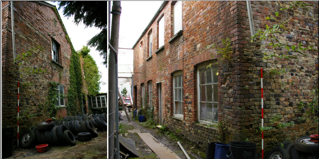
Figure 51: (left) The east elevation of (B2), viewed from the south-east.
