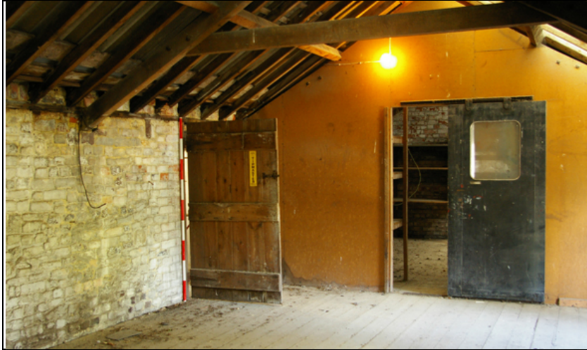
Figure 38: First floor western end of B2 (north), viewed from the north-east.
