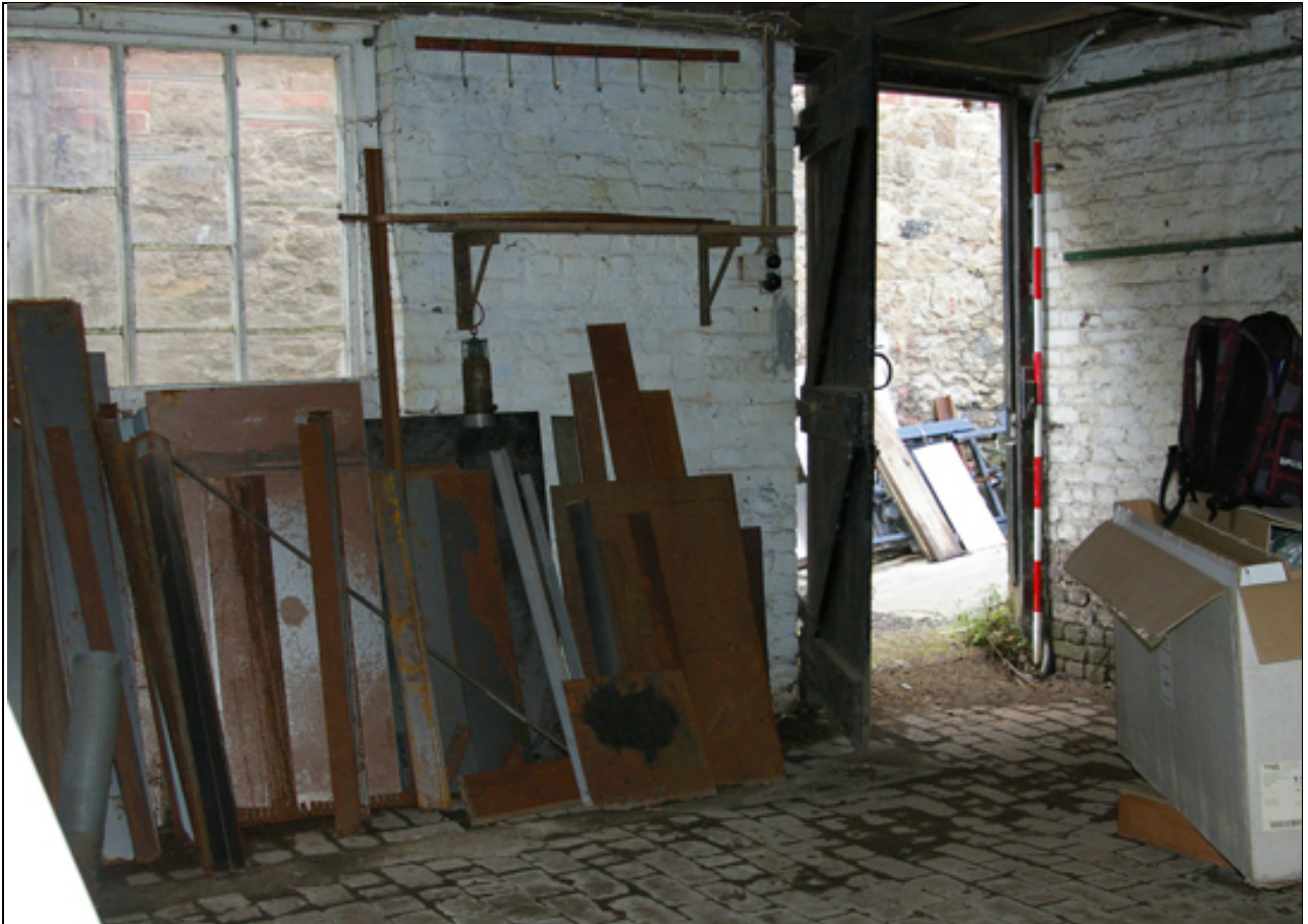
Figure 33: Interior ground floor north-west corner of B2, viewed from the south-east.
