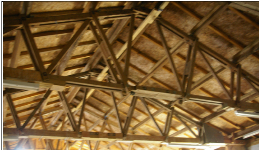
Figure 32: The roof structure over B3, viewed from the north-west.
