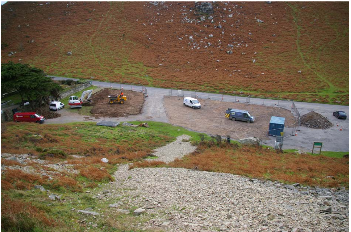
Figure 5: Site shot post-excavation, viewed from north (no scale).
