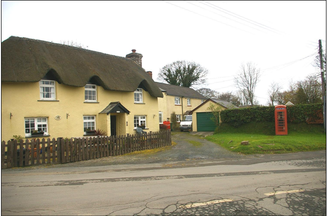
Holmdene and the K6 telephone kiosk in Ashwater, north-east of the main village green; from the south-west.
