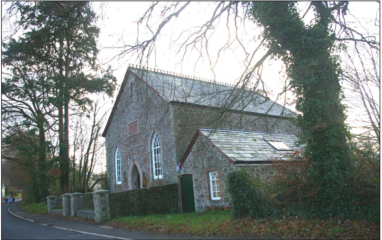
The Clawton Bridge Methodists Church in Clawton; from the south-east.
