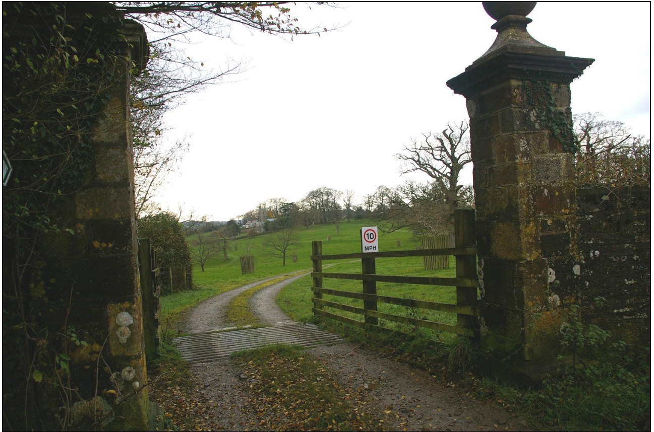
Tetcott Estate, showing the building complex set within the parkland landscape; from the north-east.
