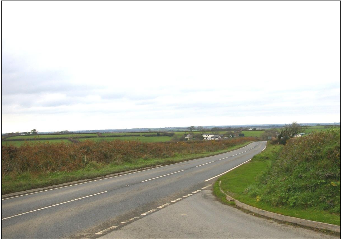
Cholditch Farmhouse, located to the west of the A388, on the northern side of a small valley; from the south-east.
