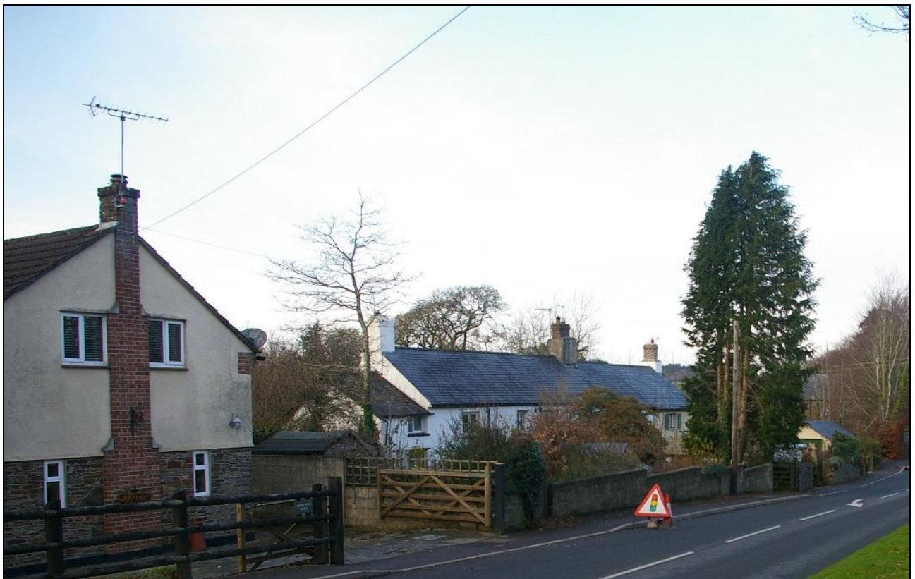
The row of attached Listed cottages in Clawton: Thorpe Cottage, Tudor Rose, Mazoe, Elm Cottage; from the south-east.
