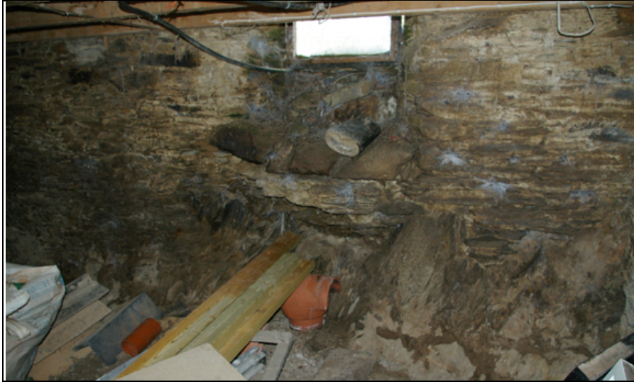
Figure 35: The interior ground-floor east wall of B1, with stone sill and window opening.
