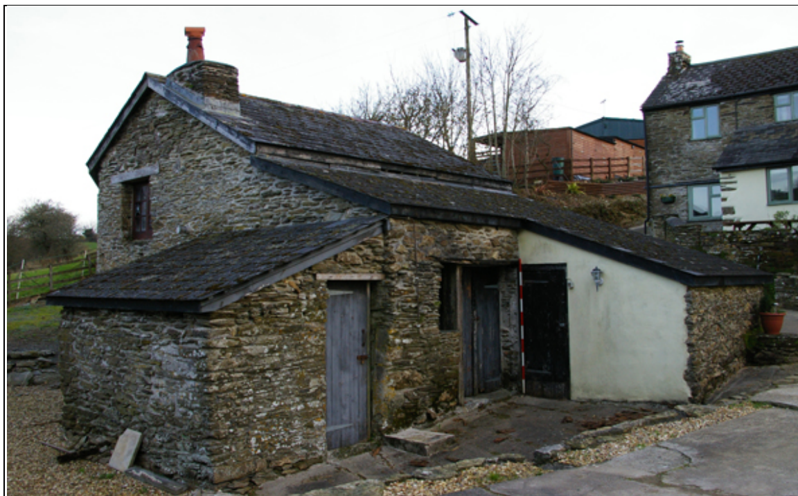
Figure 13: The mill, with lean-tos B1a, B1b & B1c built against the south elevation, from the south-west (scale 2m).
