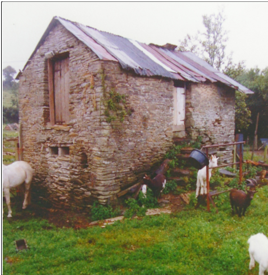
Figure 10: The north and east elevations of the granary, during the 1990s.
