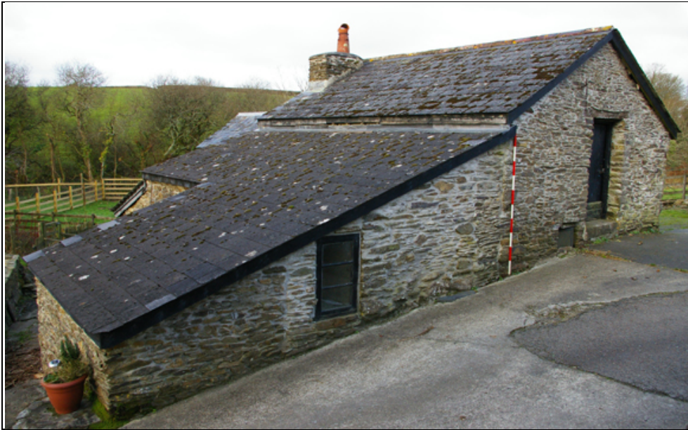
Figure 25: The east elevation of B1, from the south-east (scale 2m).
