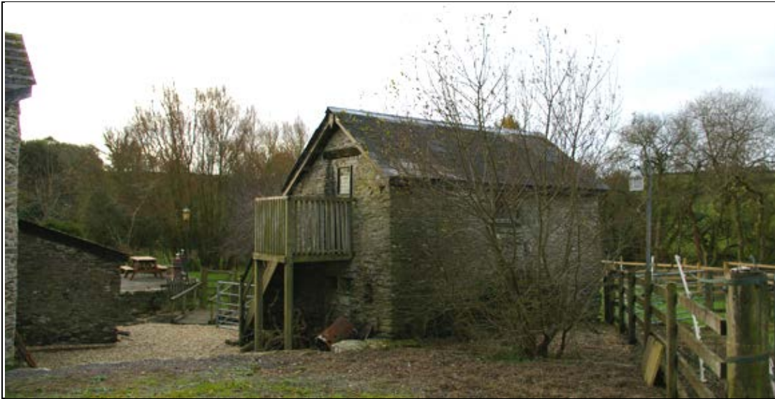
Figure 14: The Granary, Building 2 (B2), from the north-east
