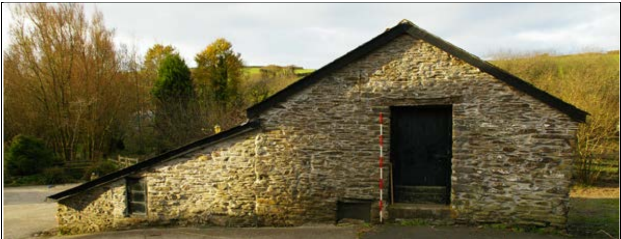
Figure 24: The east elevation of B1, from the east (scale 2m).
