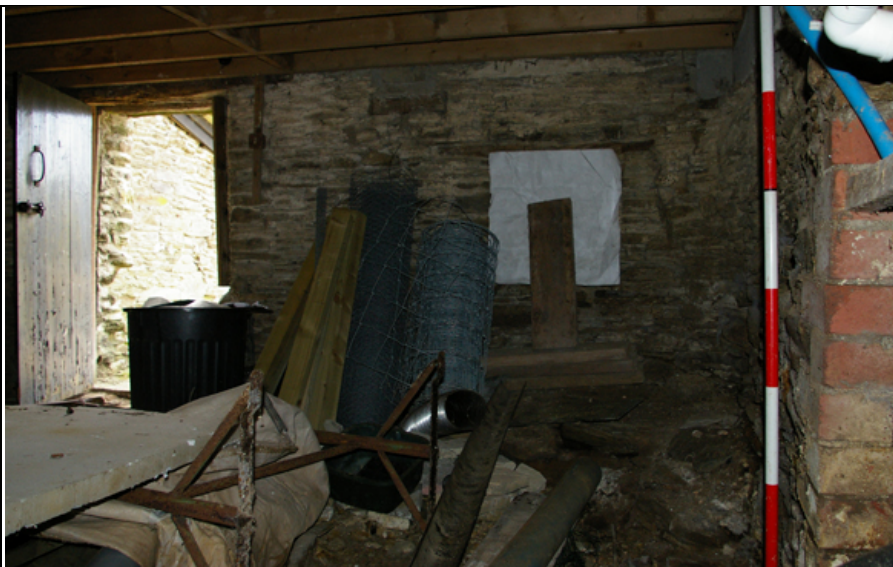
Figure 37: Ground-floor interior north-west corner of B1, from the east (scale 2m).
