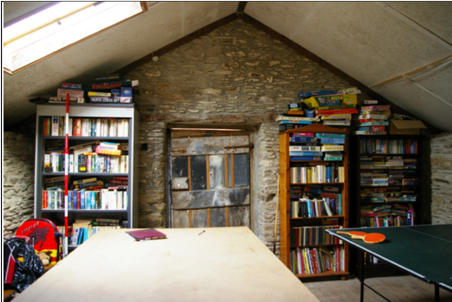
Figure 42: The interior first-floor east wall of B1, from the west (scale 2m).
