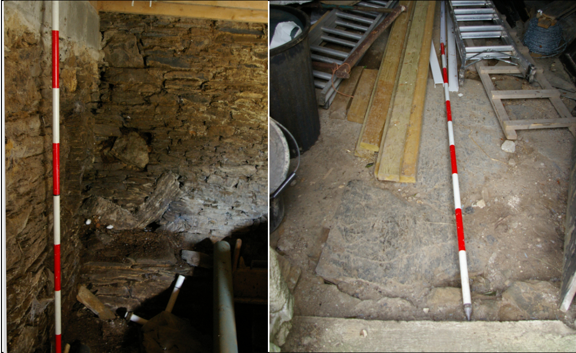
Figure 38: Detail of the interior north-east corner of B1, built on the bedrock, from the west (scale 2m).
