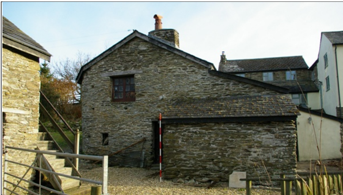
Figure 2: The west elevation of the mill (B1) and lean-to B1c, from the south-west (scale 2m).
