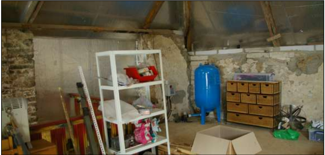
Figure 24: The cob built north-west corner of the barn, viewed from the south-east.
