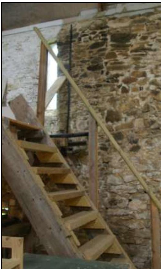
Figure 17: The disturbance in the south wall of the barn in the former position of the return of the east wall, viewed from the north.
