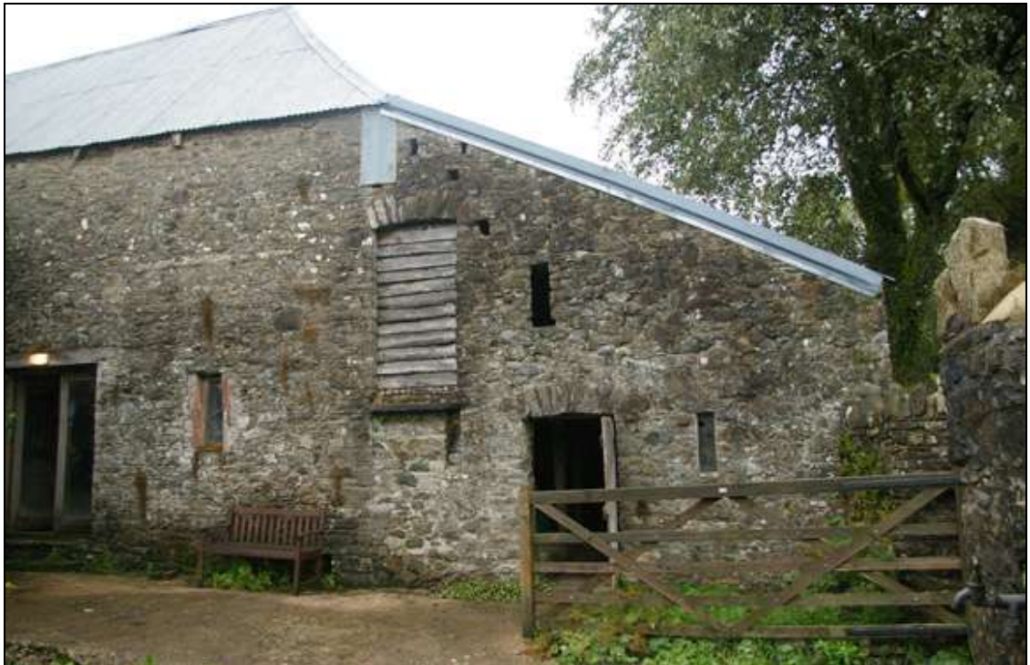
Figure 6: The south elevation of the eastern lean-to and the east end of the barn, with the entrance gate into the yard to the right; viewed from the south-east.
