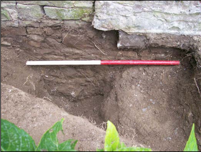
Figure 1: Footings immediately beneath repair, viewed from the west (1m scale).
