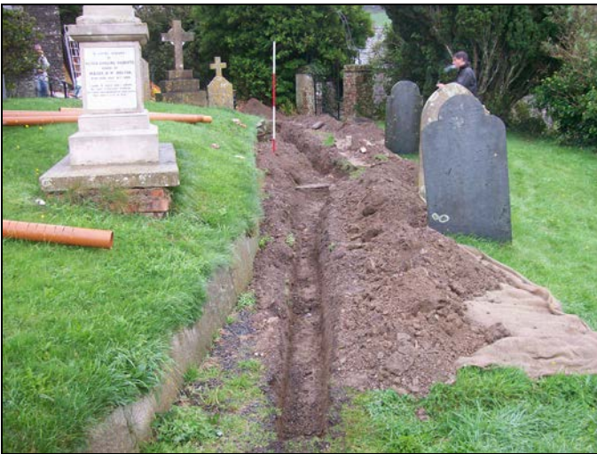
Figure 3: South part of pipe trench, viewed from the west (2m scale).
