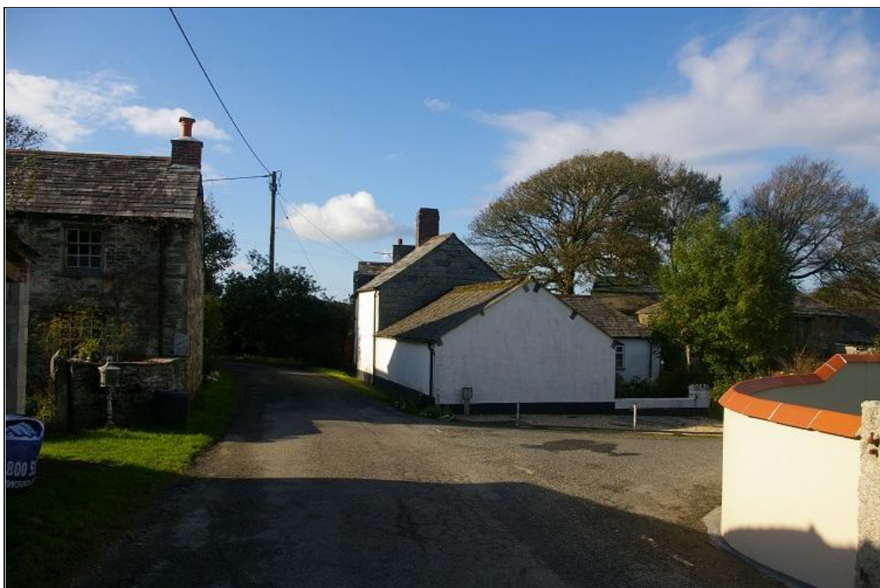
Trelash House and stone outbuilding behind adjacent cottage, both within Trelash settlement; from the east.
