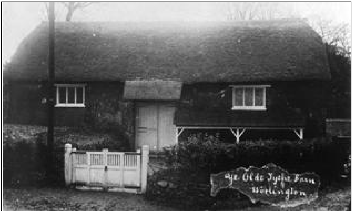
Figure 4: Photograph of the building dating from the early part of the 20 th century, showing the mullioned windows, ‘pent house’ and verandah.
