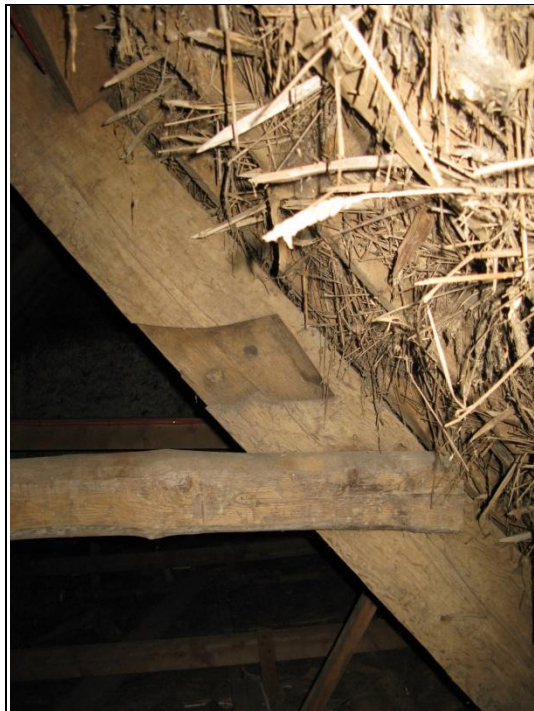
Figure 8: The former collar joint above a later spiked timber on an early roof truss.
