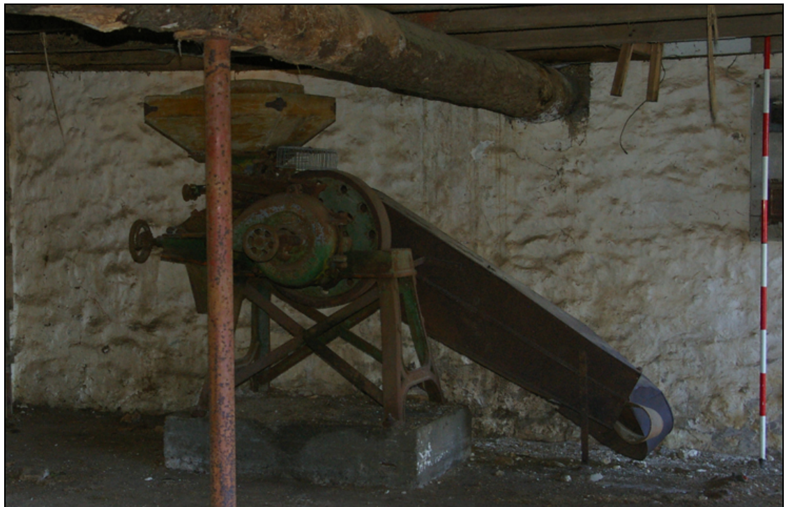
Figure 10: The ground floor south-west corner of B1, with the Bentall Grinding Mill, viewed from the north-east.
