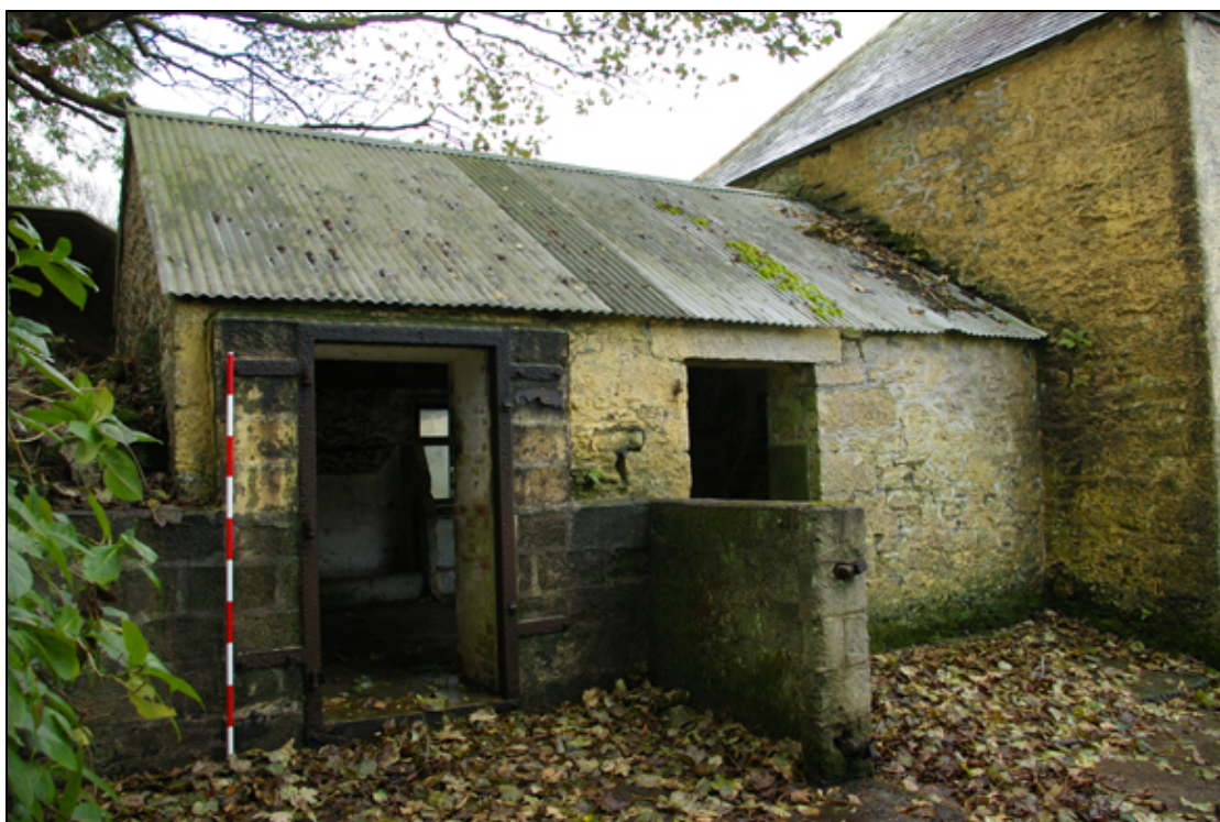
Figure 14: The north elevation of B1a, viewed from the north
