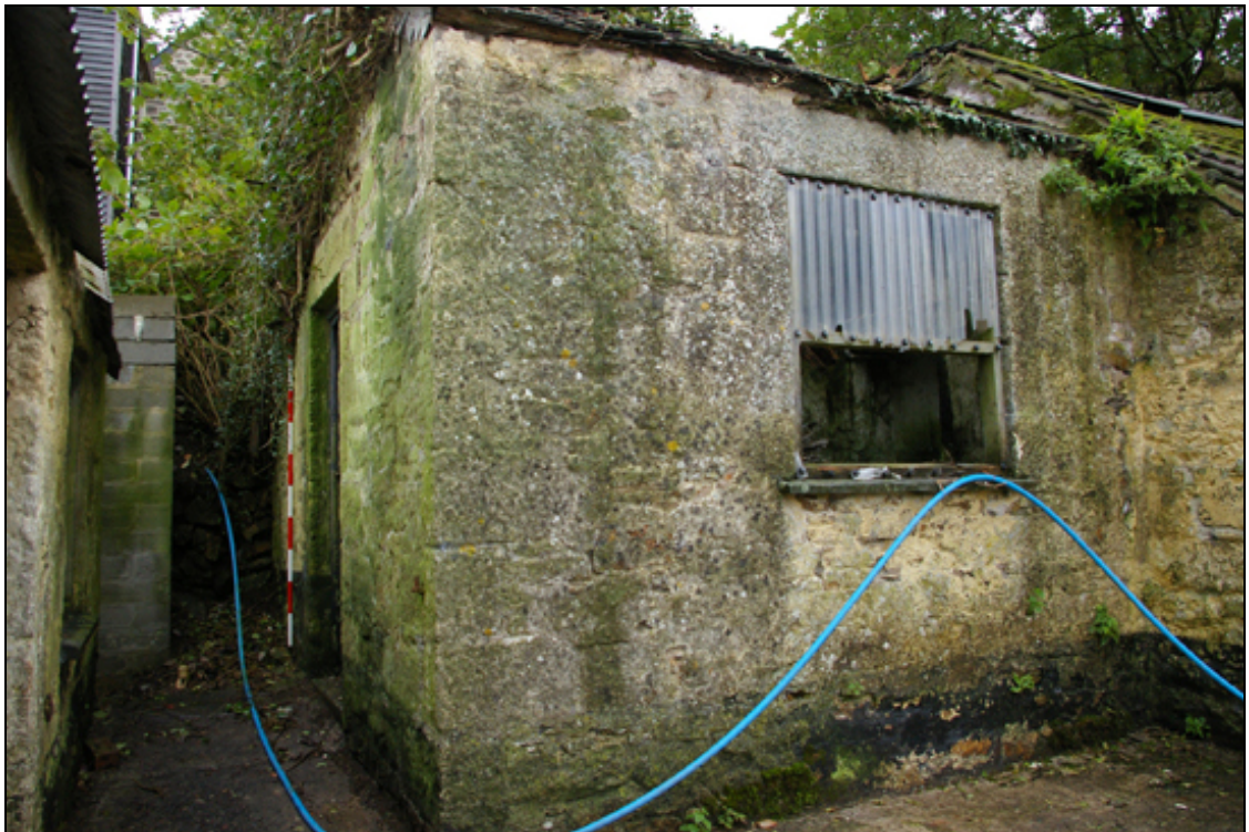
Figure 20: B2a, viewed from the west.
