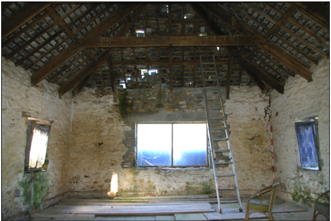
Figure 13: The interior west end of the first floor of the chall barn (B1), with central inserted window, viewed from the south-east.
