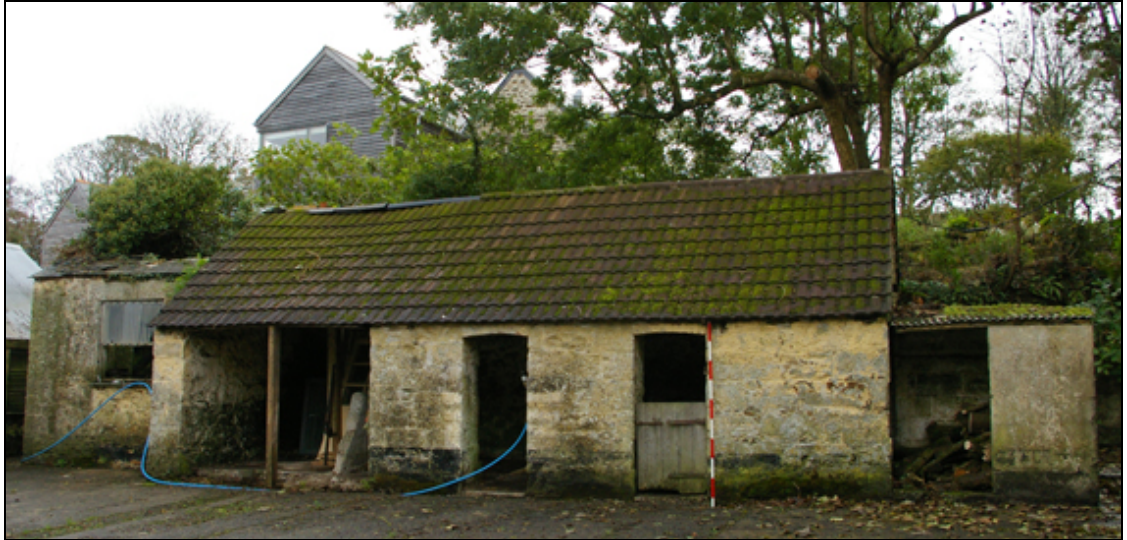
Figure 18: The west elevation of B2, viewed from the west.
