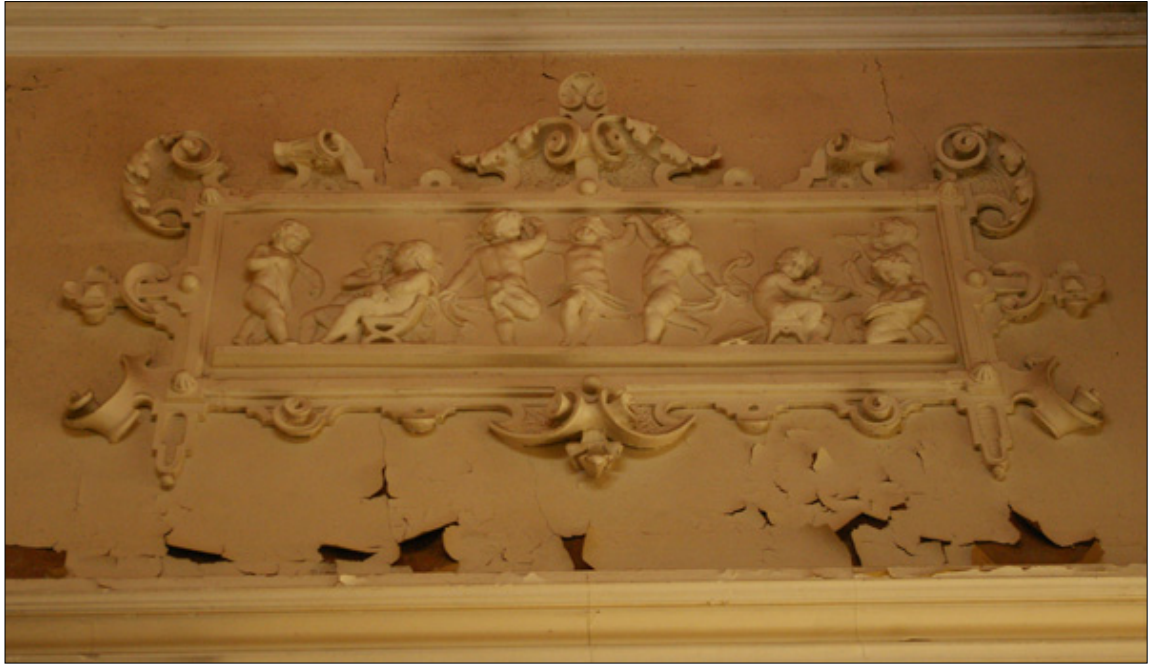
Figure 13: Plaster decoration within the stairwell.
