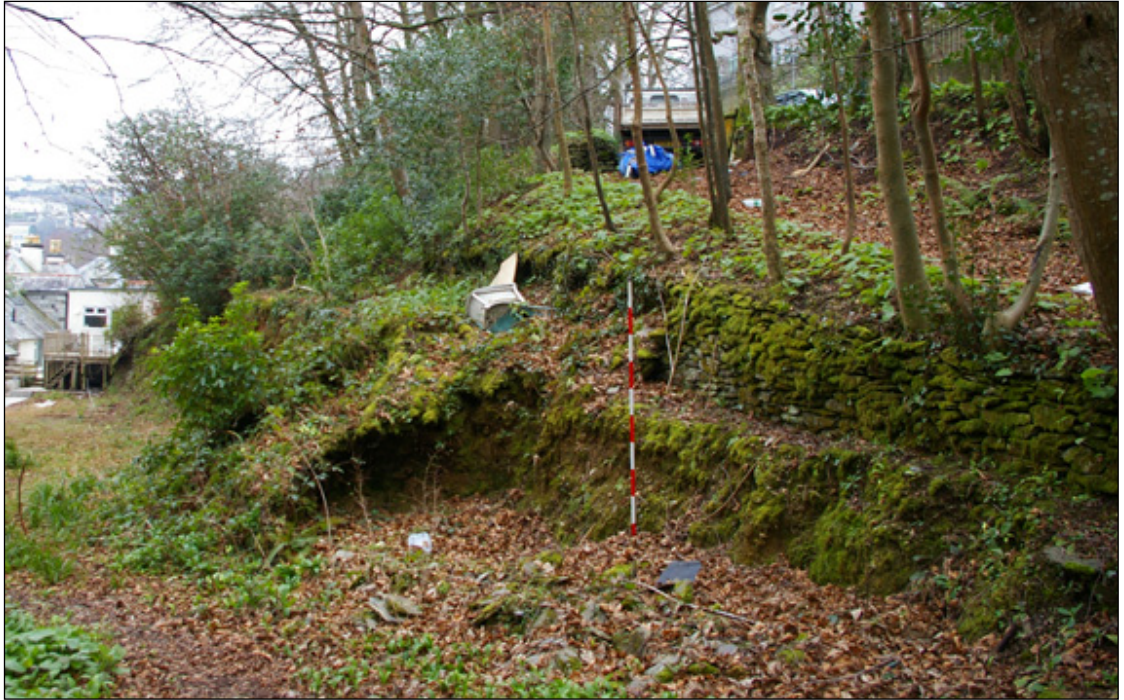
Figure 22: The modern access track to the east of the former garage (van positioned in entrance), with a partially truncated pathway beneath, and the wider path further below, viewed from the west (2m scale).
