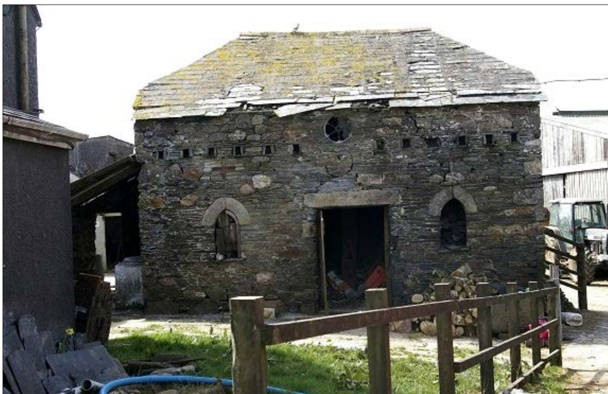
Listed outbuilding on Trela Farm, showing how it is blocked by the modern buildings ; from the north.
