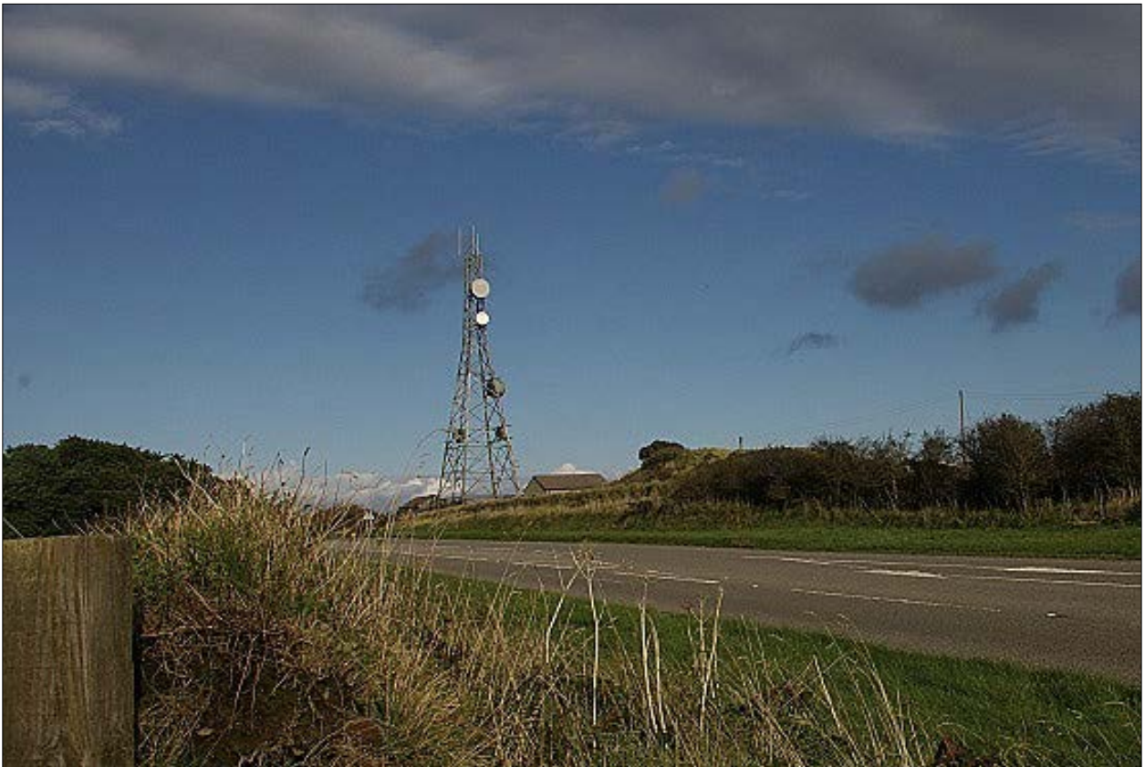
Barrow cemetery near Trehane Pool, Titich barrow, with adjacent mast and sub station; from the south-west.
