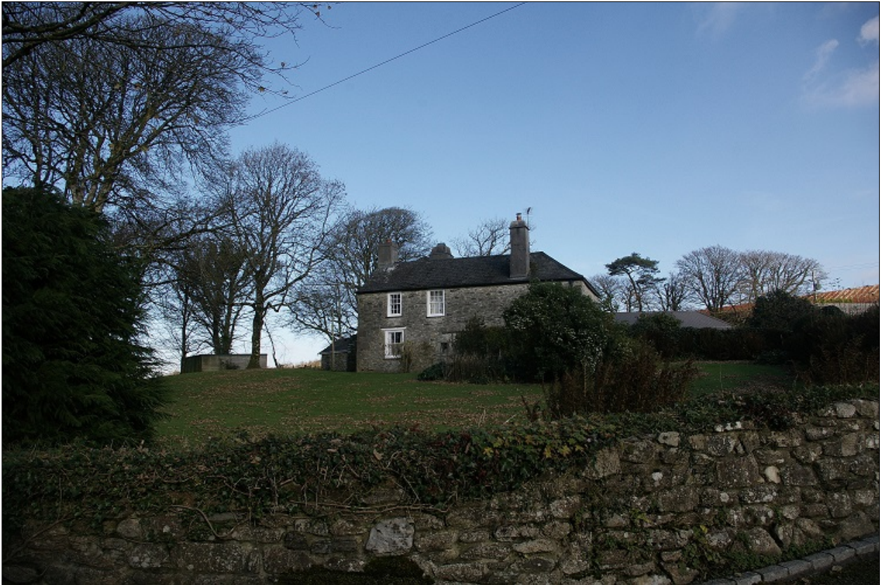
Trethin Farm, showing how the house sits north of its barns and buildings and is surrounded by trees on the hedgebank which forms the farmstead enclosure; from the west.
