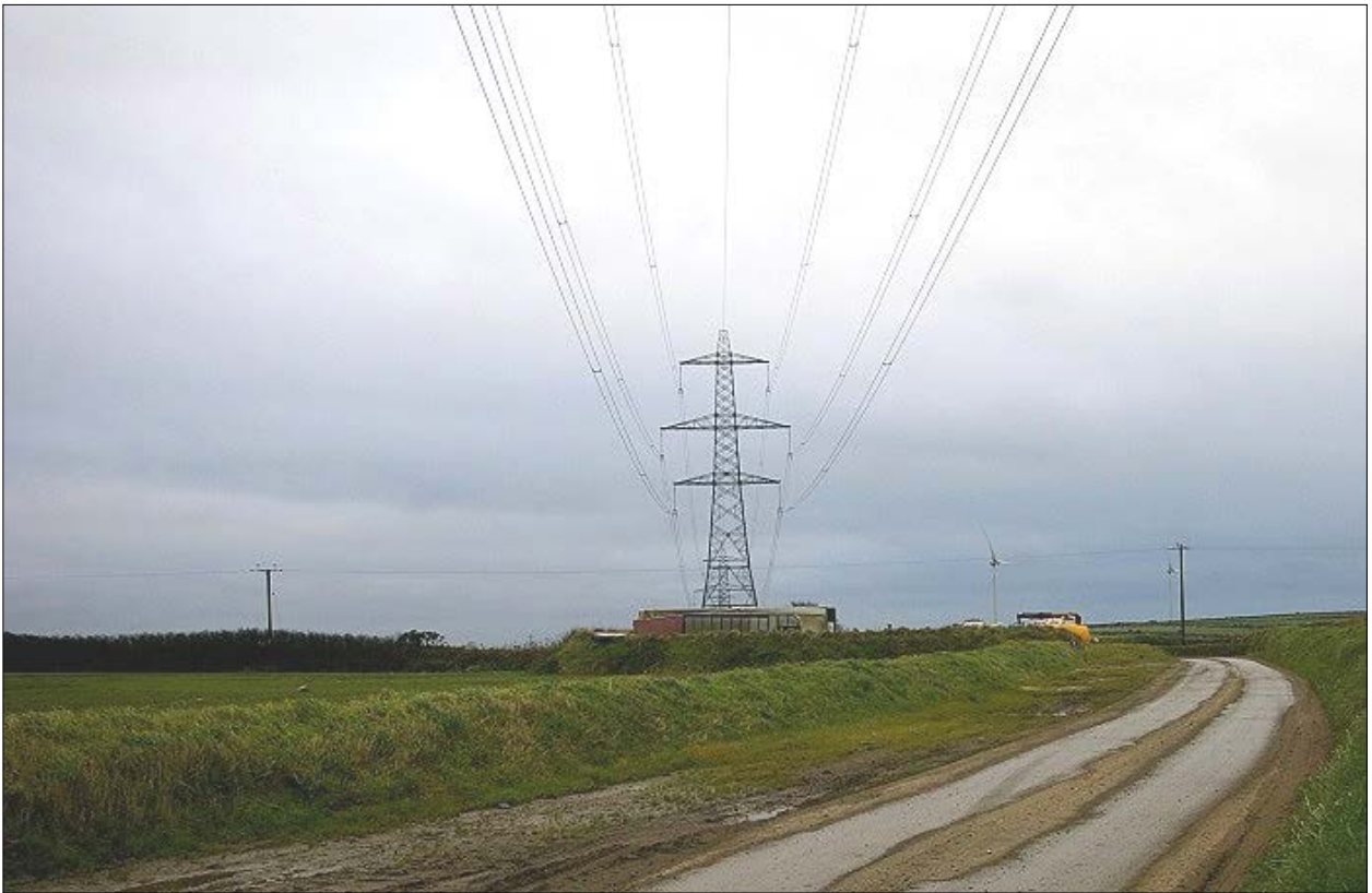
The track entrance to the site, lorry park area and line of pylons; from the north-east.
