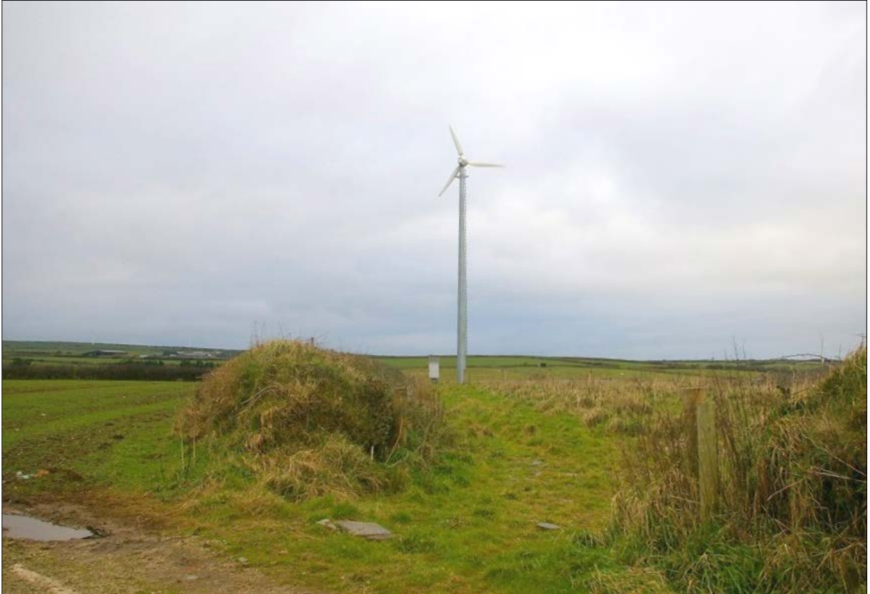
As above, detailed view of the extant turbine; from the south.
