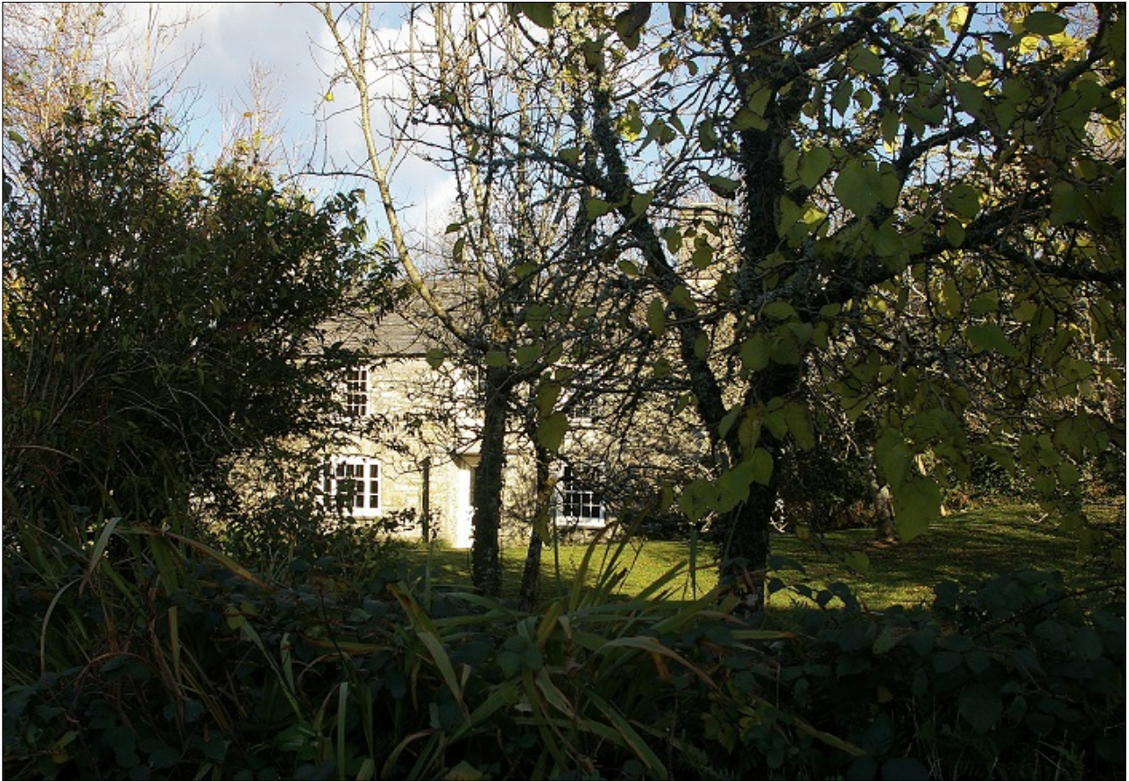
Glen Mead, Listed building to the west of Helstone, set in its own gardens, shielded by apple trees and mature shrubs; from the south-east.
