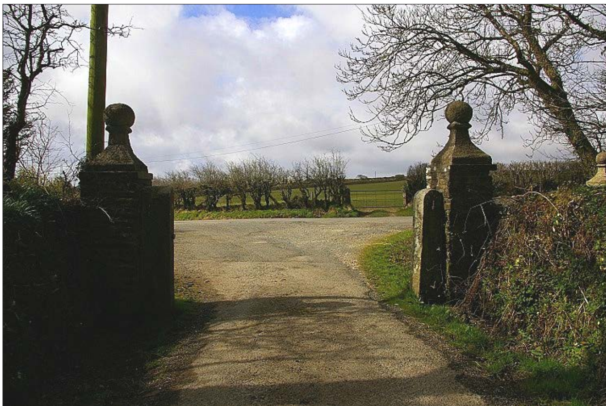
The gate piers at Halwill Barton; from the north-east.
