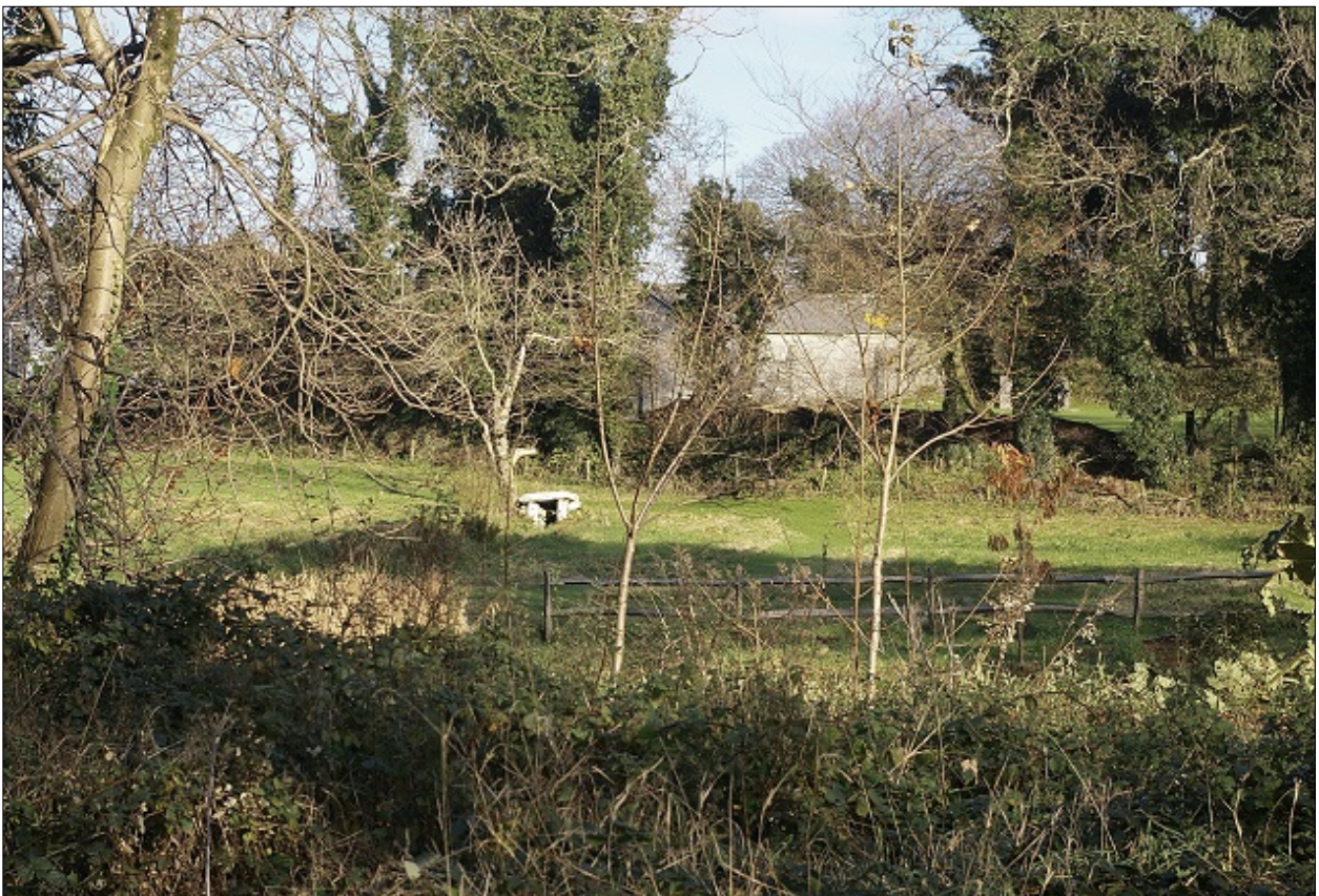
The well house at Trethin Farm, set into a sloping bank, with little to no landscape presence and easily locally blocked by the hedgebanks and trees of the fields; from the south-west.
