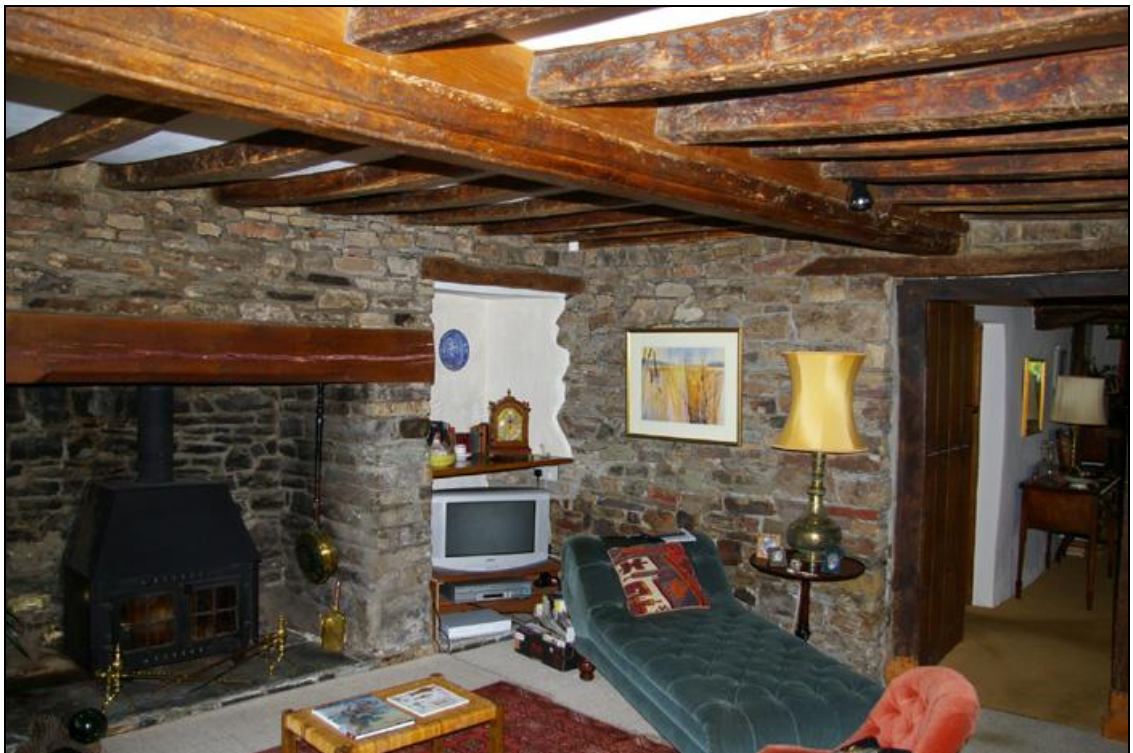
Figure 14: The drawing room (3) showing the fireplace, the possible former door opening and the 17 th century doorframe; viewed from the south-west .
