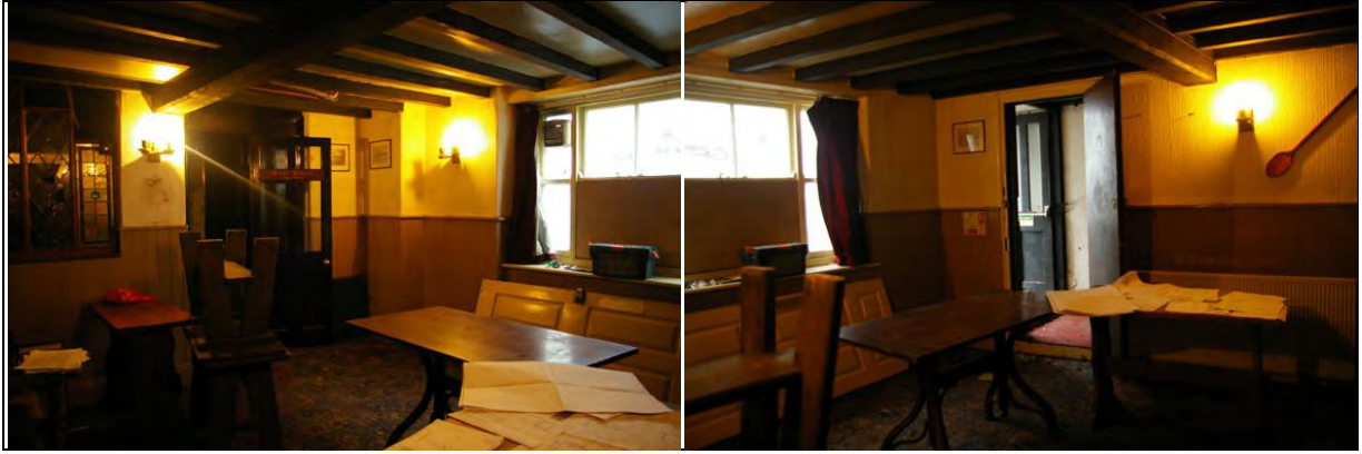
Figure 34: Left: The N-W corner of G2, from S-E. Figure 35: Right: The SE corner of G2, from S-W.
