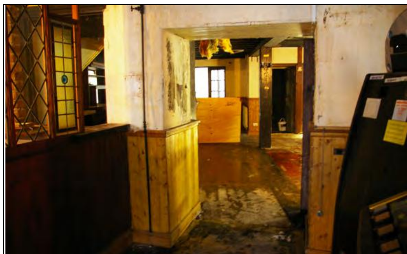
Figure 41: Opposed door opening in S wall, from N.
