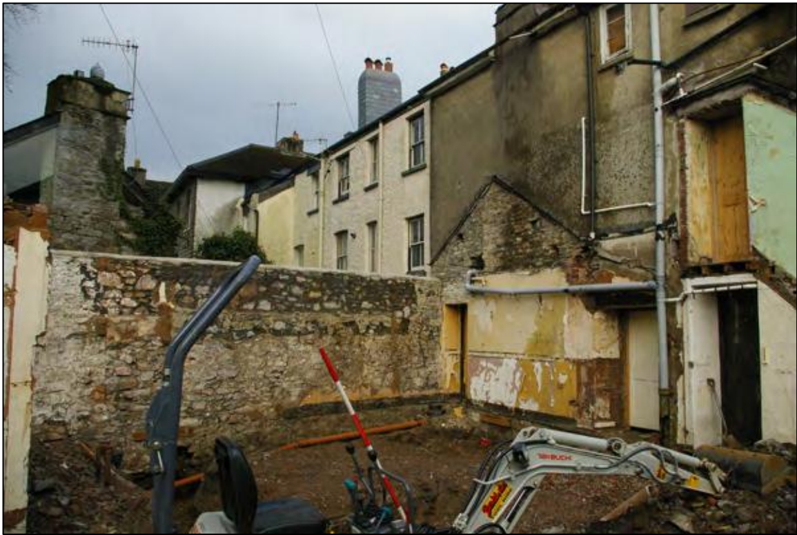
Figure 19: Site shot post excavation, viewed from the south-east.
