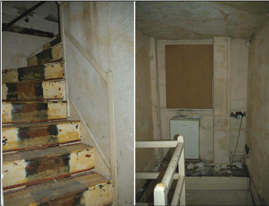
Figure 56: Left: stair to second floor, from S.
