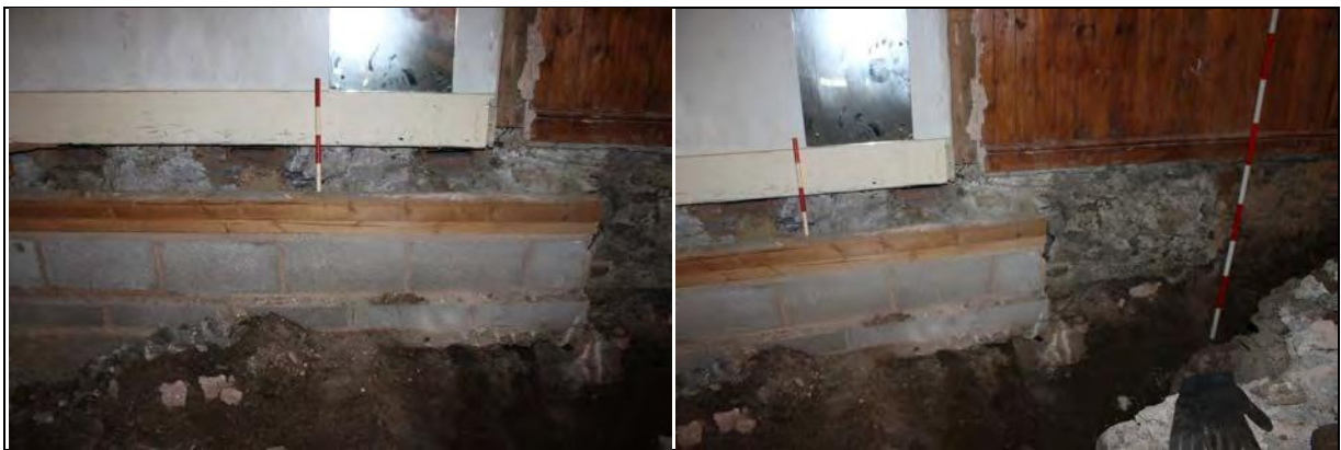
Figure 81: Left: W wall within demolished toilet block (G5), from E.
