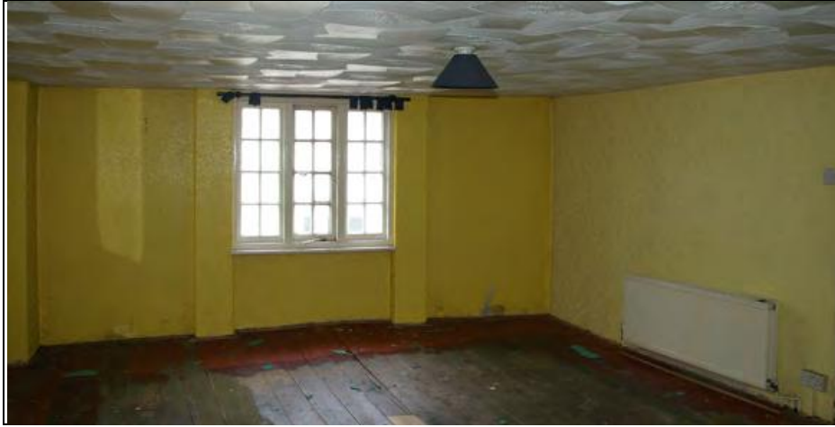
Figure 62: N-E corner of S5, from S-W.
