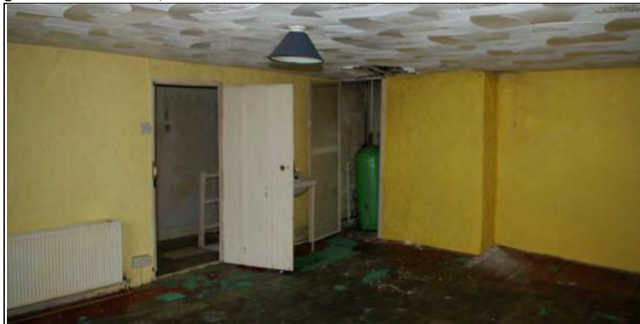
Figure 61: S-E corner of bedroom S5, from N-W.
