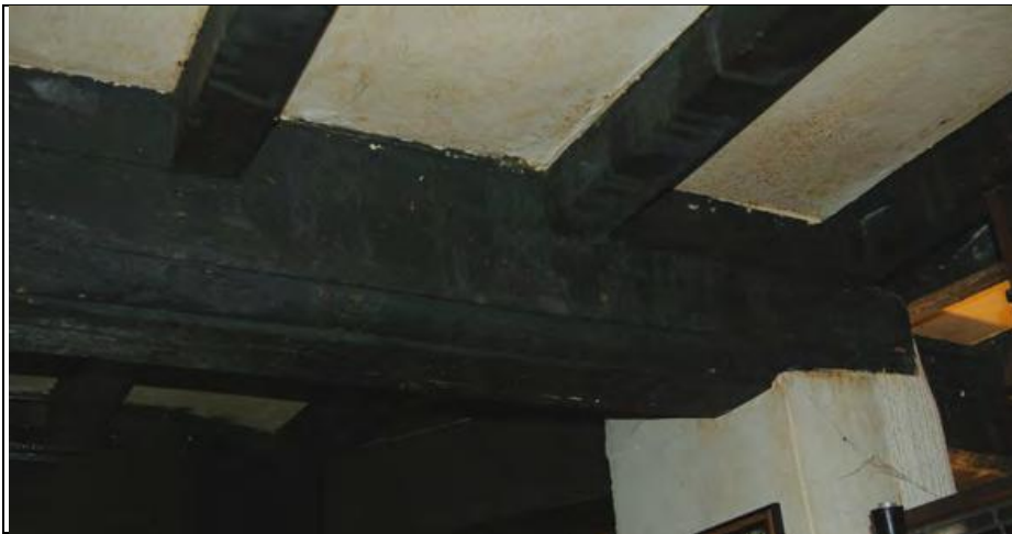
Figure 8: The truncated 17 th century moulded beam in G3, from the south.
