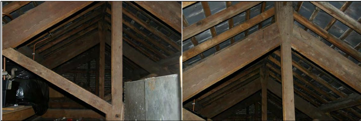
Figure 67: Left: roof structure over rooms S4 & S5, from the E.
