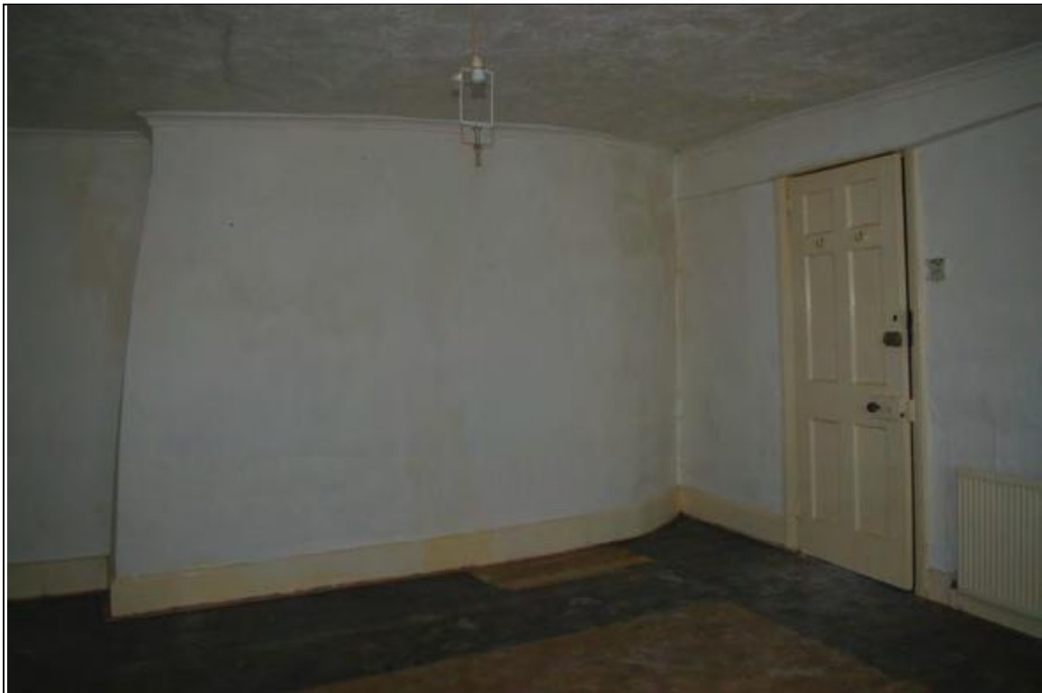
Figure 13: The chimney projection within the south-west corner of room F2, from the north-east.
