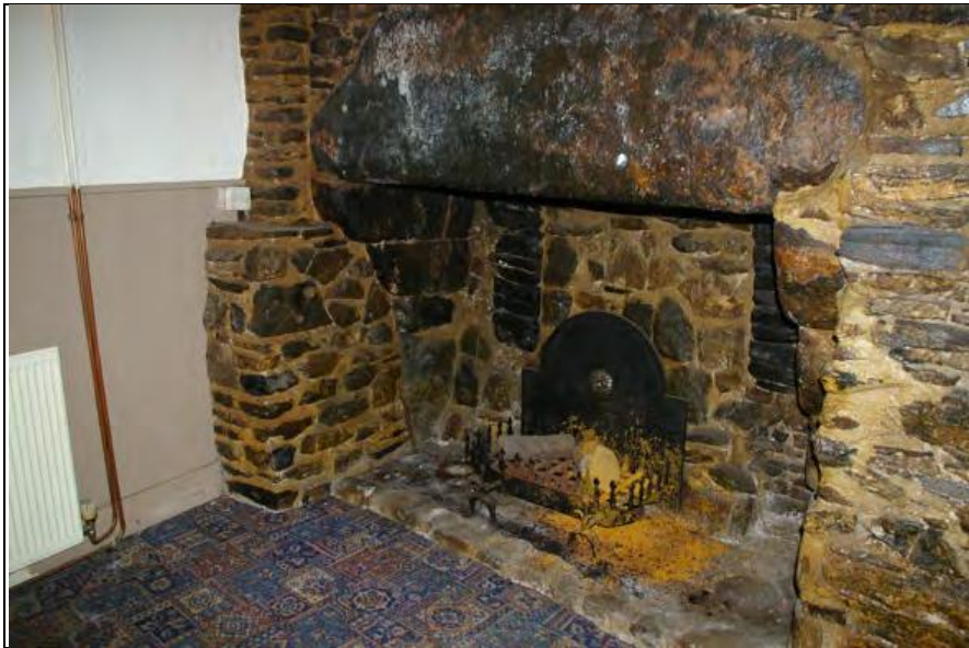
Figure 36: Fireplace in G2, from N-W.
