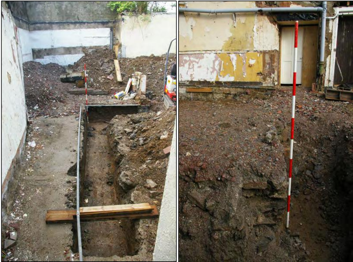
Figure 20: Eastern footing trench, viewed from the north (2m scale).
