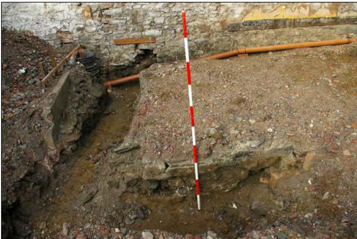
Figure 22: Middle and south end of footing trench showing wall {108}, viewed from east (2m scale).
