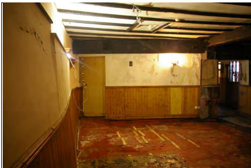
Figure 44: N and W walls of G4, from S.
