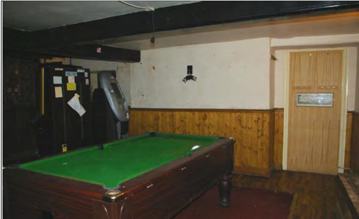
Figure 11: The interior south wall of the former games room (G3), with fireplace projection to the centre and forced opening to the right, with former cross passage to the left; from the north-east.
