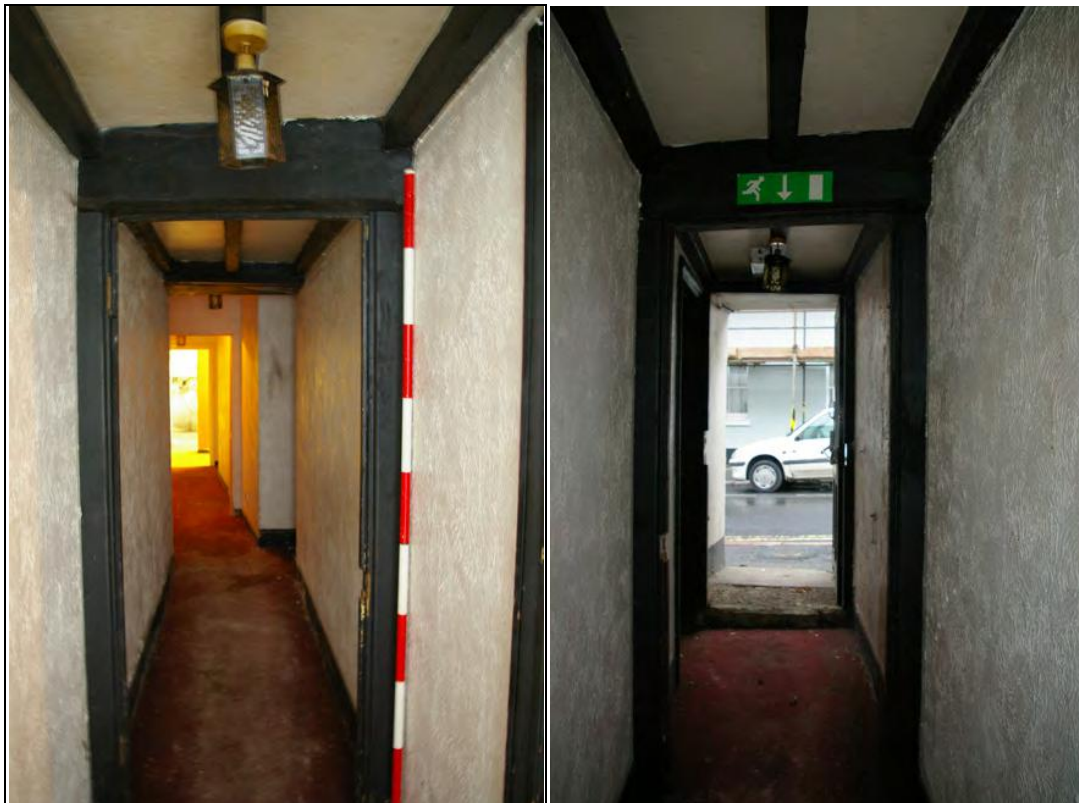
Figure 32: The E passageway G1, with chamfered joist, from the N.
