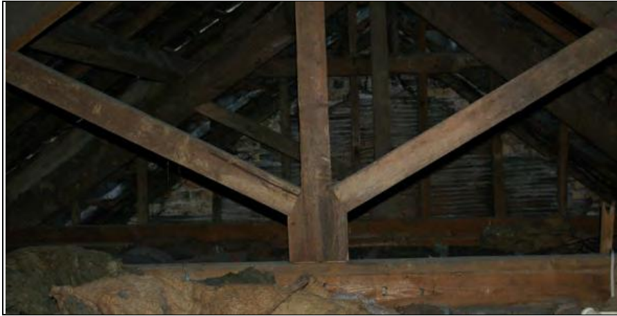
Figure 66: Roof structure over S3, from the W.
