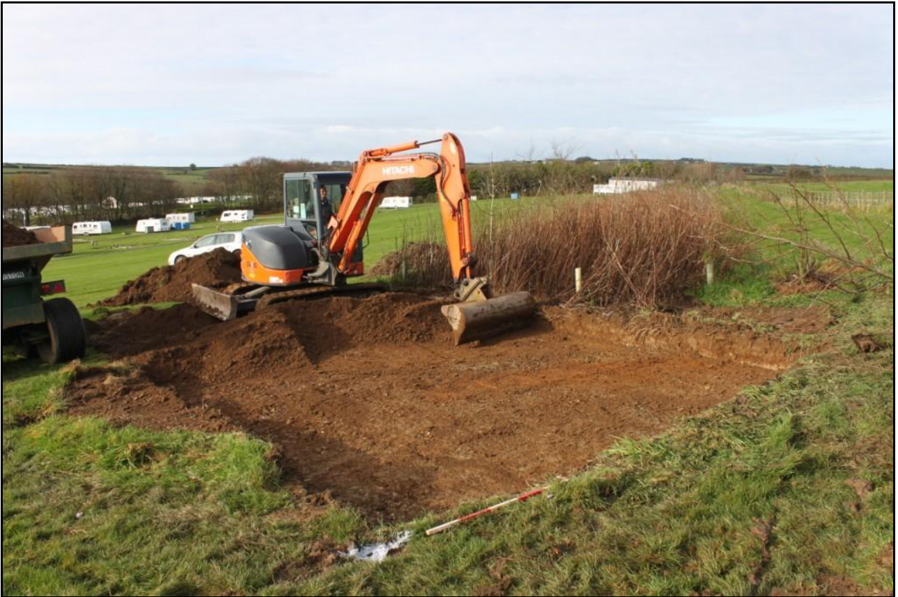
23. PLOT H, DURING EXCAVATION; VIEWED FROM THE NORTH-EAST (1M SCALE).
