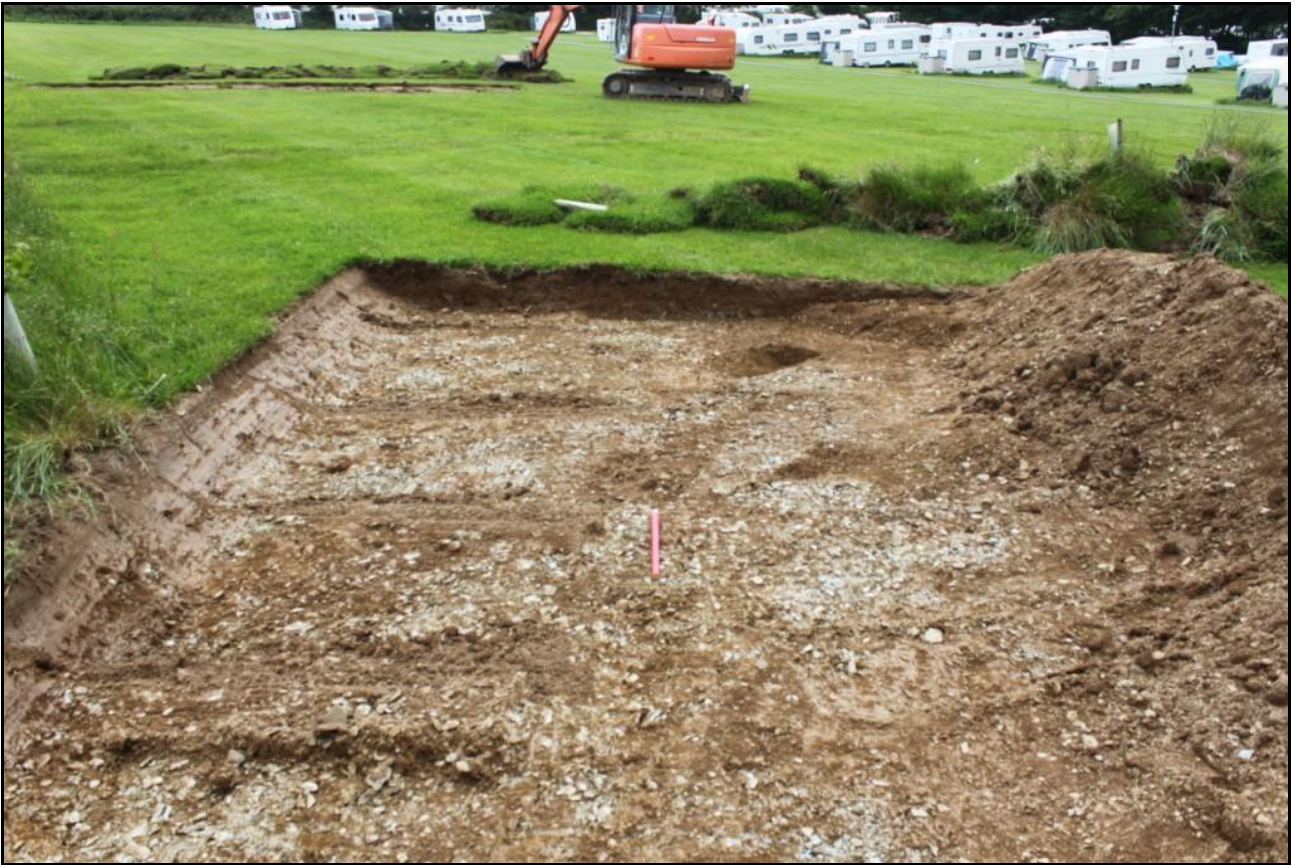
7. POST-EX SHOT OF PLOT C; VIEWED FROM THE NORTH-WEST (0.5M SCALE).
