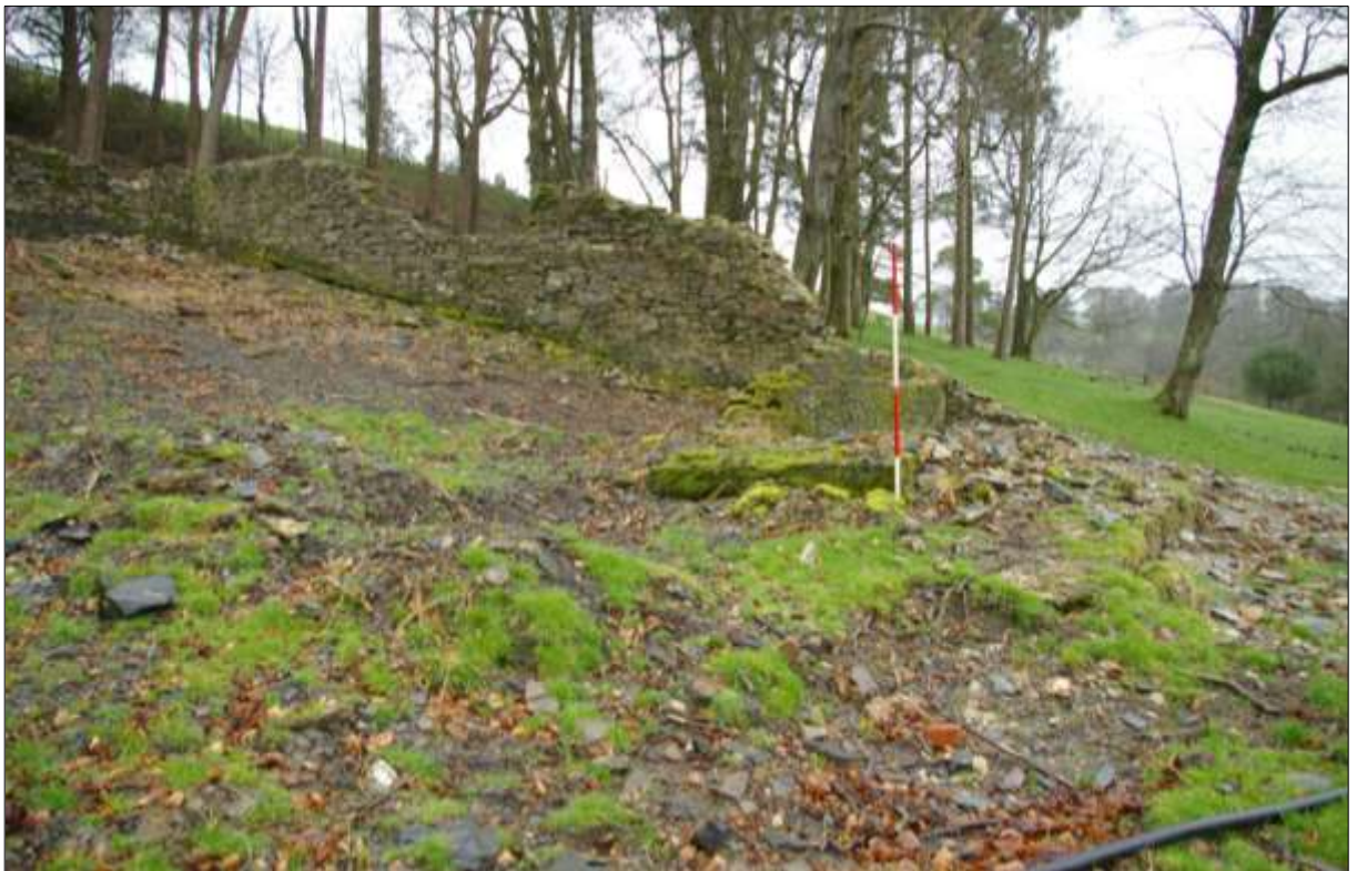
The east and south elevation and the interior room, from the west.
