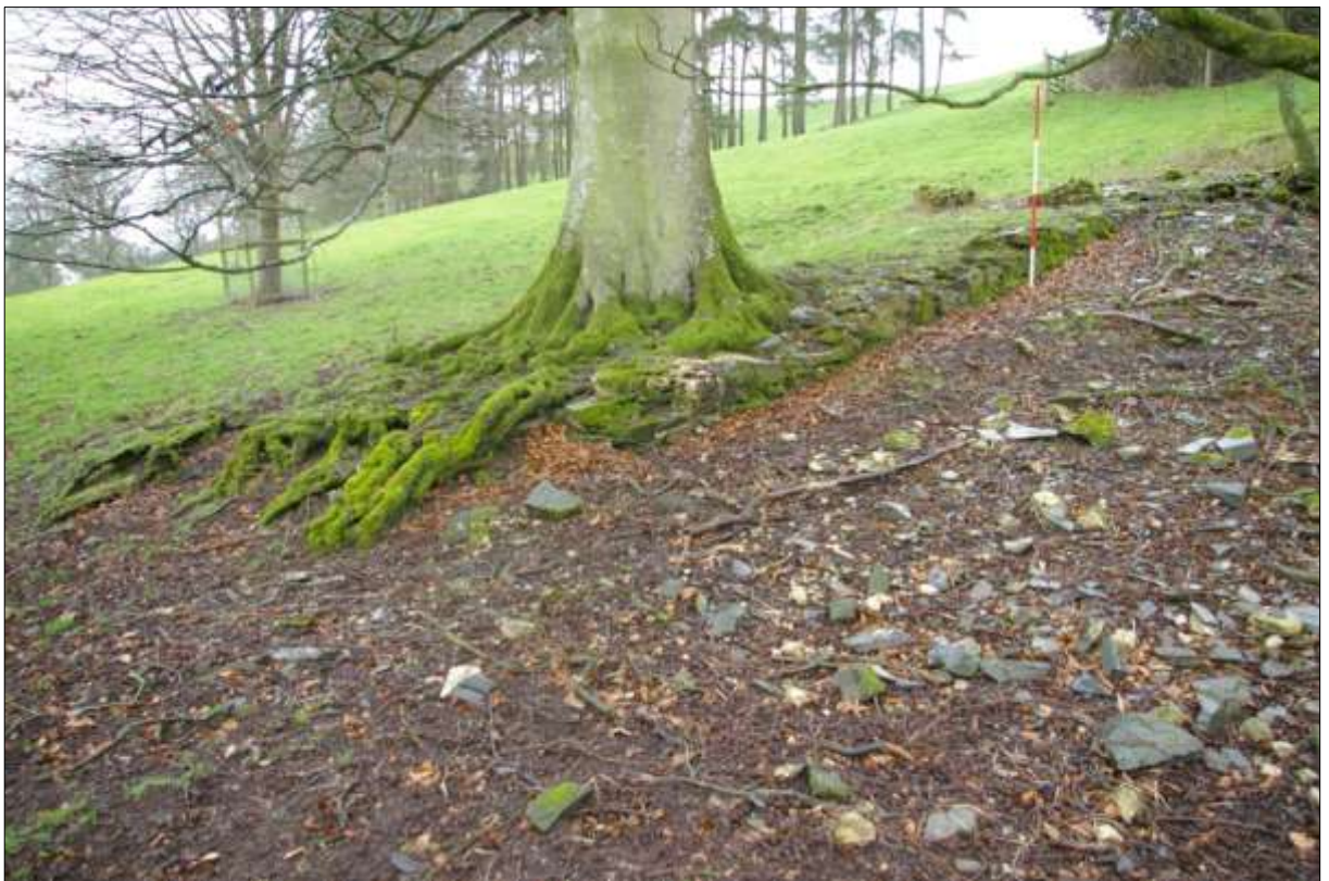
The west elevation including the large beech tree, from the south-east.
