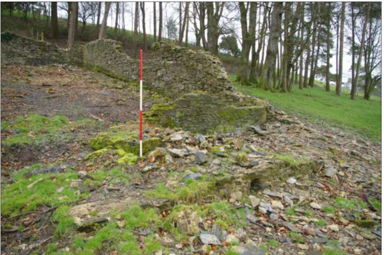
The east elevation and the small interior room, from the south-east.
