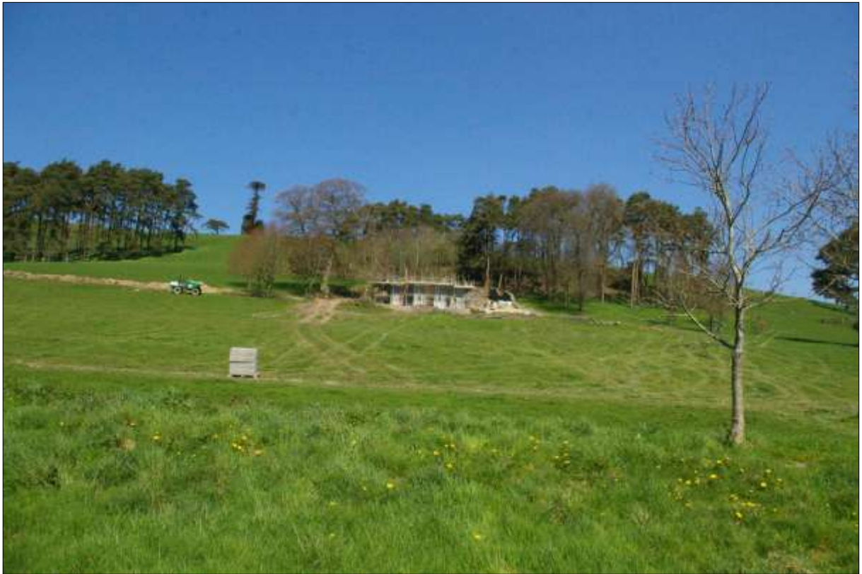
The site during construction, viewed from the south-west.
