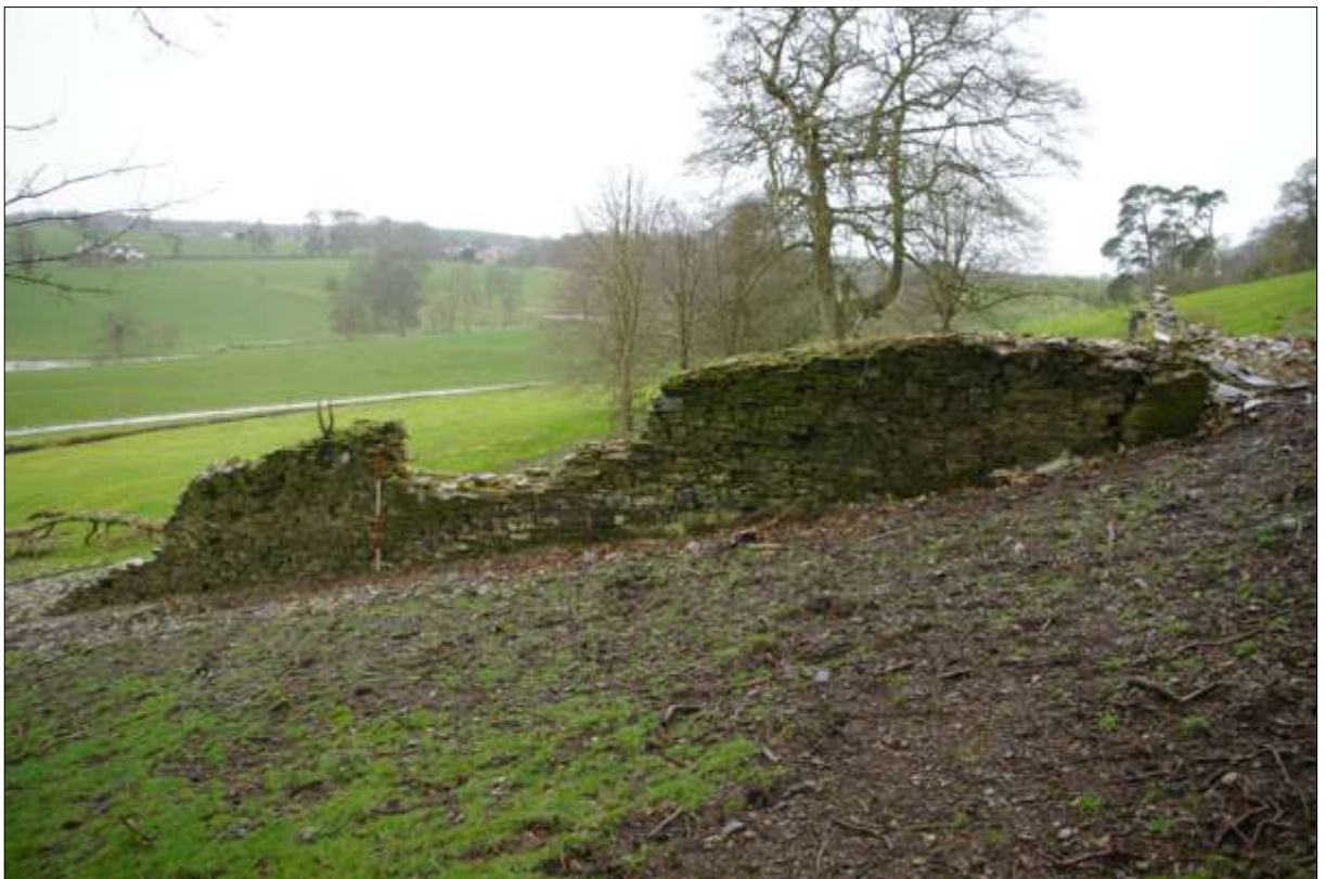
The east elevation, from the north-east.
