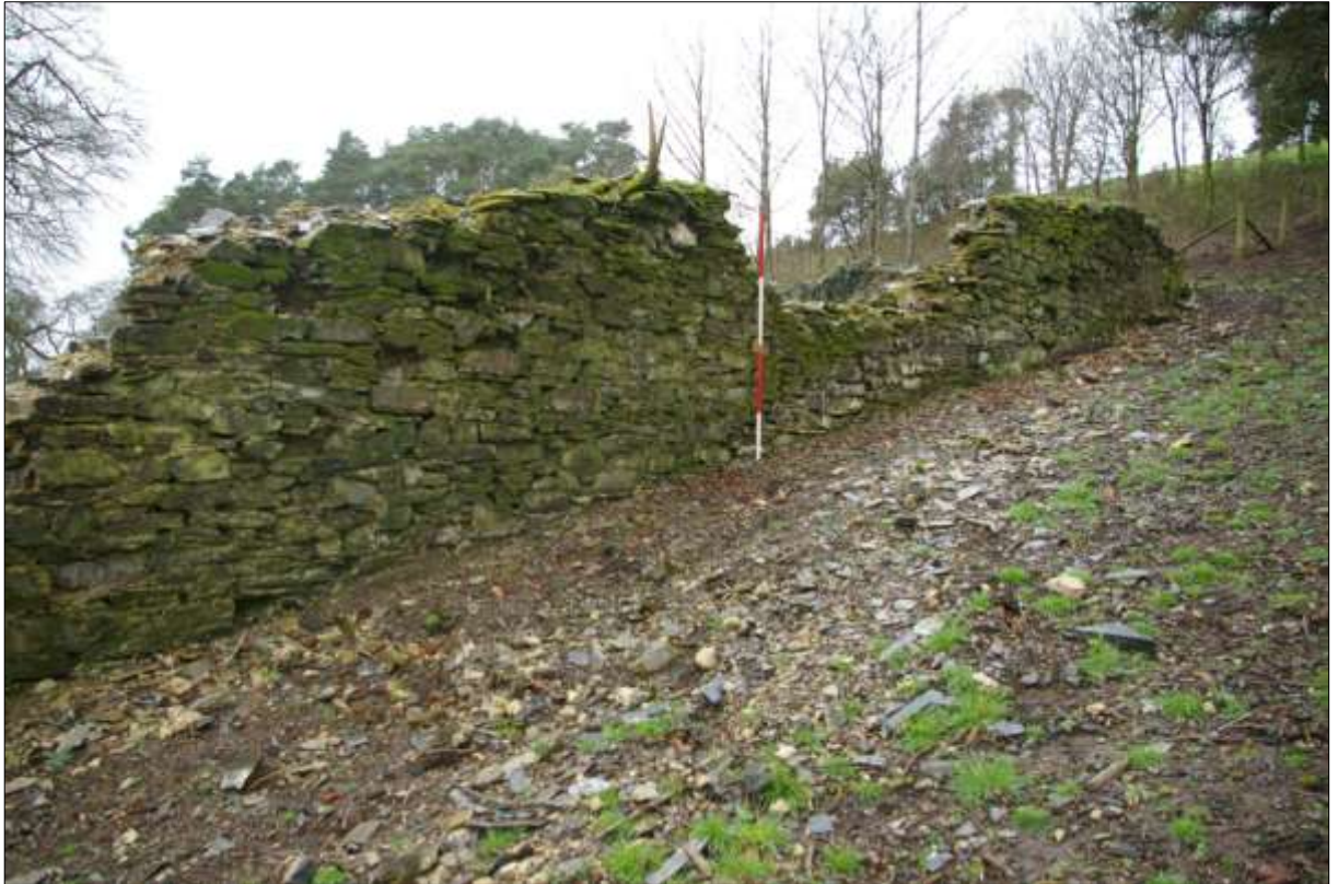
The north end of the east elevation, from the south-east.
