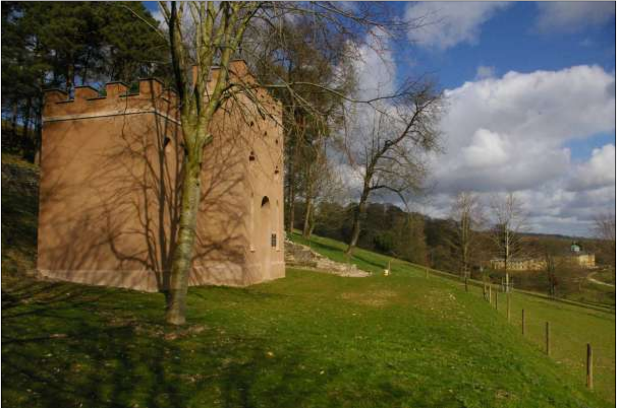
As above, looking east.
