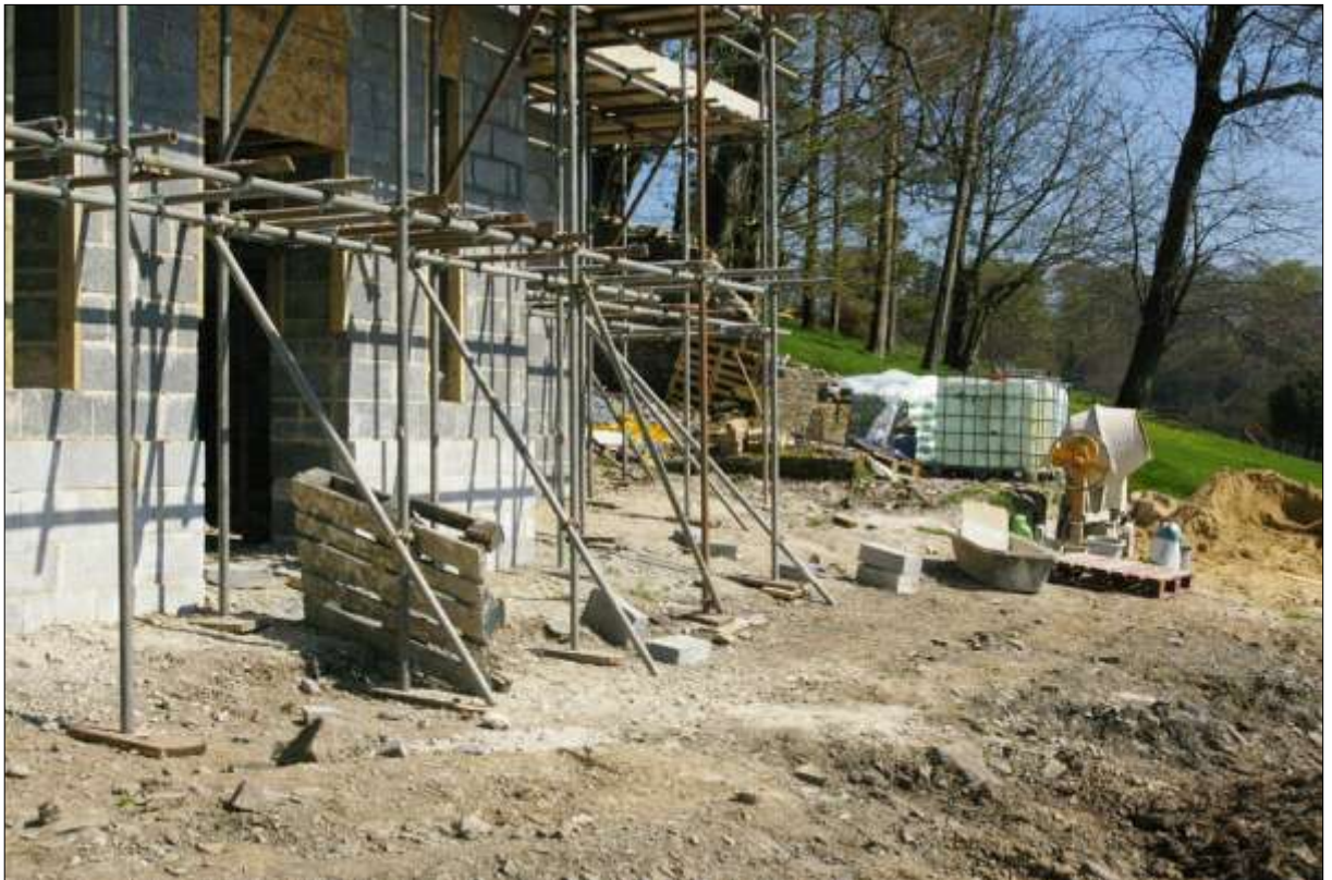
The south front of the new build, viewed from the south-west.
