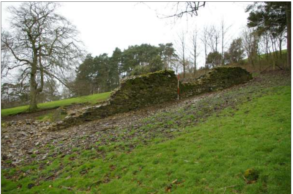
The east elevation, from the east.
