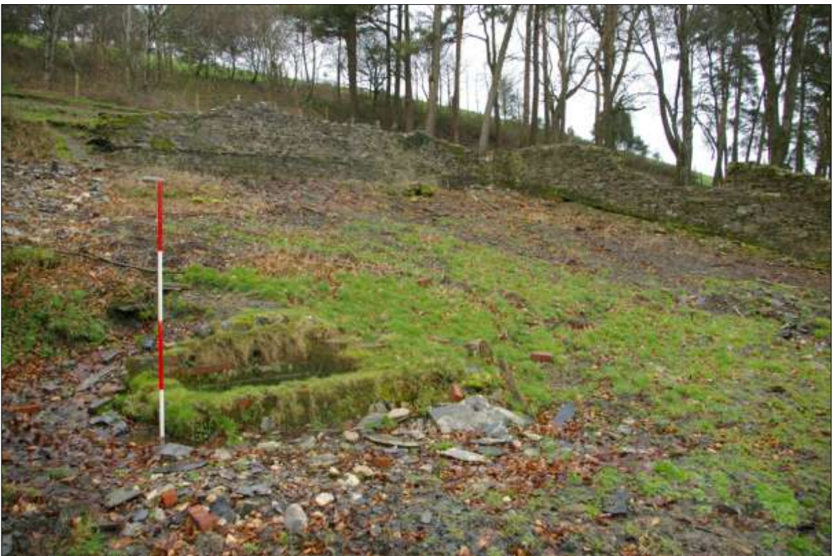
View across the water trough towards the north east corner of the structure, from the south-west.
