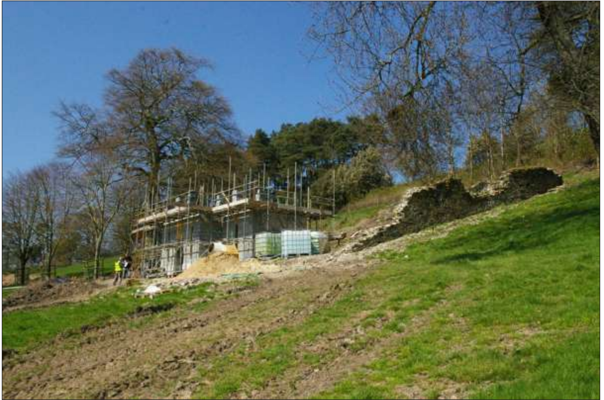
As above, viewed from the south-south-east.
