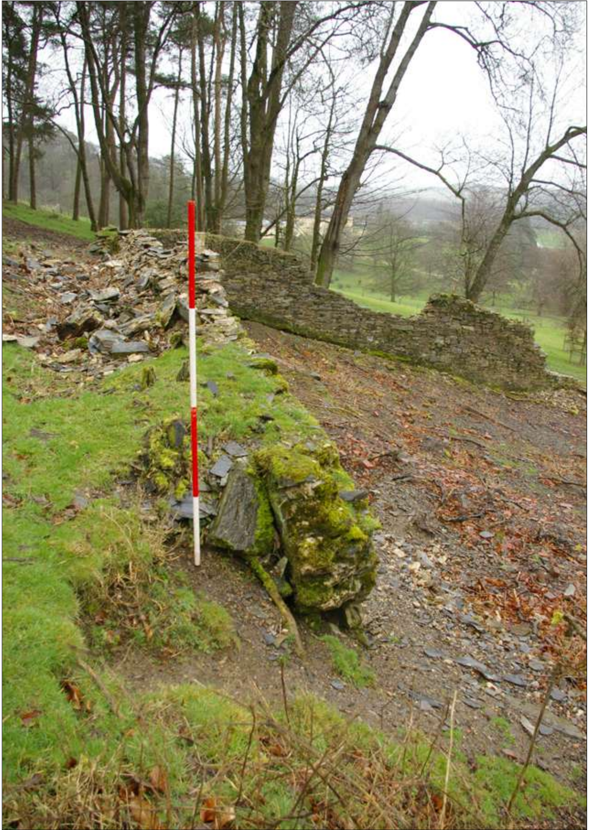
As above and also showing detail of the end of the upstanding section of the north elevation, from the west
