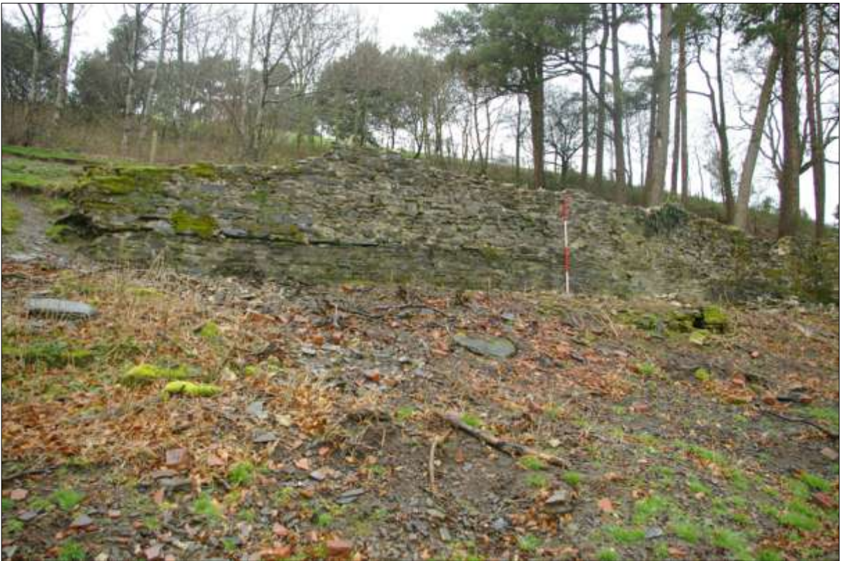
The northern elevation, from the south.
