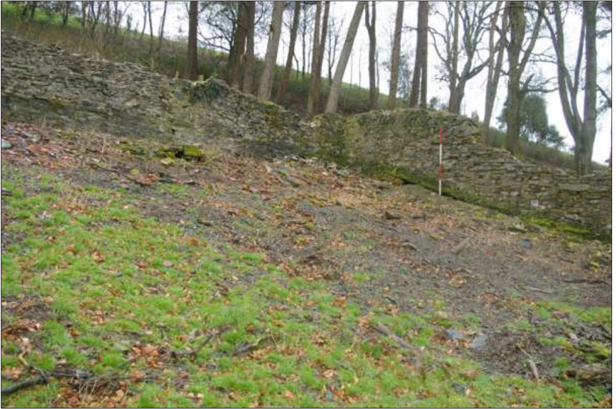
The north-east corner of the structure, from the south-west.
