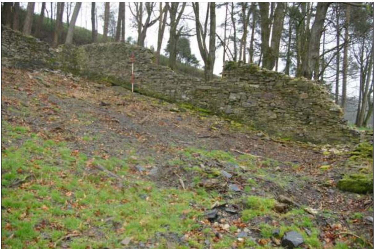
The east elevation, from the west.
