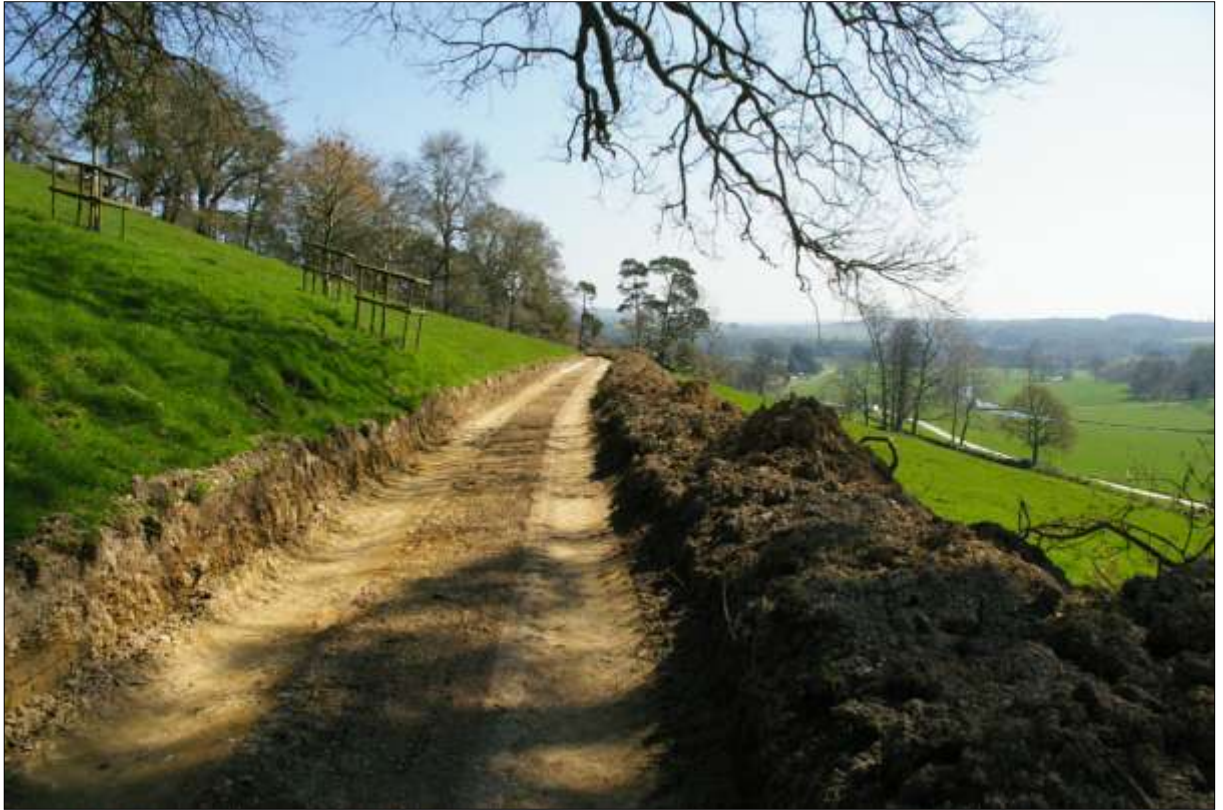
As above, looking east.
