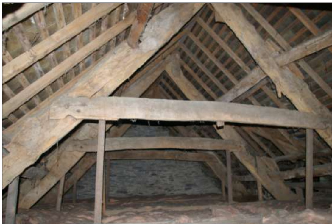
Figure 25: The 17 th century roof trusses, viewed from the south.
