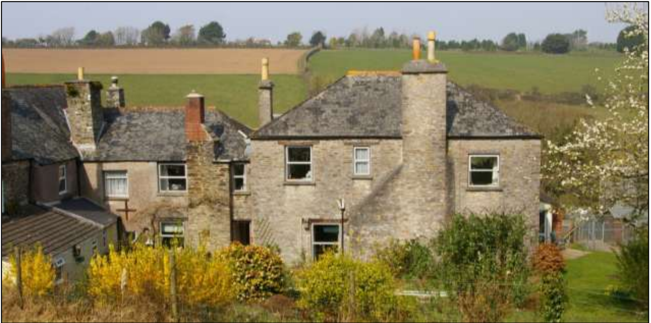
Figure 85: The south-facing elevation of the 20 th century Studio and the 19 th century block.
