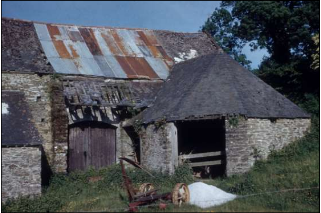
Figure 88: The west elevation of the Great Barn and Horse Engine House in 1960. Note the pentice over the western threshing door of the Barn (courtesy of Stanley Jones).
