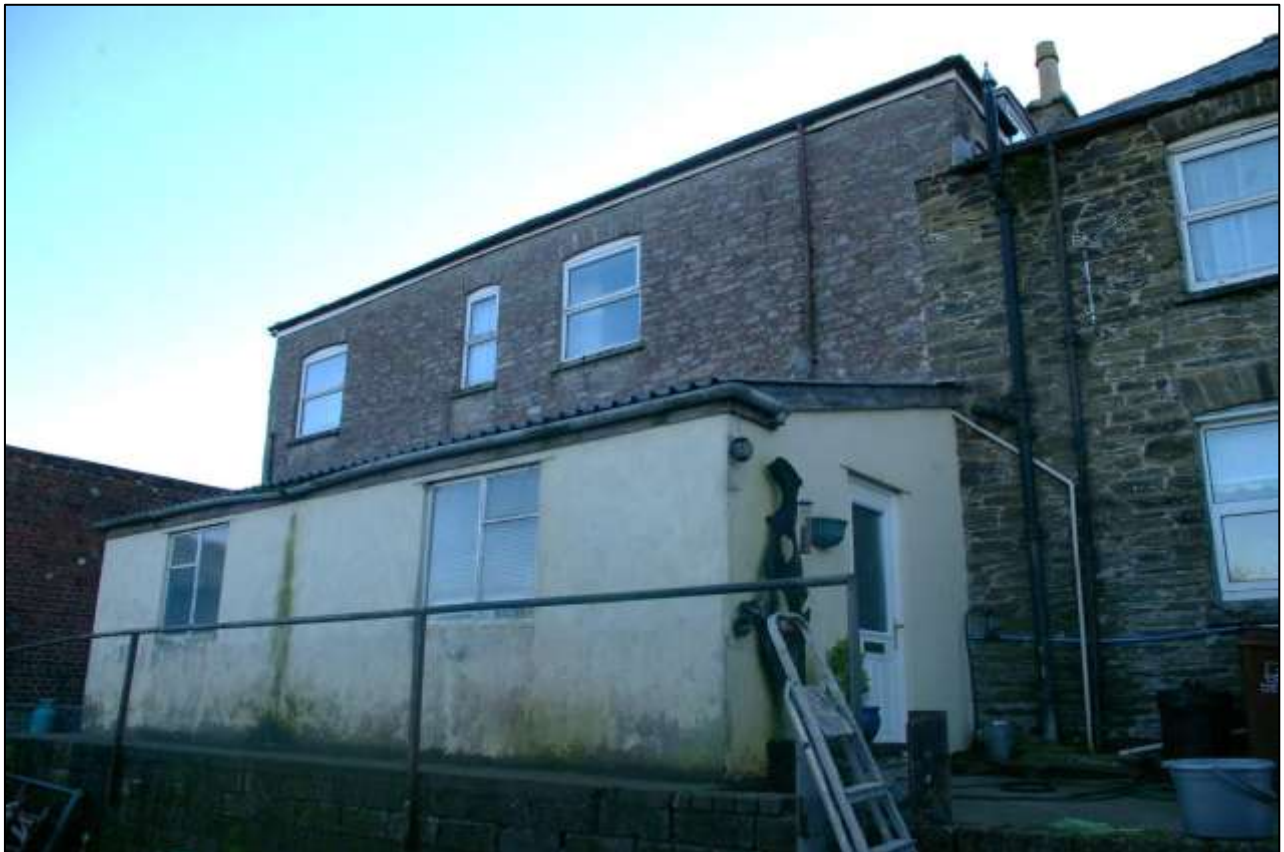
Figure 84: The north-facing elevation of the 20 th century Studio and modern outshut.
