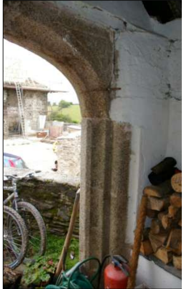
Figure 79: The inside of the porch, showing the internal face of the moulded doorway and spandrel panel.
