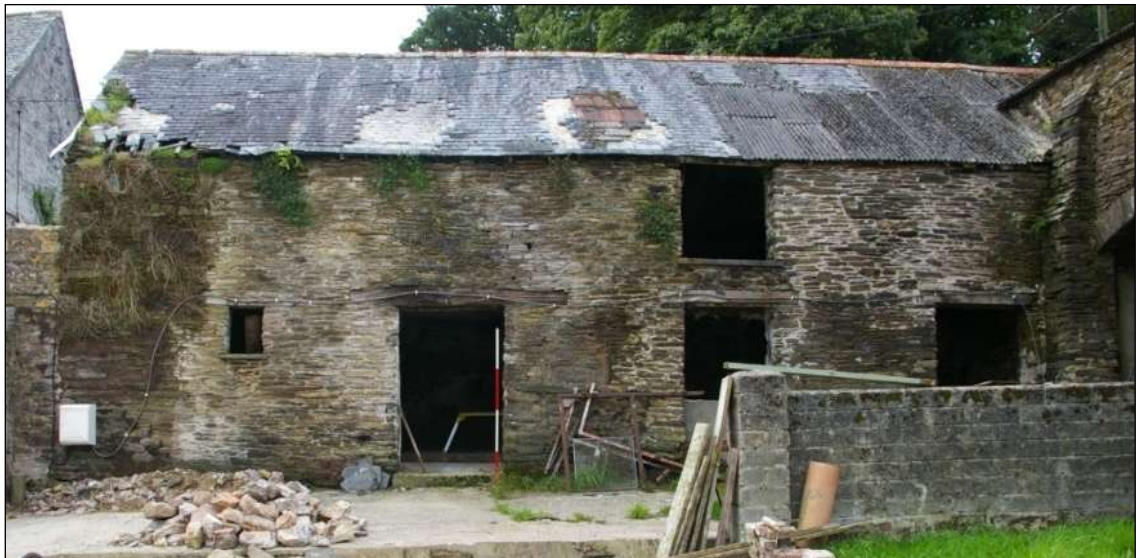
Figure 98: North elevation of the Stables, viewed from the north (scale 2m).
