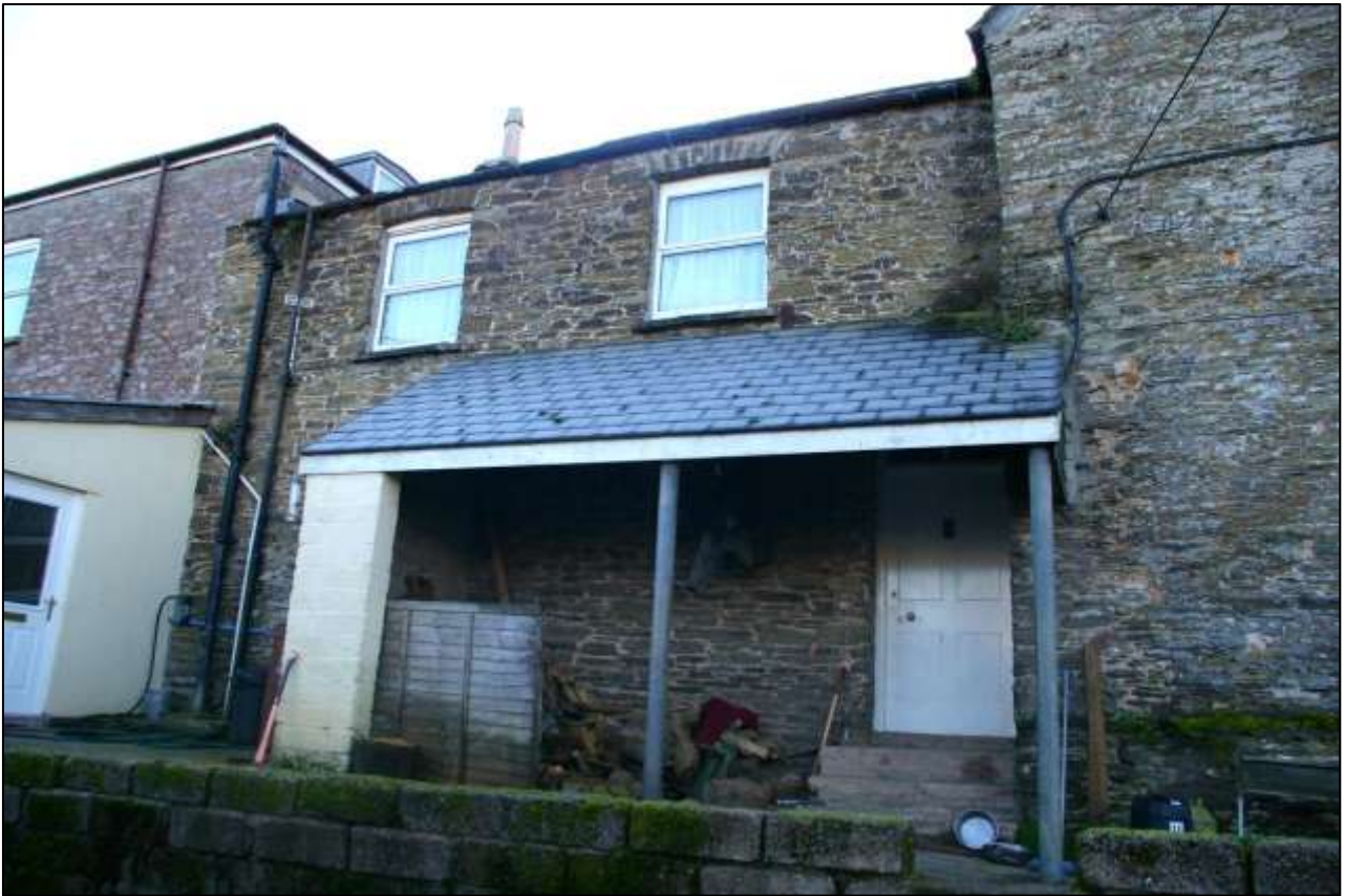
Figure 82: The north-facing elevation of the 19 th century block.
