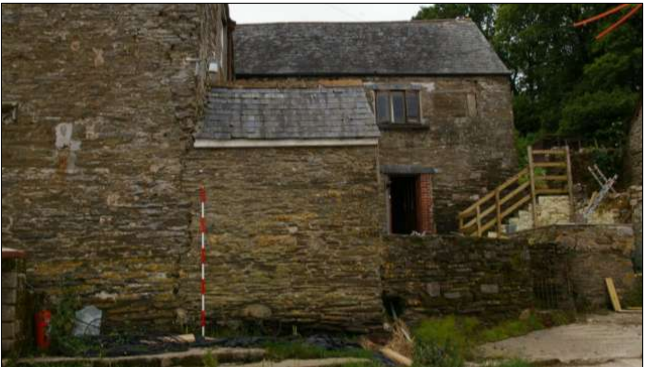
Figure 81: The north-facing elevation of the porch (scale 2m).
