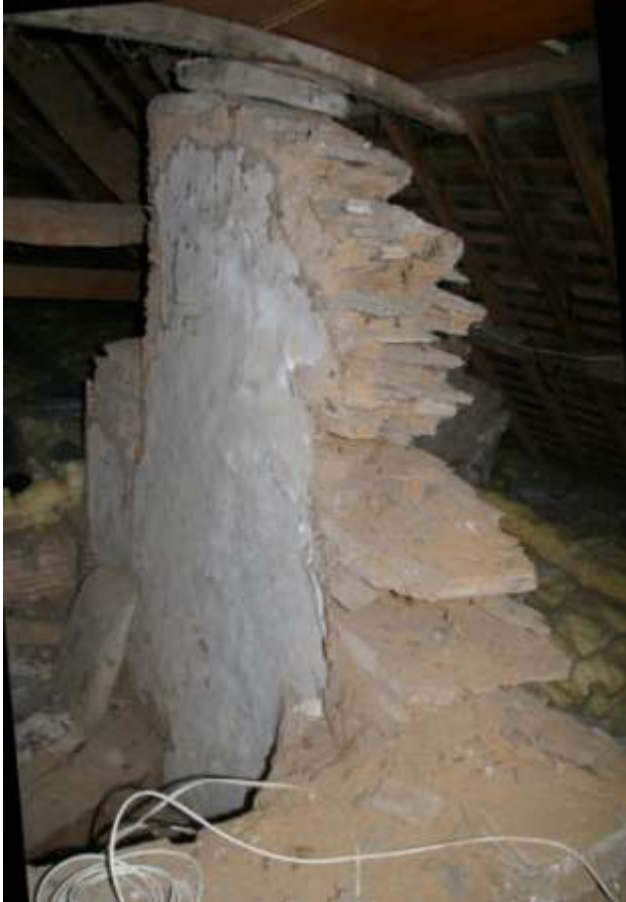
Figure 70: The south wall of the stairwell; viewed from the west.
