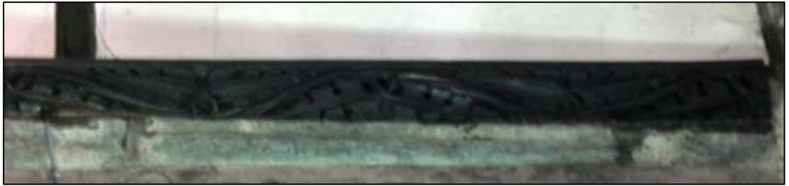
Figure 52: Detail of the scrolling vine-leaf decoration on the wallplate within the nave of Tavistock Church.
