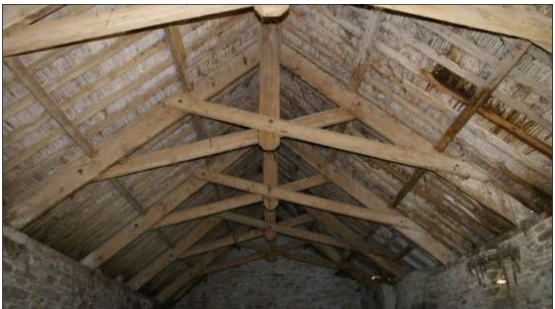
Figure 105: Roof structure of the Shippon, viewed from the west.
