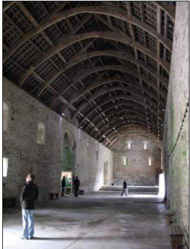
Figure 41: The interior of the barn at Buckland Abbey. Unlike the Great Barn at Coombe, the arch-braced roof rises from the wall plate and lacks wind-braces.
