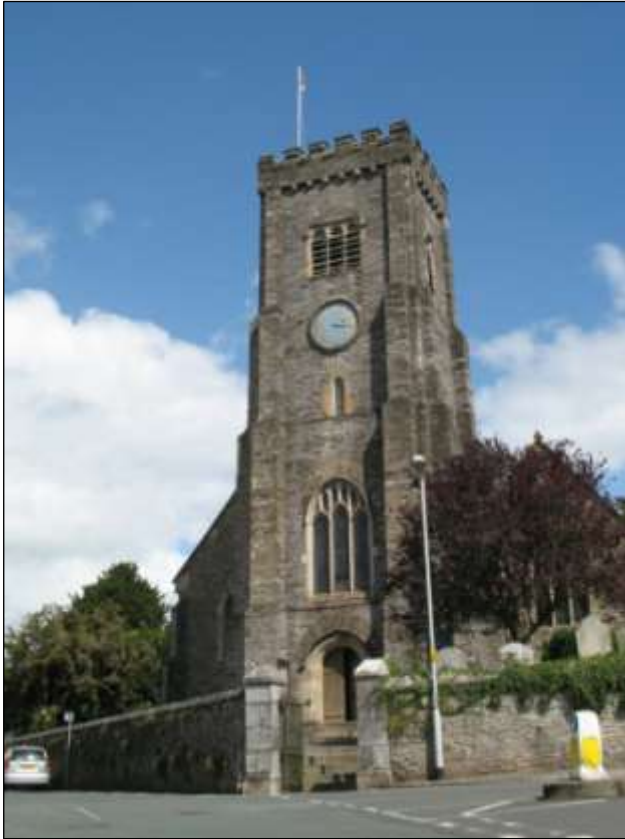
Figure 48: The tower at Plymstock Church; viewed from the south-west, looking north-east.
