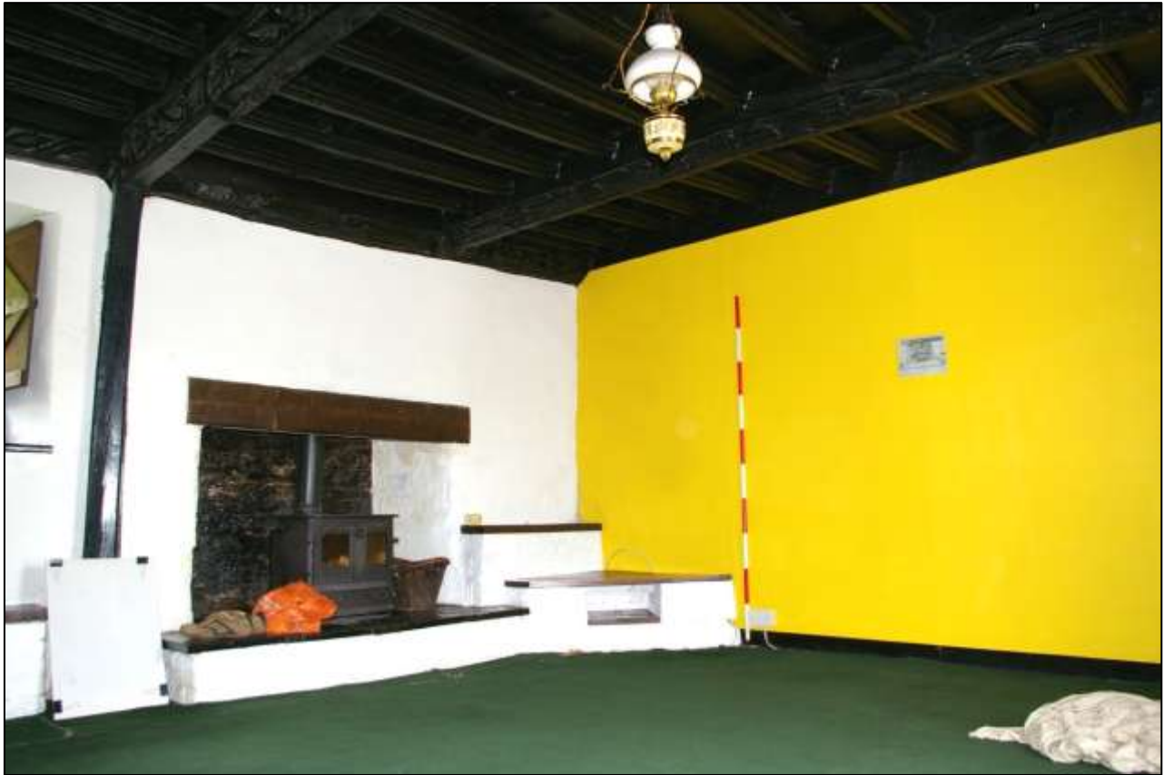
Figure 63: R1; viewed from the north-east, looking south-west (scale 2m).
