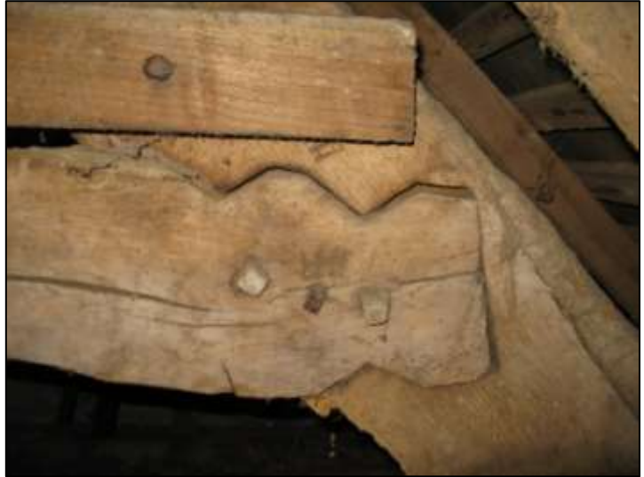
Figure 76: Detail of the complex notched half-lapped joints on the collars, and the chiselled carpenter's marks (Truss I, north blade).
