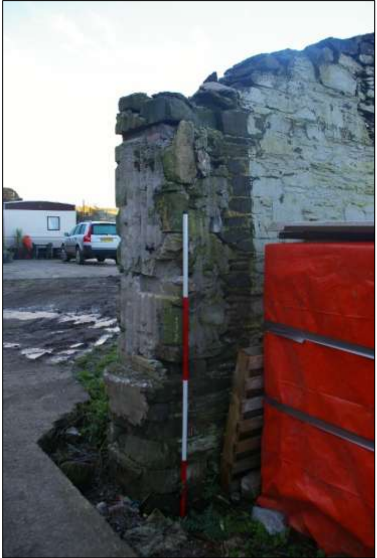
Figure 109: The western cartshed: the rounded end of the west gable (scale 2m).
