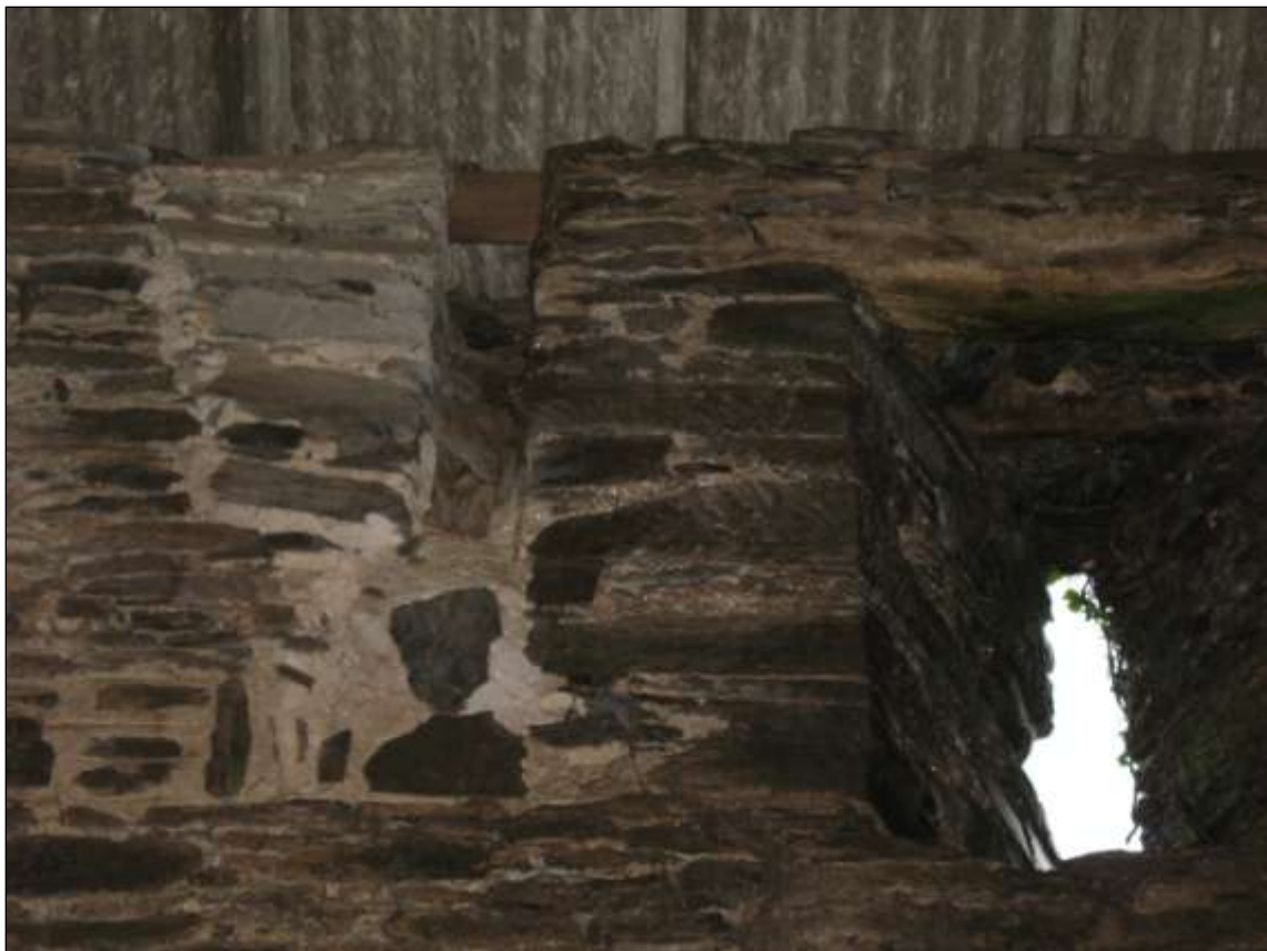
Figure 93: Detail of one of the asymmetric truss sockets and later infill.
