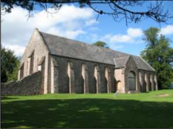
Top: Figure 43: The western gable end of the Spanish Barn at Torre Abbey, viewed from the north-west. Bottom: Figure 45: The south elevation of the Spanish Barn at Torre Abbey, viewed from the south-west.
