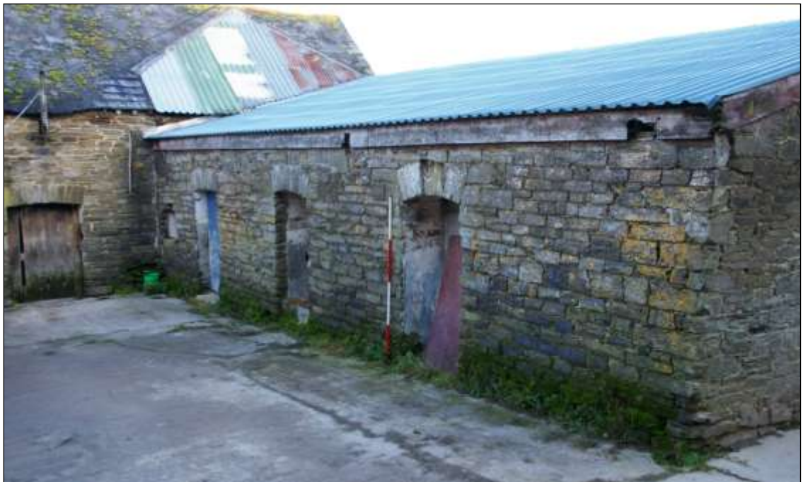
Figure 102: West elevation of Milking Parlour, viewed from the south-west (scale 2m).
