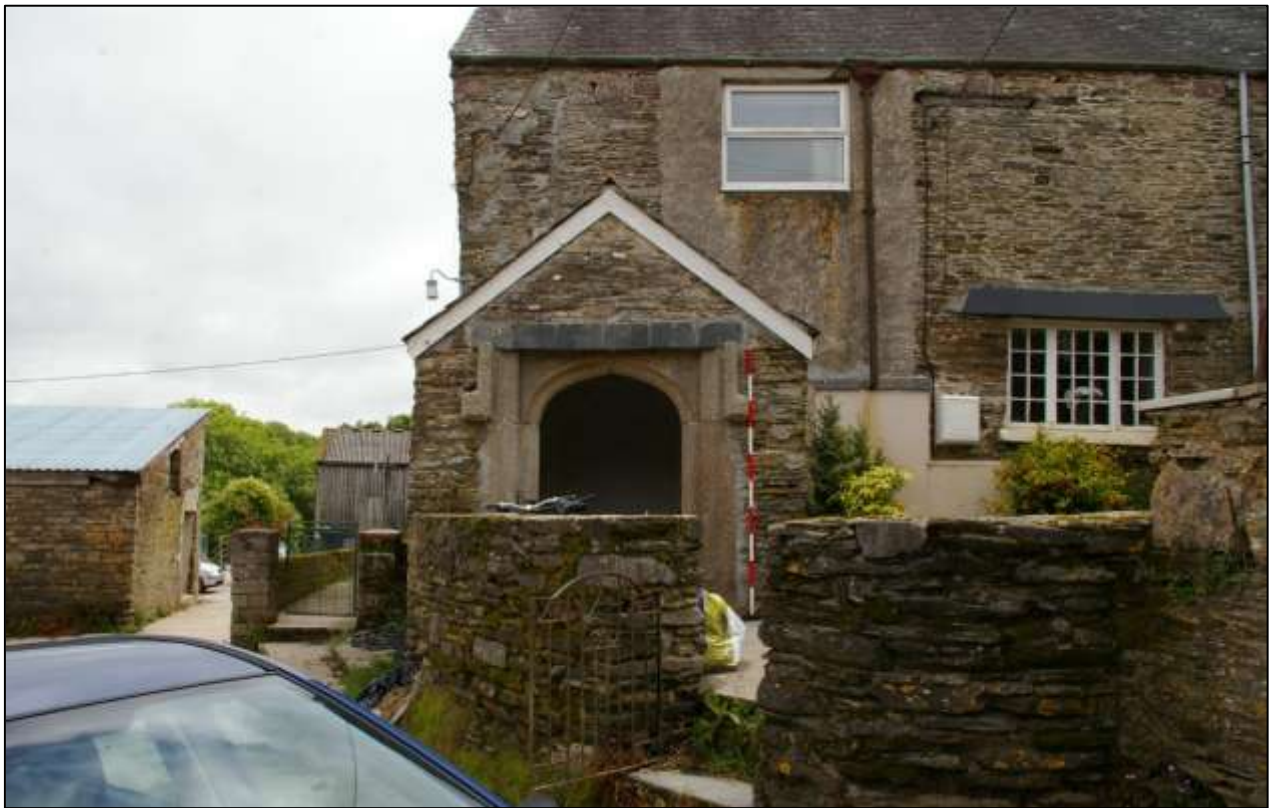
Figure 74: The west-facing elevation of the 17 th century block (scale 2m).
