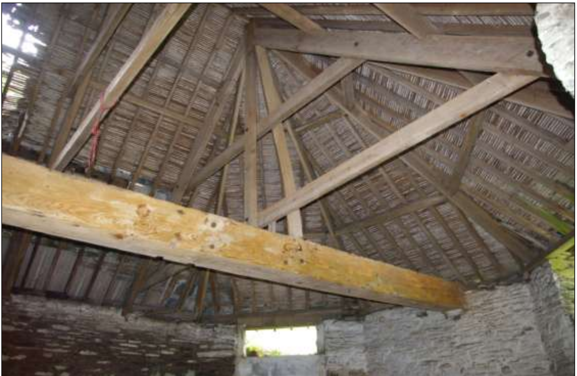
Figure 101: The interior of the Horse Engine House, viewed from the north-east.
