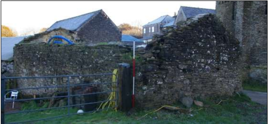
Figure 107: The western Cartshed; viewed from the north-west, looking south-east (scale 2m).
