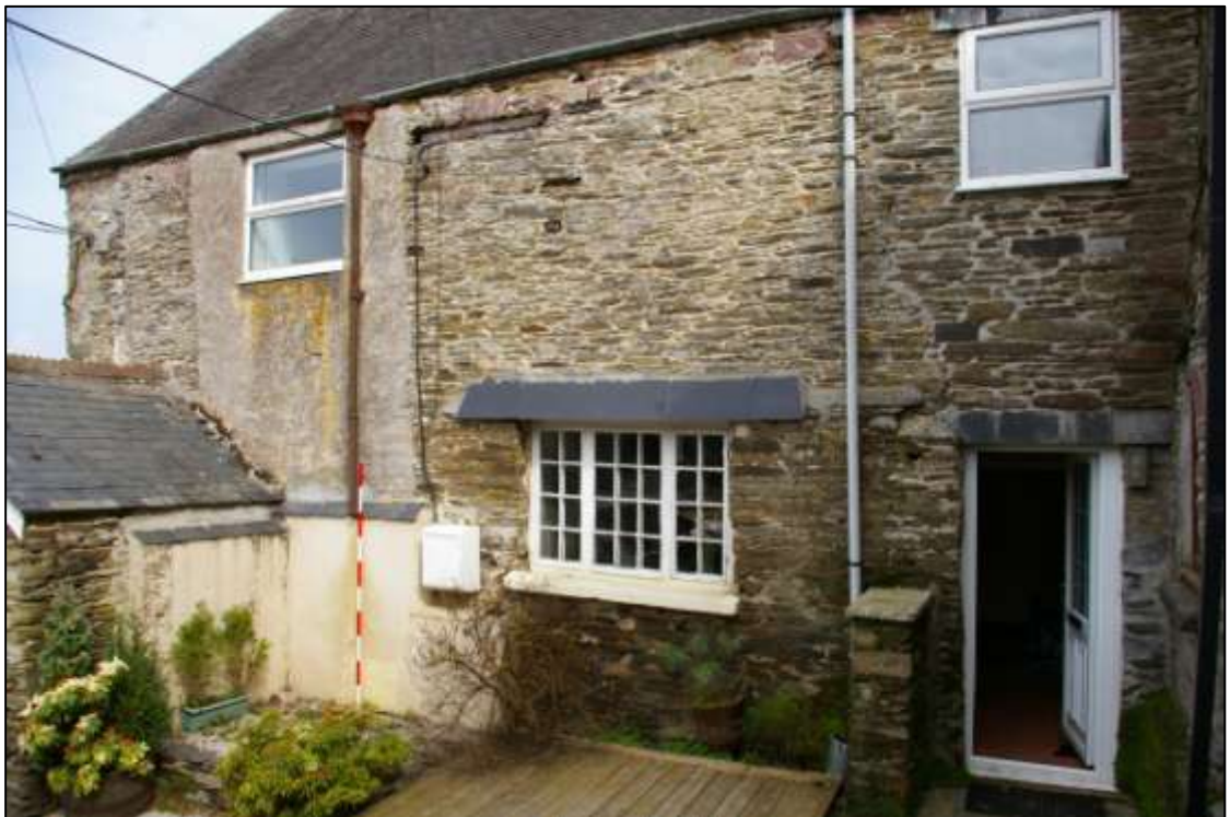
Figure 23: The west-facing elevation of the 17 th century block (scale 2m).
