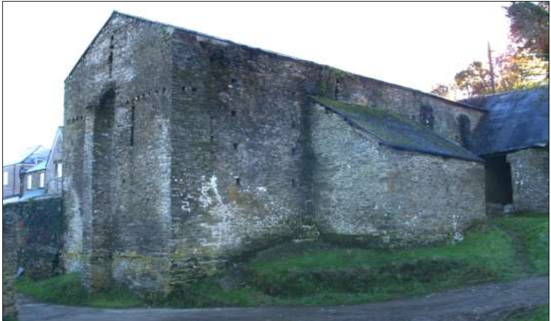
Figure 89: North and west elevations of the Great Barn, viewed from the north-west.
