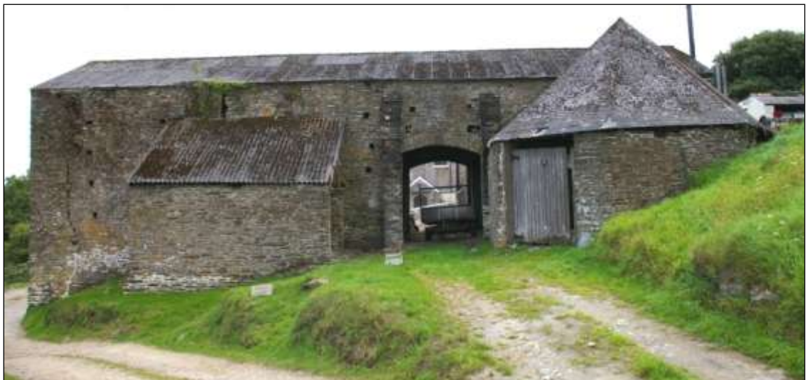
Figure 87: West elevation of the Great Barn, viewed from the west.
