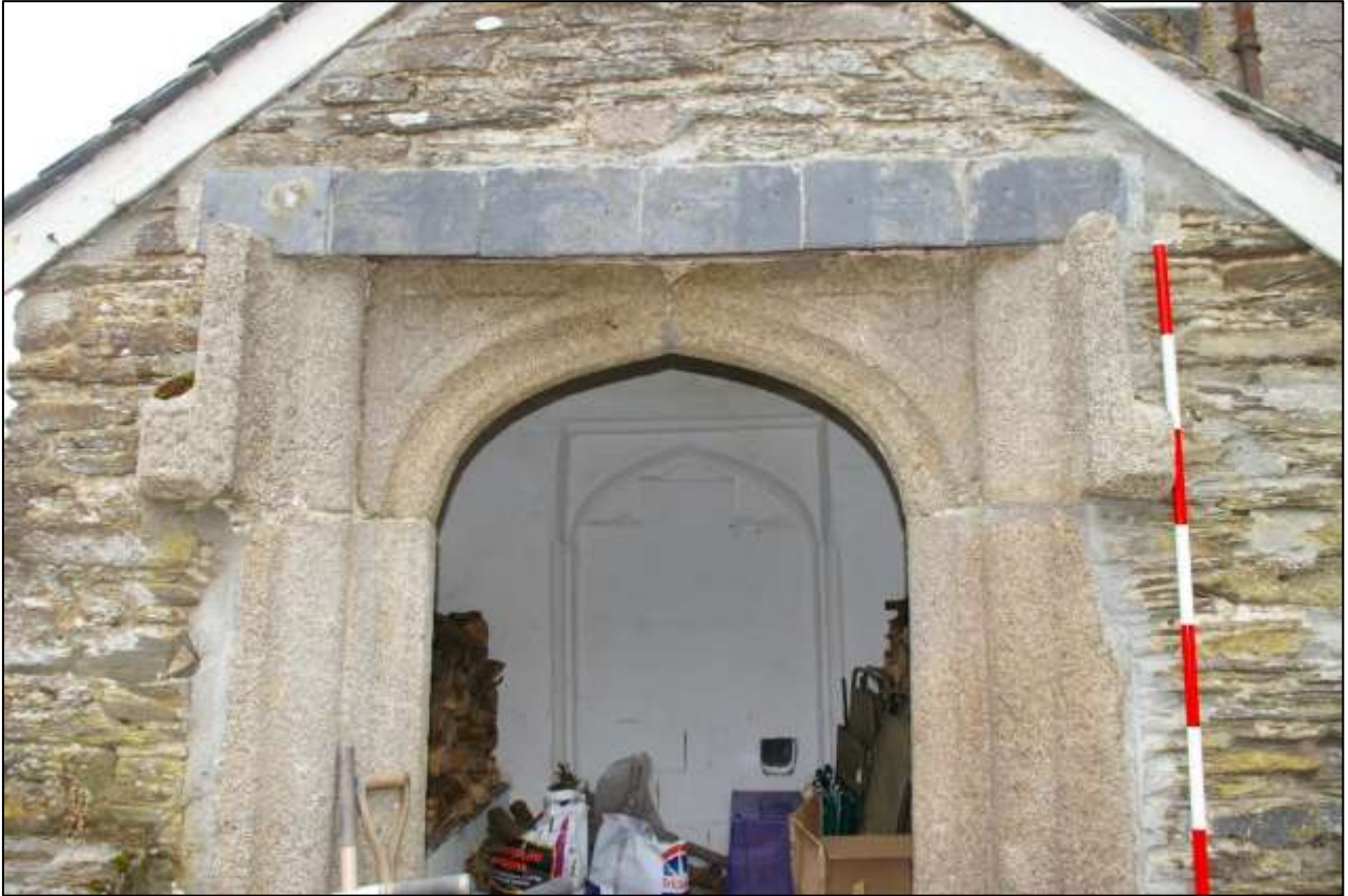
Figure 80: The granite-moulded doorway, showing the blocked internal doorway (scale 2m).
