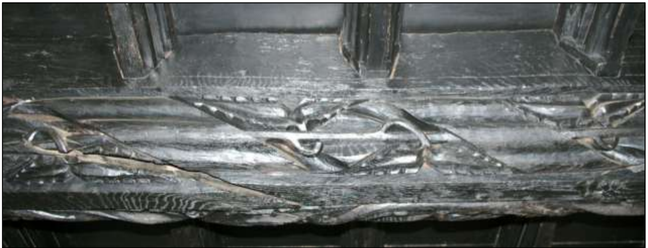
Figure 65: The west face of the eastern beam, Style 2.
