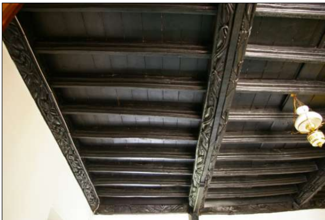
Figure 21: The carved beams in R1; the eastern beam and Style 4 wallplate; viewed from the north.
