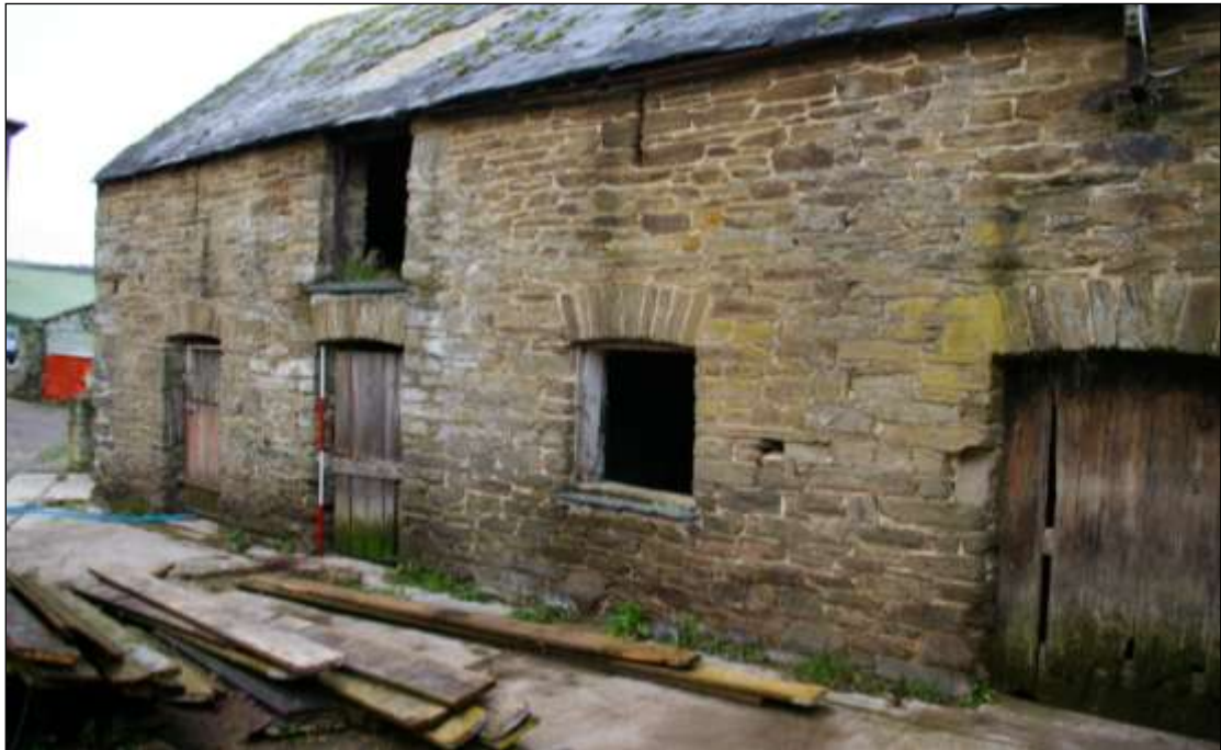
Figure 103: South elevation of the Shippon, viewed from the south-east (scale 2m).
