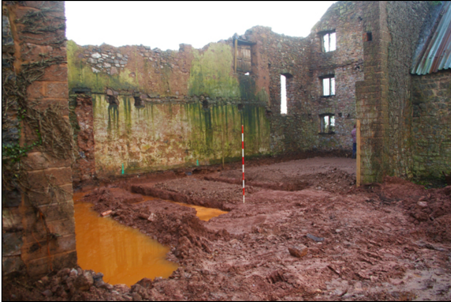
Figure 2: Mill during renovation groundworks, viewed from west (2m scale).
