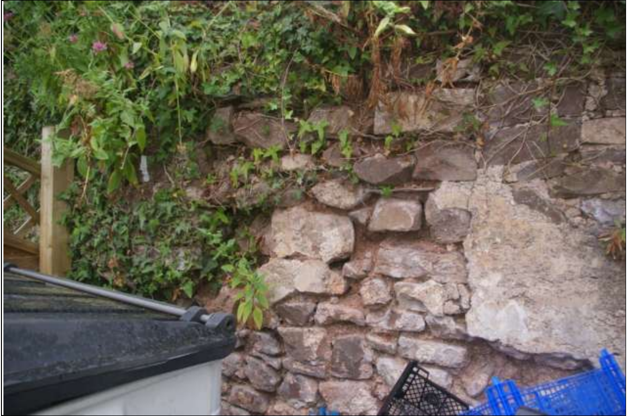
Shot of wall behind the bin store, western end (no scale).
