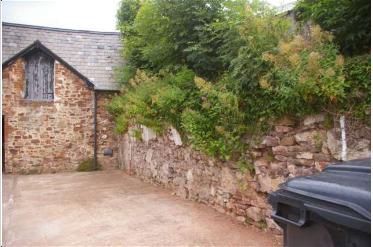
General shot of wall, viewed from the east-north-east (1m scale).
