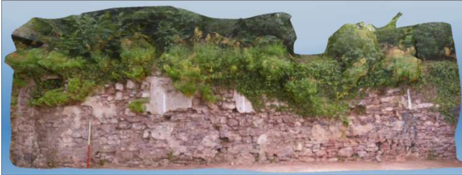
Figure 12: The north-facing elevation of the wall (rectified image produced using Autodesk 123D Catch imaging software).
