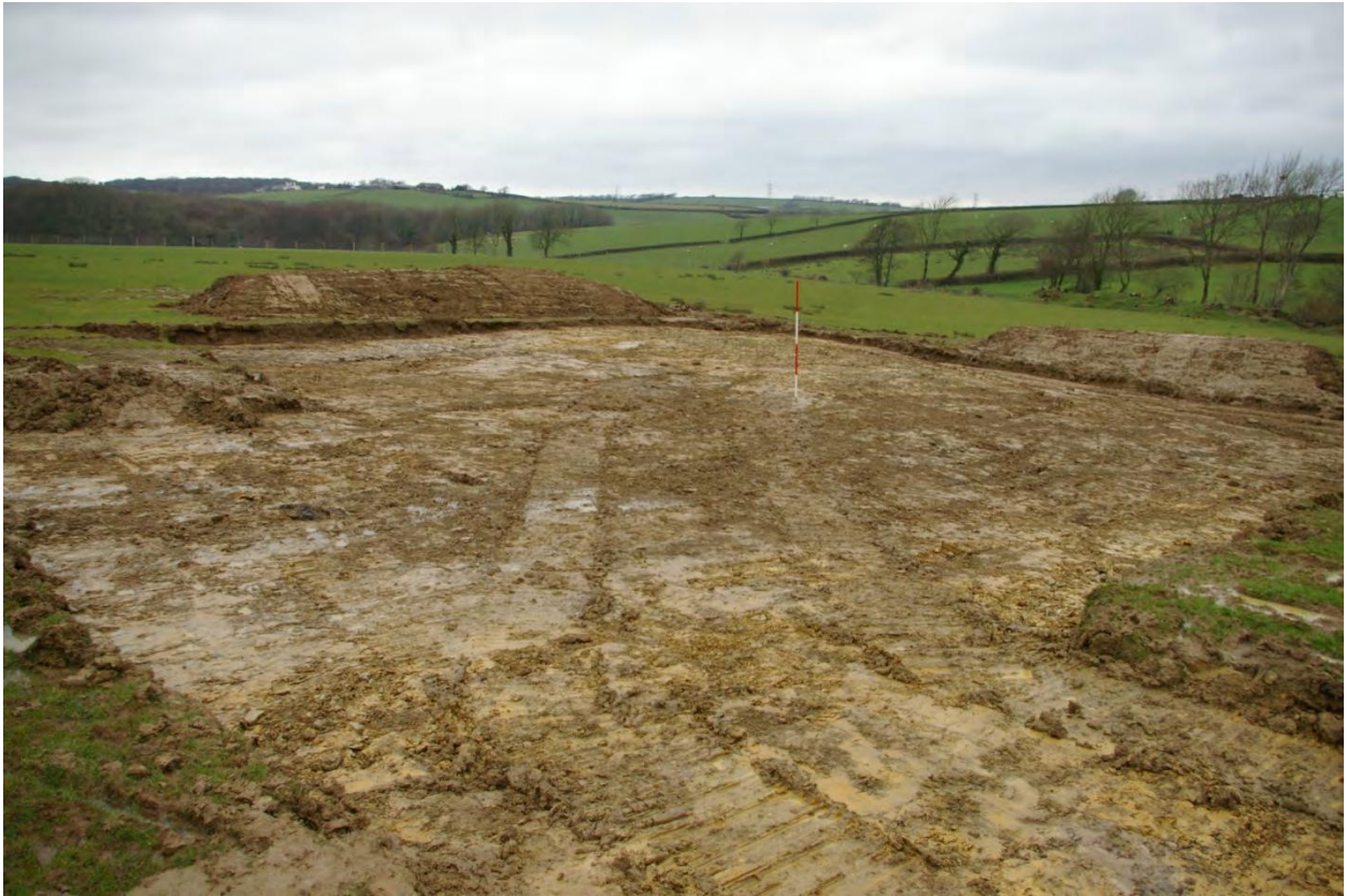
Post-excavation, compound area; from the south-east, 2m scale.
