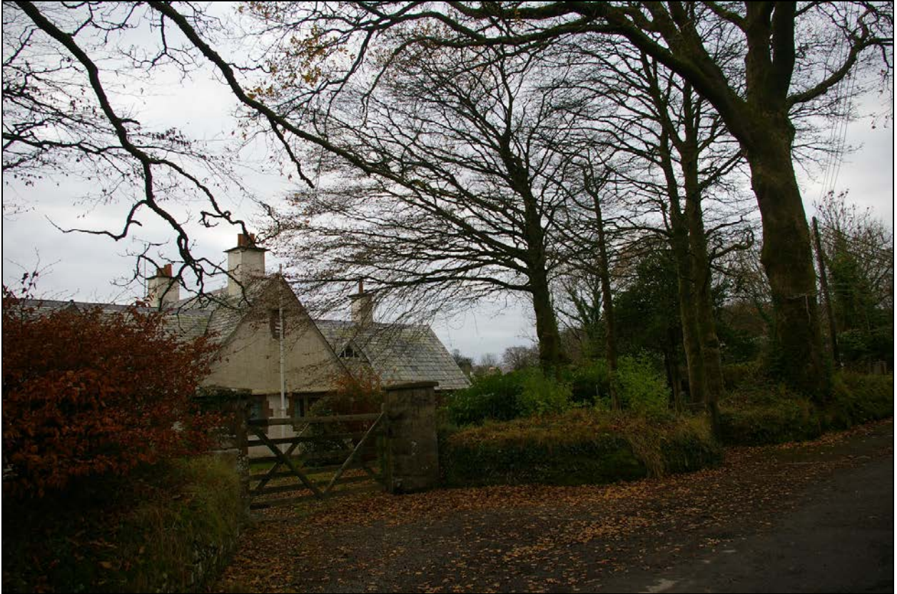
Winsford Hospital, Halwill Junction, a low single storey building, shielded by the trees which line its boundary; from the north-east.
