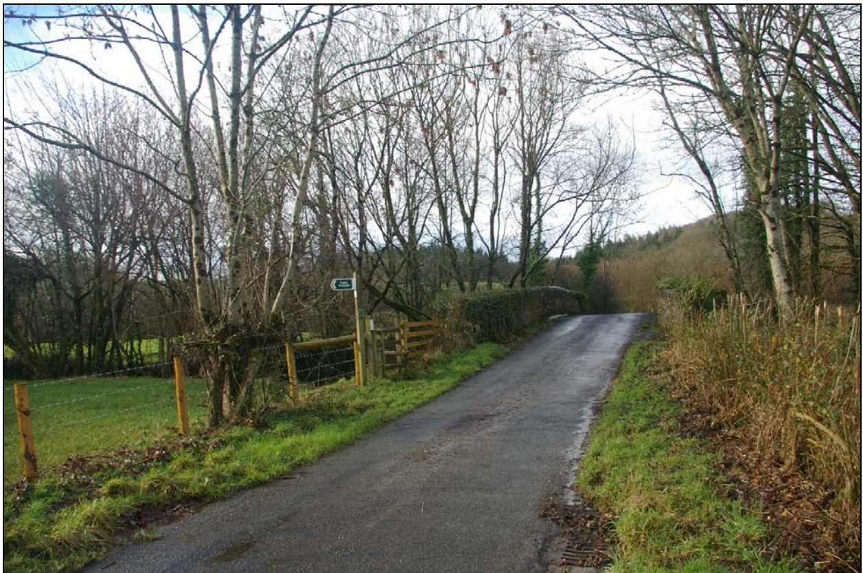
Lewer Bridge, Hatherleigh, set in a wide valley north-east of the town, with views down the valley to the south, towards the proposed turbine site; from the north-east.
