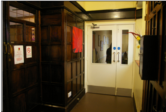
Figure 26: The western door leading from the entrance porch G16, with panelled cupboard to north, from the north-east.
