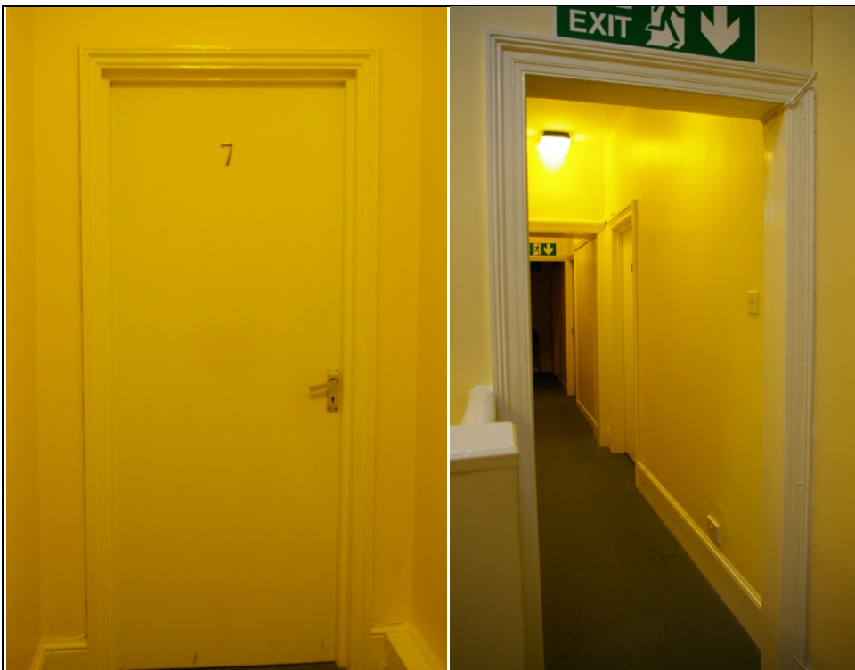
Figure 18: The door into F14, with moulded architrave as to rooms F15 & F16, from the south.
