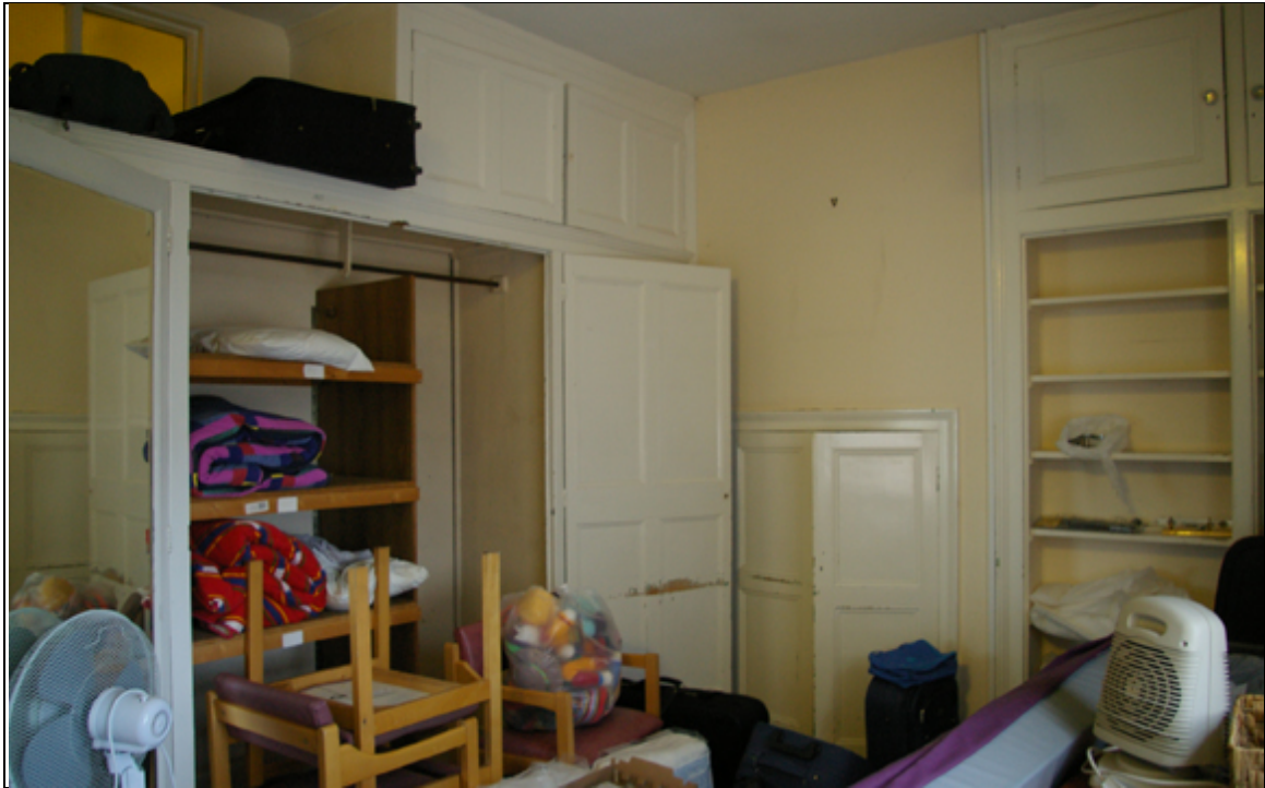
Figure 14: The north-east corner of former dressing room F12, from the south-west.
