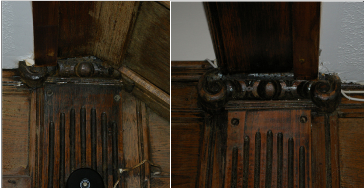
Figure 29: Detail of ionic capital of pilaster beneath the stair and landing on the west wall of G17, from the east. Figure 30: Detail of ionic capital of pilaster below the landing rail on the east wall of G17, from the west.
