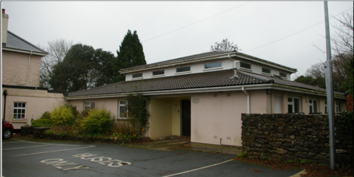
Figure 38: The north and east elevations of Fairwinds , from the north-east.
