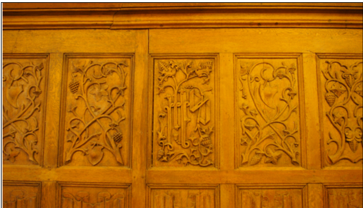
Figure 12: Detail of the panelling on the north wall of G23 with central monogram, from the south.
