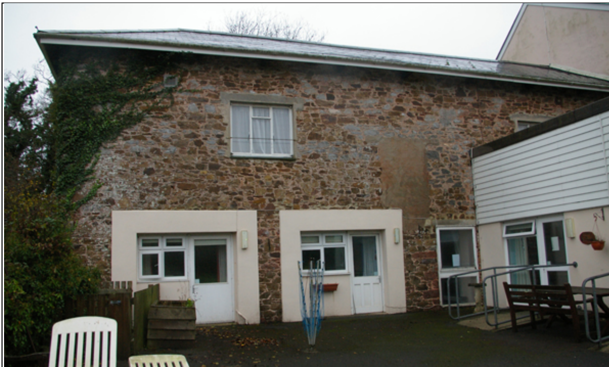
Figure 35: The east elevation of the former stable block to the south of the house, from the east.
