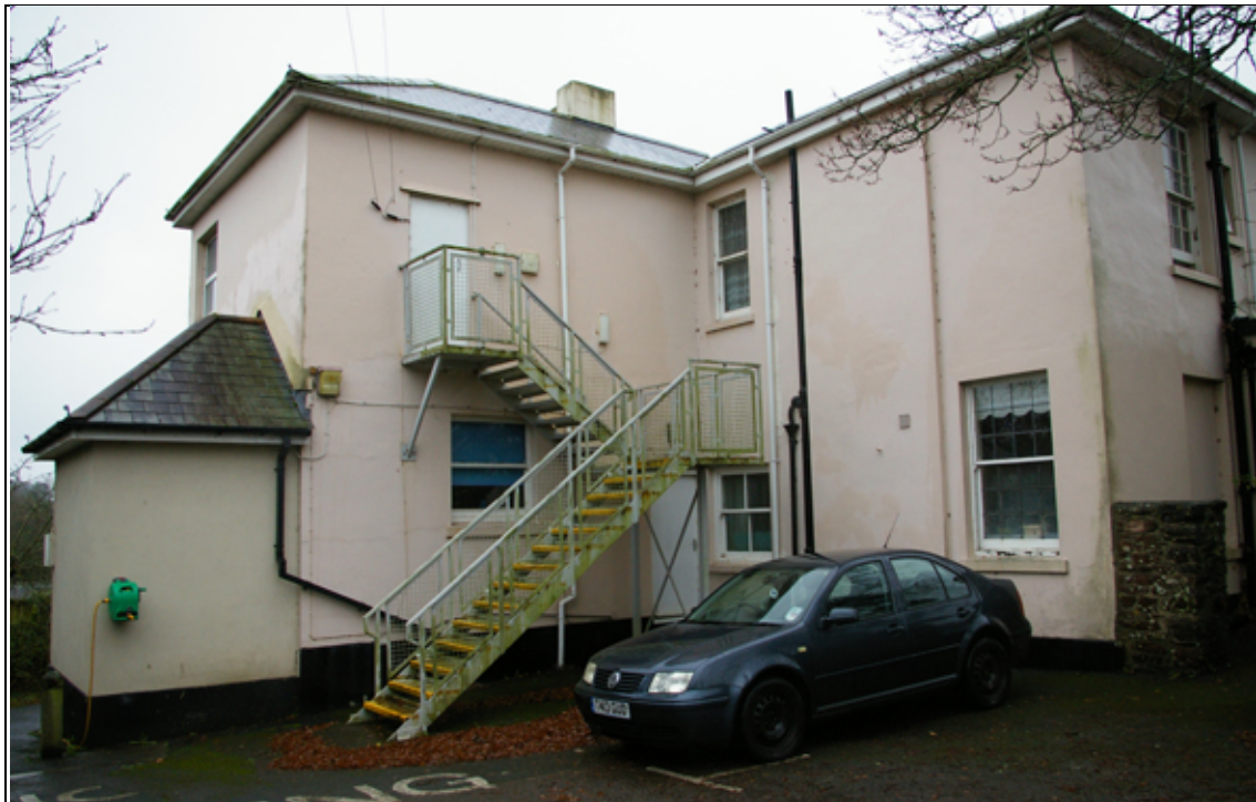
Figure 37: The north-eastern end of Occombe House, from the north-east.
