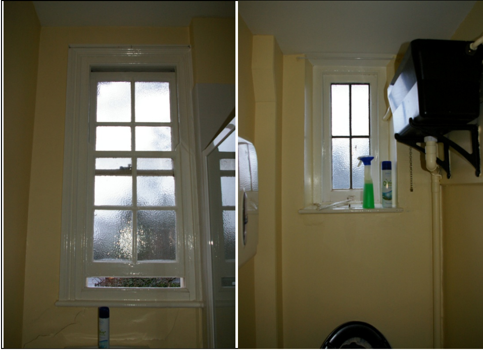
Figure 20: Window in toilet F08, from the south.
