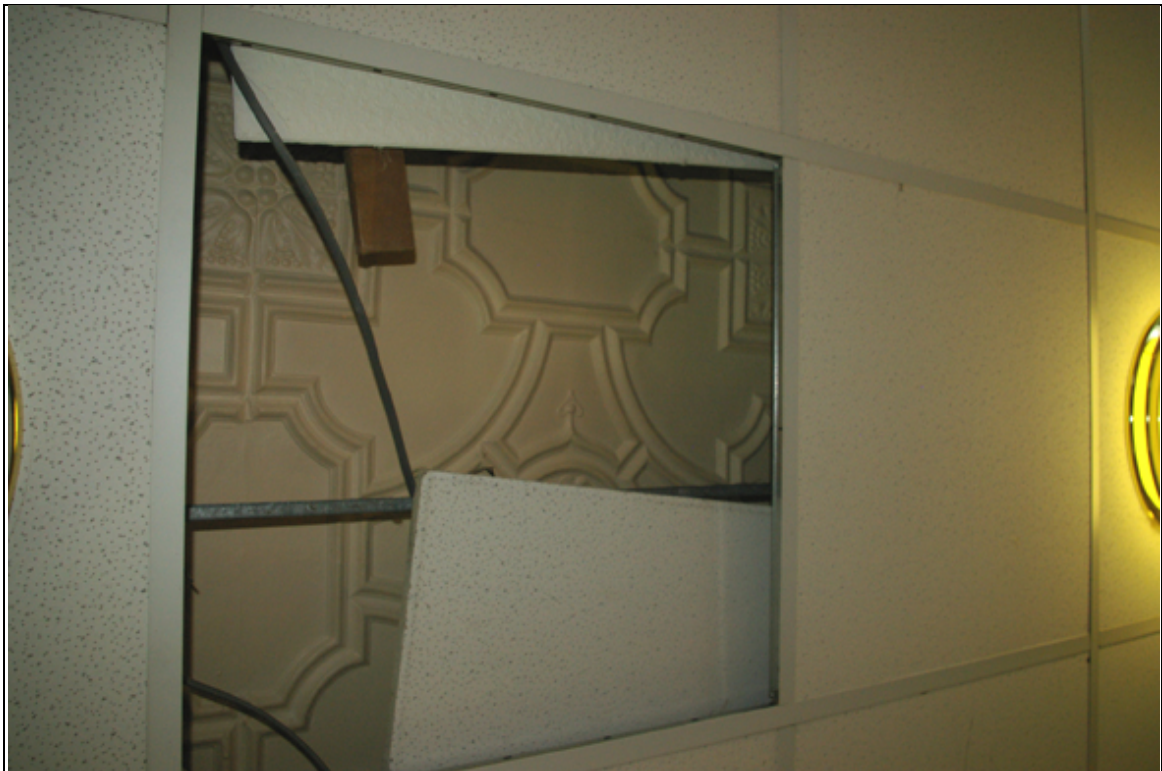
Figure 10: A small portion of the moulded plaster ceiling, above the modern ceiling in G22.
