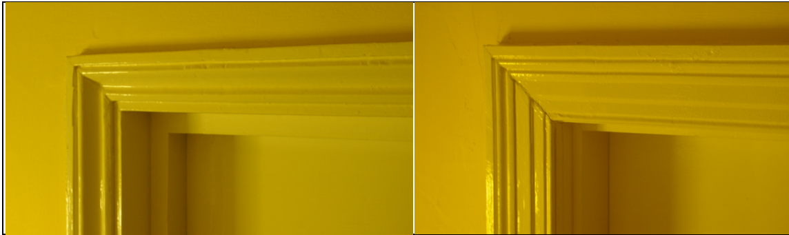
Figure 13: Left – The architrave type of door frames to rooms F14, F16 and F17 (interior). Right - The architrave type of door frames to rooms F01, F04, F07, F08, F10, F12 & F17 (exterior).
