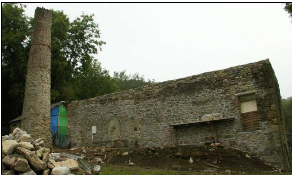
Figure 14: The west elevation of the engine house and the chimney; viewed from the north-west from downslope (no scale).
