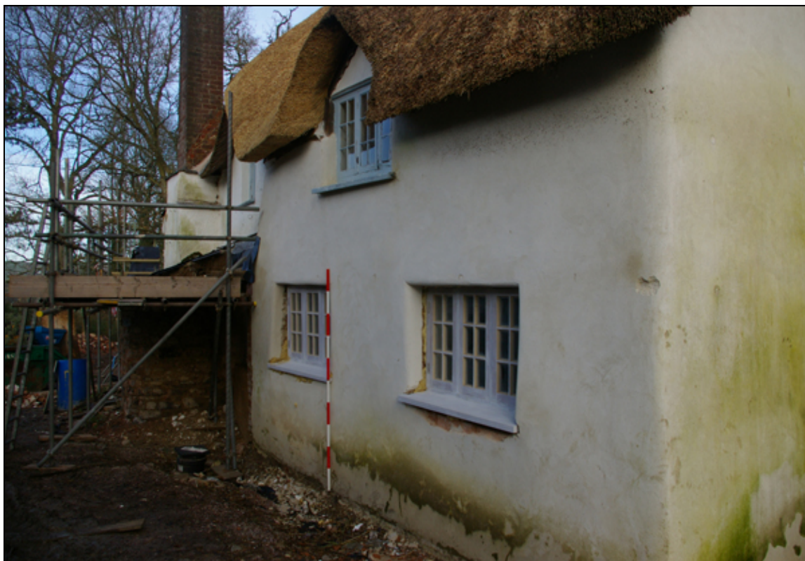
Figure 19: East end of south elevation, viewed from south-east (2m scale).
