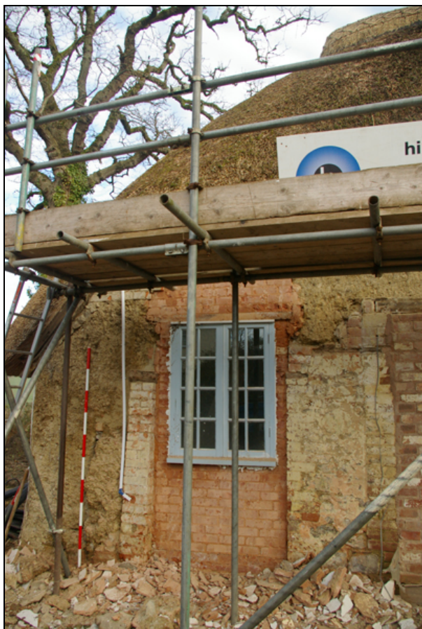
Figure 20: west end of south elevation, viewed from south (2m scale).
