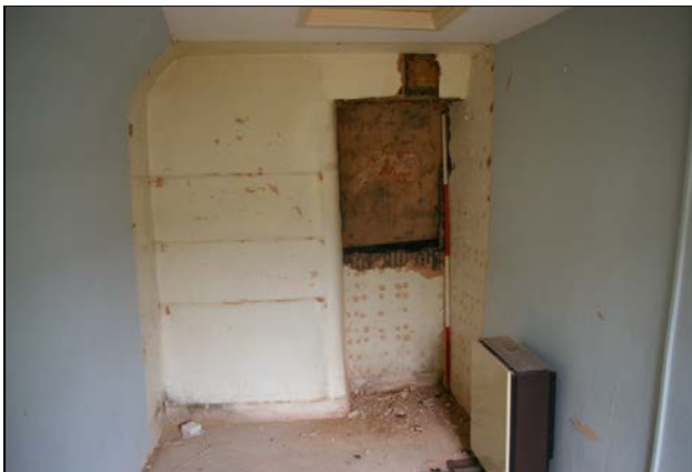
Figure 4: Room 1, viewed from South (2m scale).
