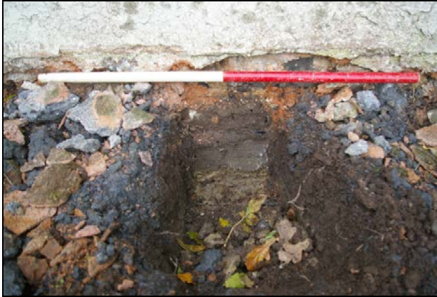
Figure 15: Test Pit 3, establishing depth of north elevation foundations, viewed from north (1m scale).
