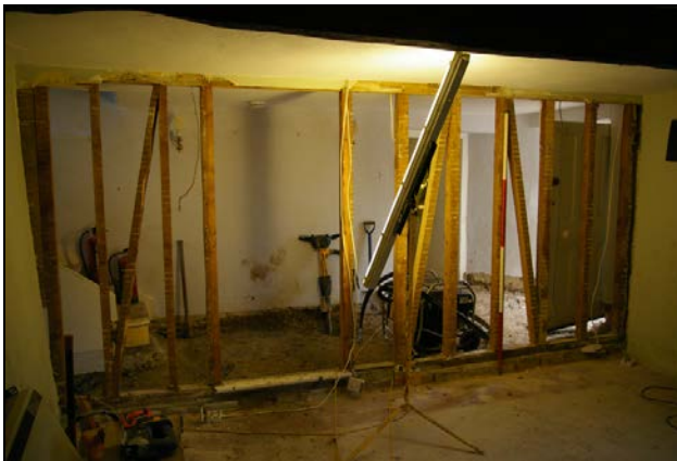
Figure 8: Room 4, viewed from north-west (2m scale).
