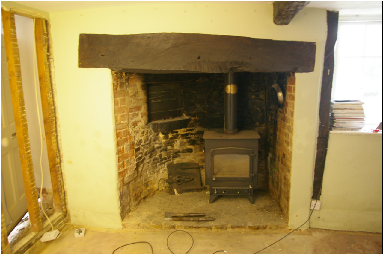
Figure 10: Room 4, fire place and oven, viewed from north (no scale).
