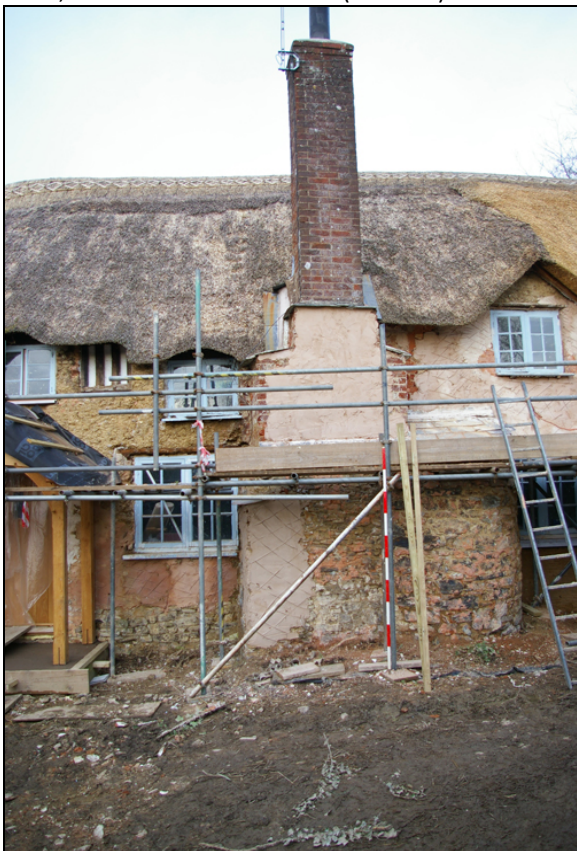
Figure 24: chimney stack and oven exposed viewed from south (2m scale).
