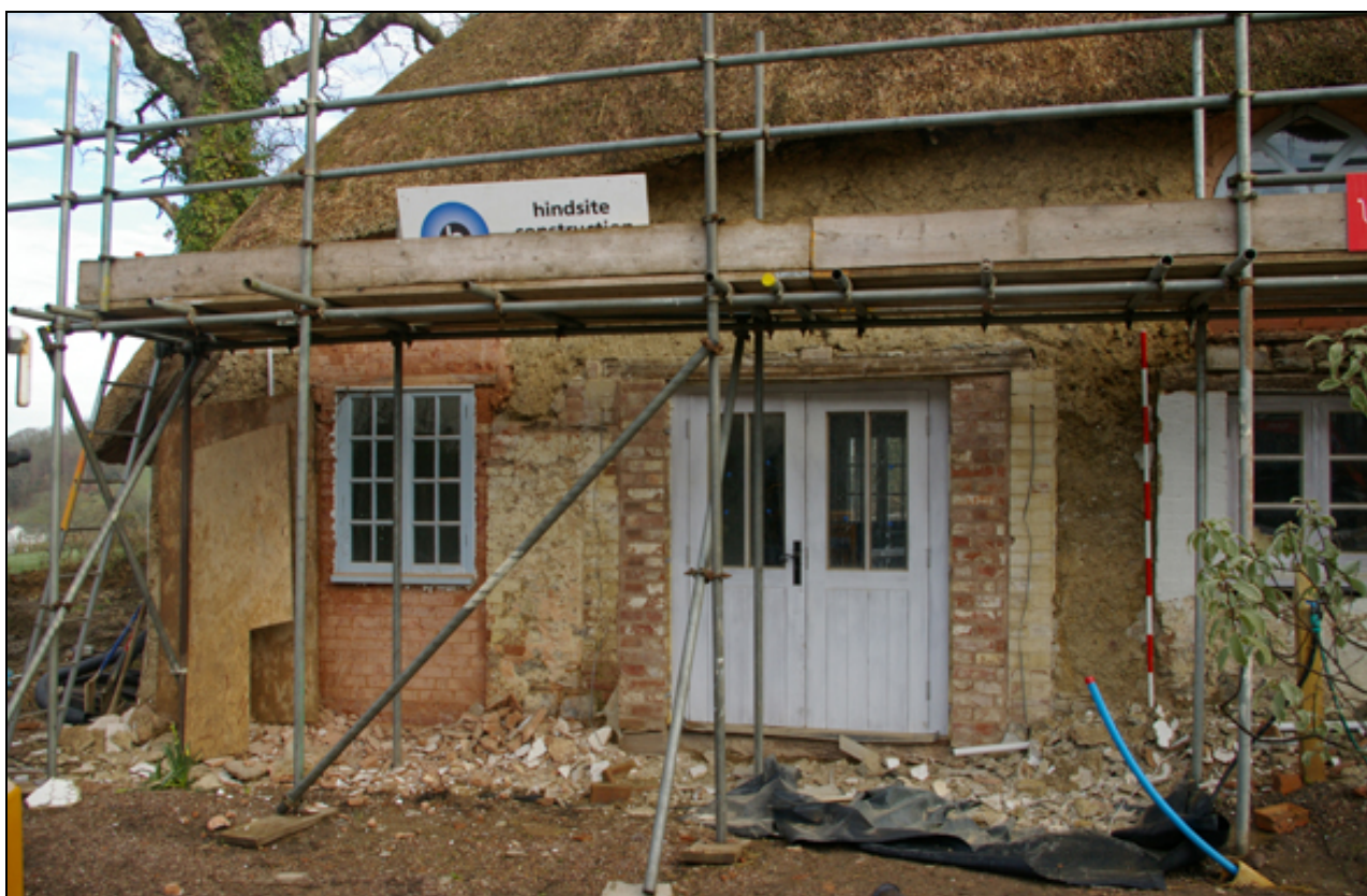
Figure 18: Exposed west end of south elevation, viewed from south-east (2m scale).
