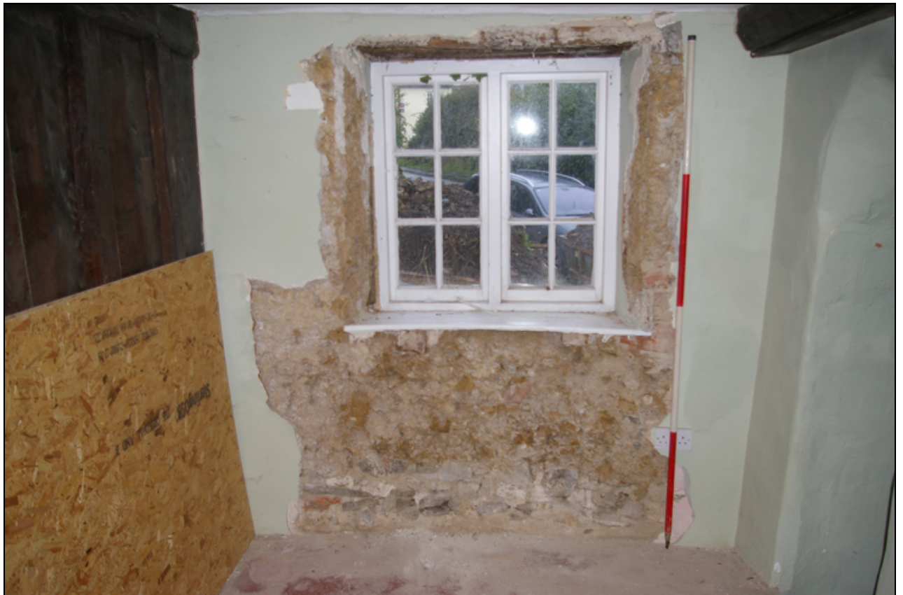
Figure 6: Room 3, south wall, viewed from north (2m scale).
