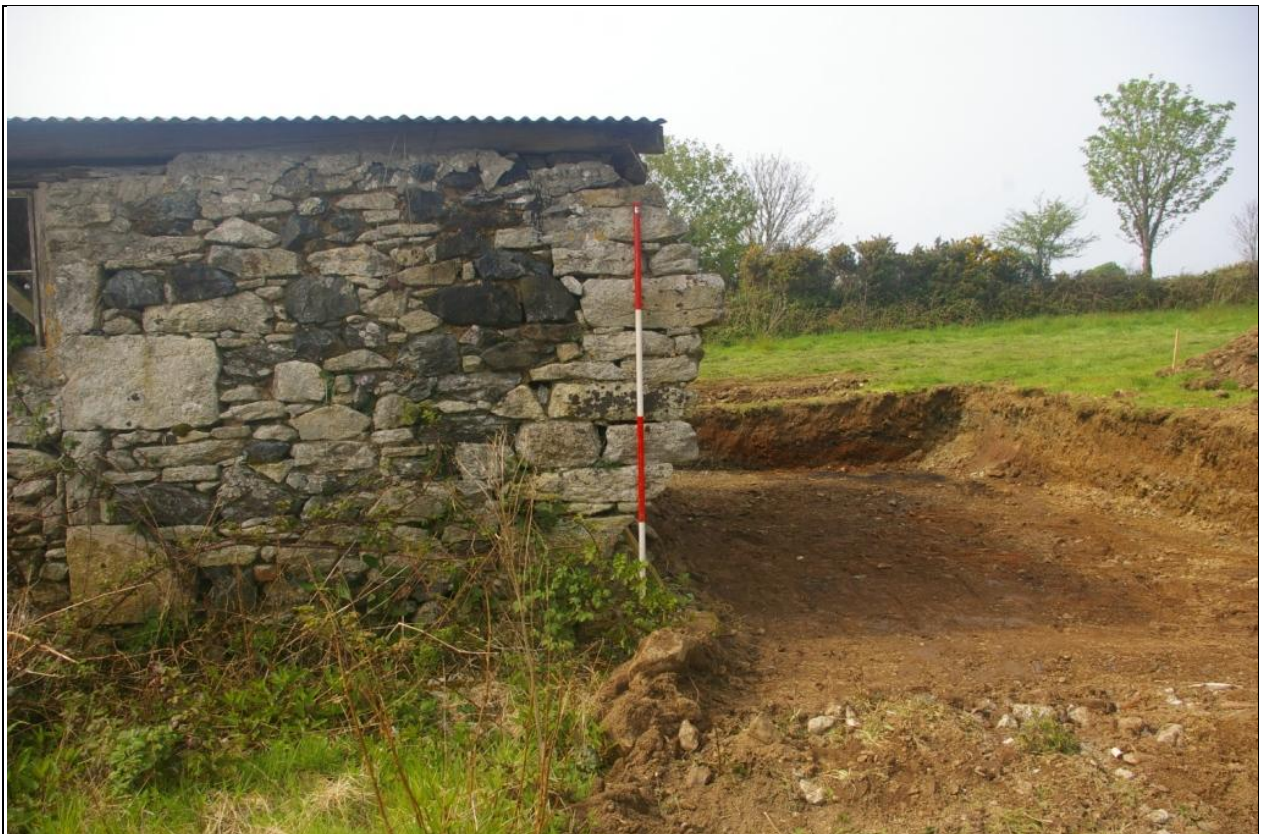
DETAIL OF THE RAGGED EDGE TO THE EAST OF THE SOUTH FACING ELEVATION, VIEWED FROM THE SOUTH (2M SCALE).
