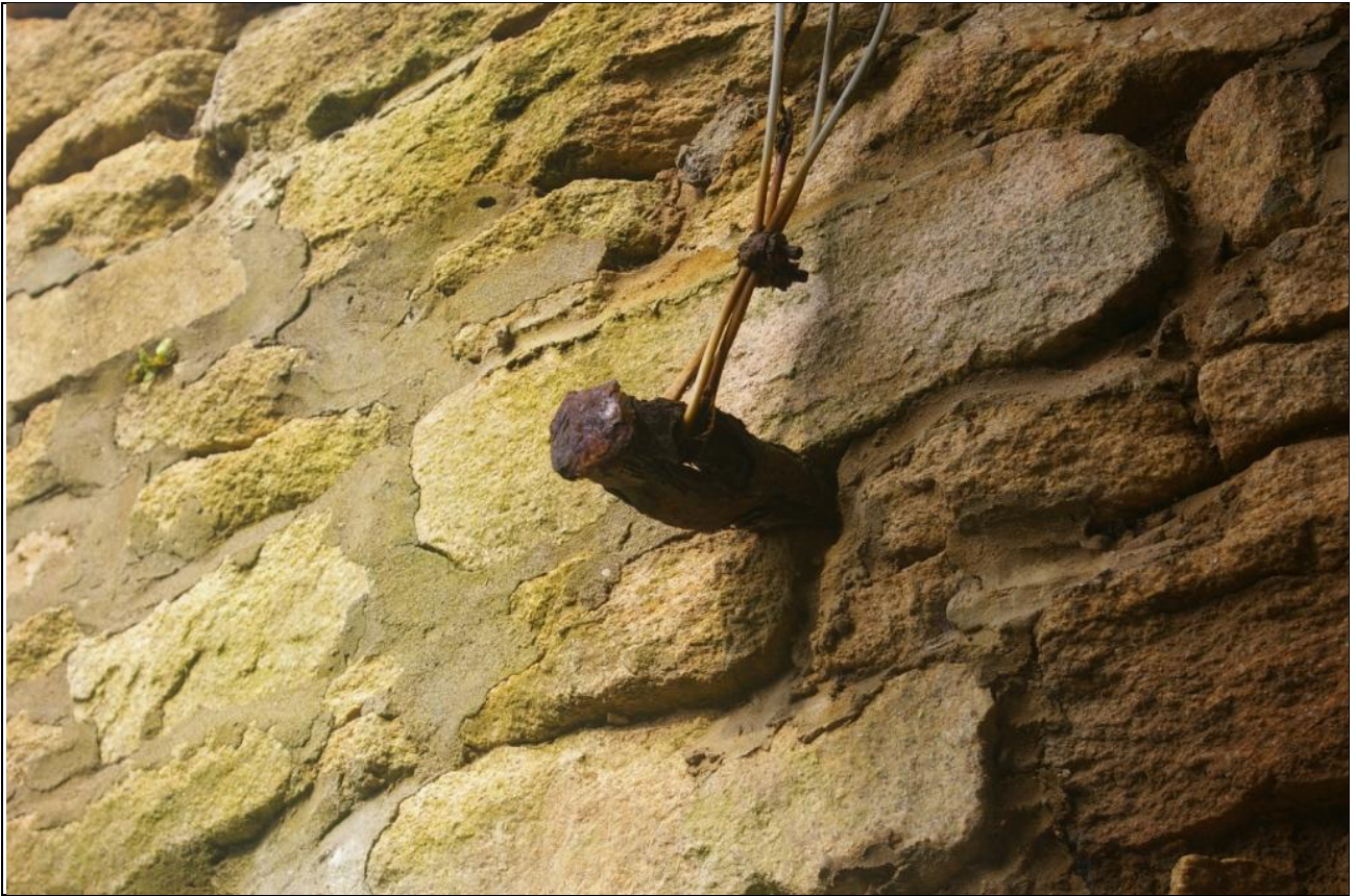
SHOT OF ONE OF THE MINERS METAL HAMMERS SET INTO THE WALL, WRAPPED WITH WIRE TO HOLD ON THE ROOF (NO SCALE).
