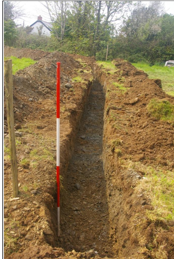
THE EASTERN RUN OF THE SERVICES TRENCH, FROM THE NORTHERN BOUNDARY TO THE BUILDING TRENCH; VIEWED FROM THE SOUTH-EAST (2M SCALE).
