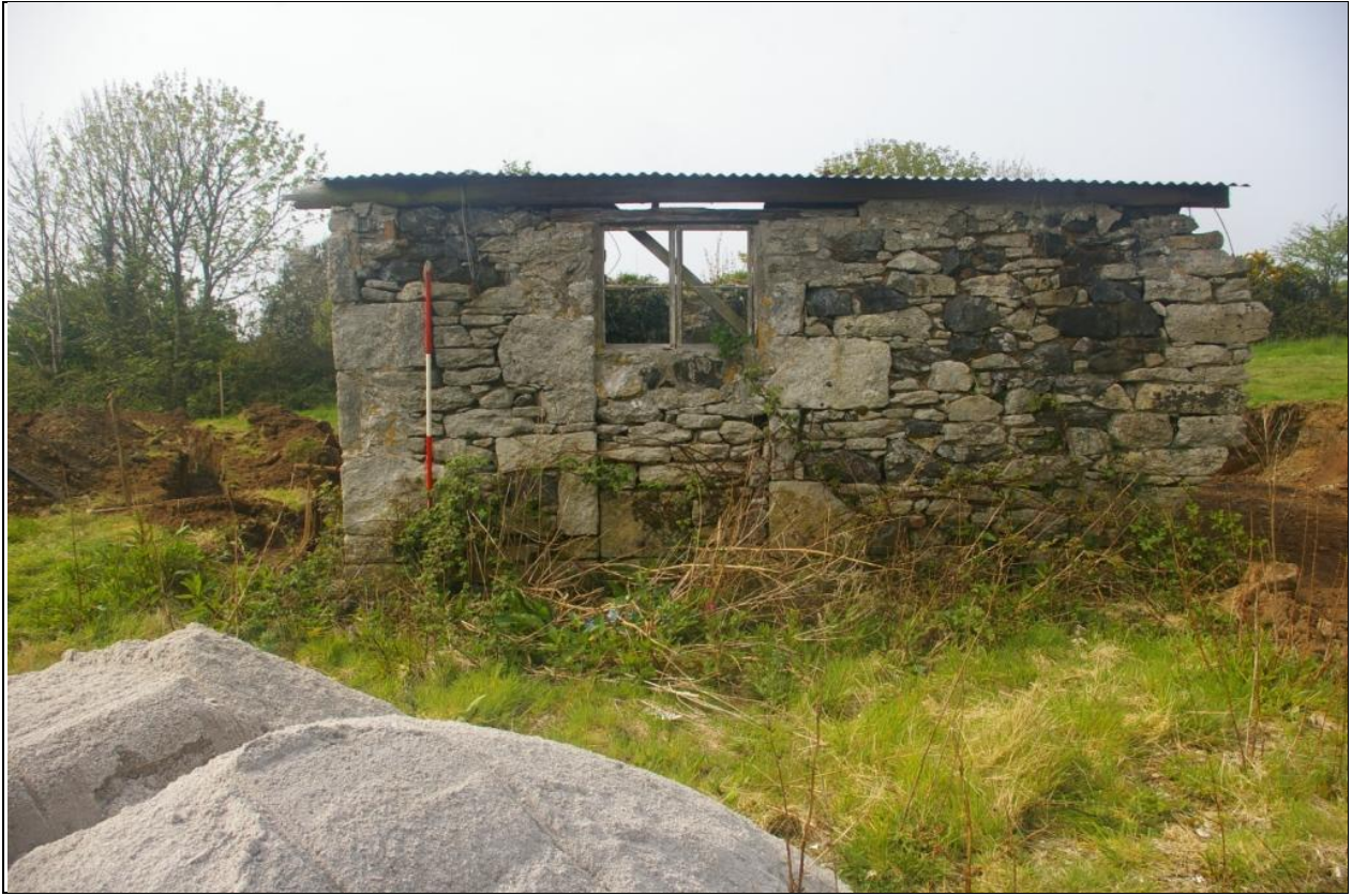
THE SOUTH FACING ELEVATION VIEWED FROM THE SOUTH (2M SCALE).
