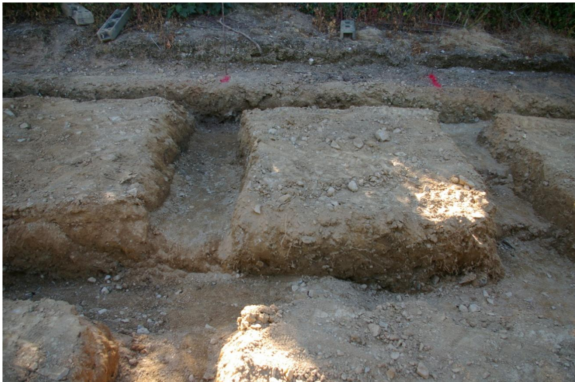
Figure 4: Representative section of building footings, from the east (no scale).
