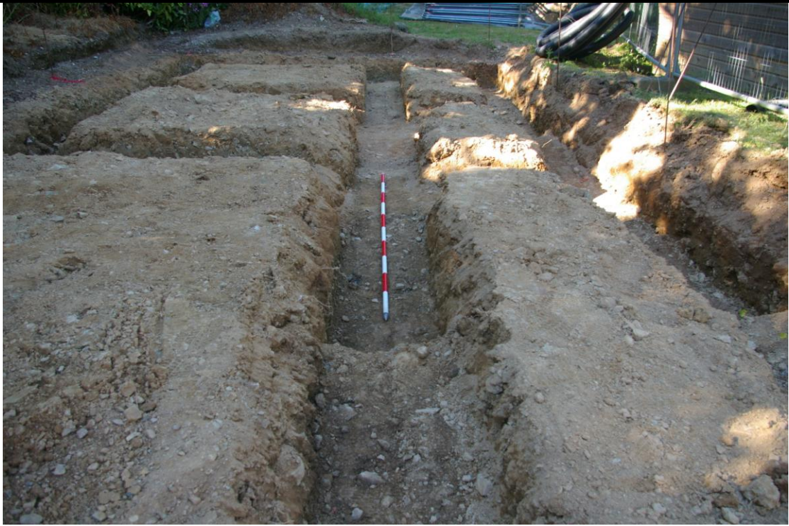
Figure 3: Excavated area for Tractor Store, from the south (scale: 2m)
