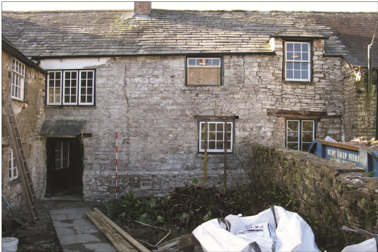
Figure 4 Photograph of the north east elevation
