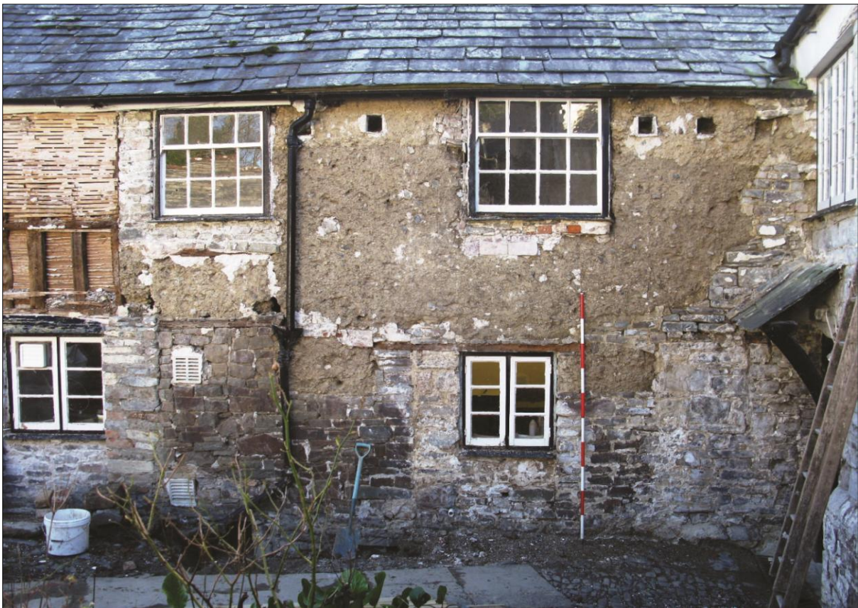
Figure 6 Photograph of north west elevation
