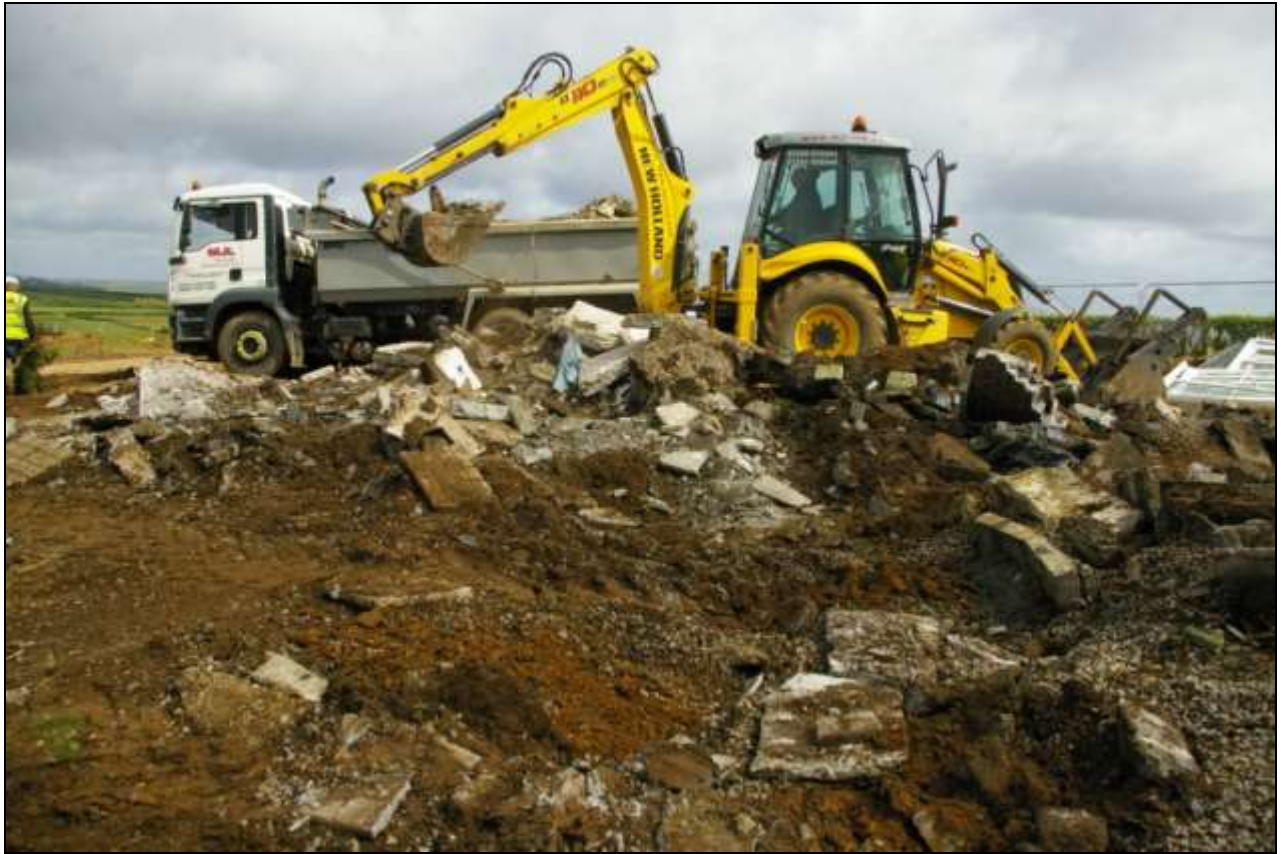
Remains of the bungalow during grubbing up, viewed from the south-west.
