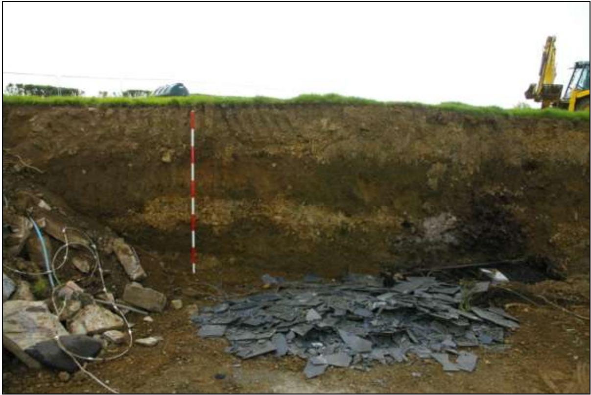
Detail showing the terracing to the rear of the demolished agricultural buildings, viewed from the north (2m scale).
