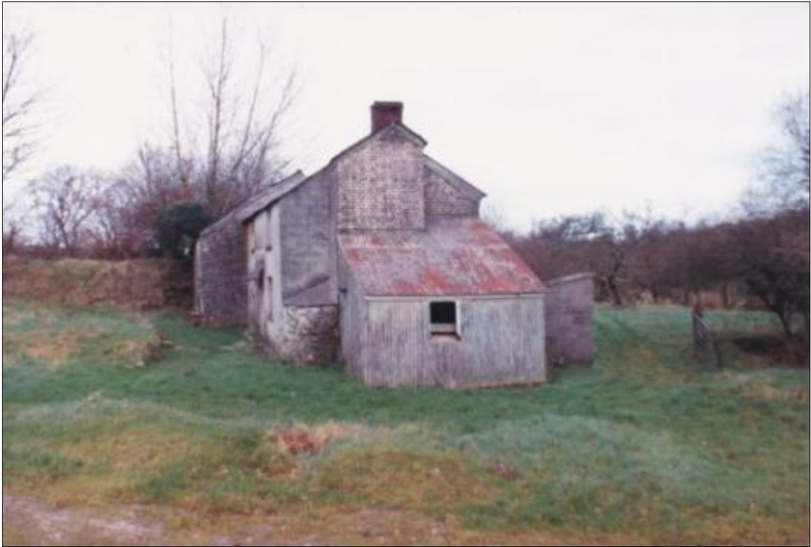
Figure 10: South-east gable elevation of the Cottage in 1988.
