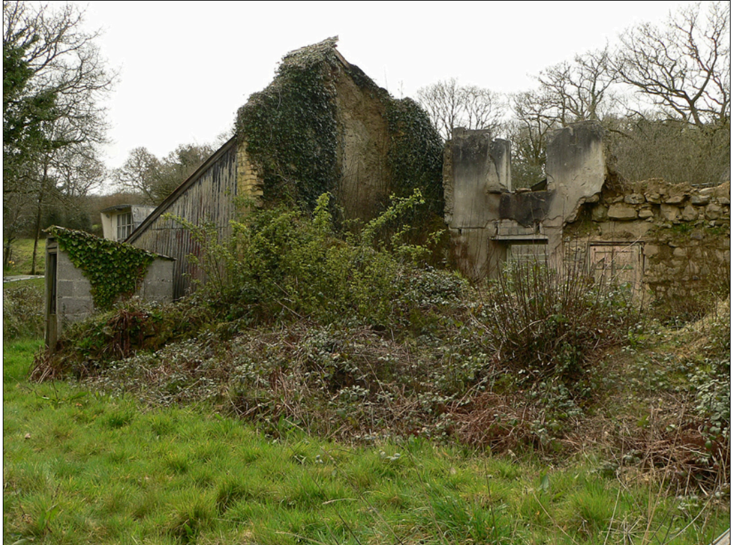
The collapsed north-east (rear) wall of the Cottage.
