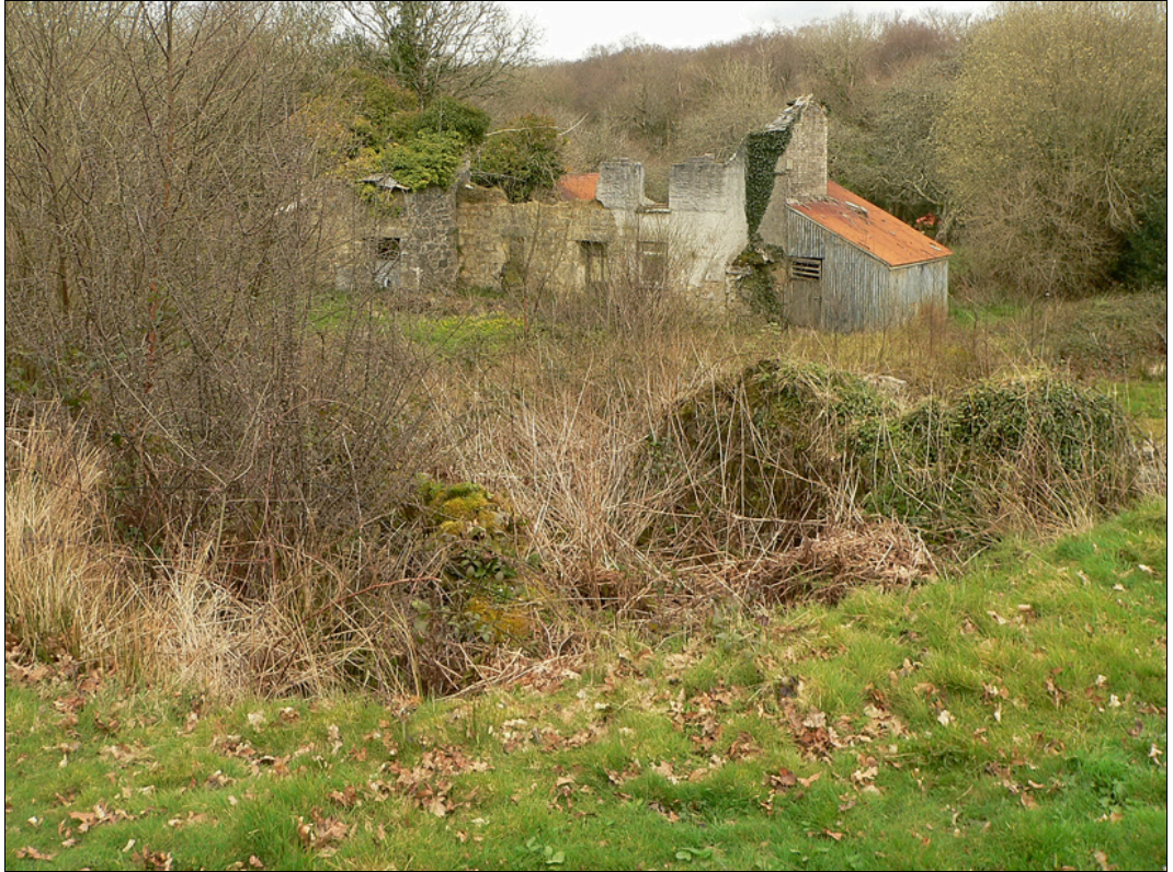
One of the collapsed outbuildings, from the south.
