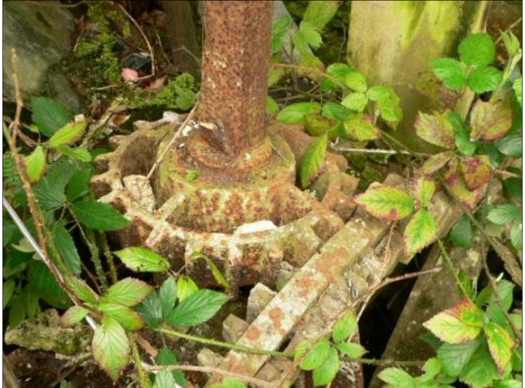
Drive to upstream millstones.
