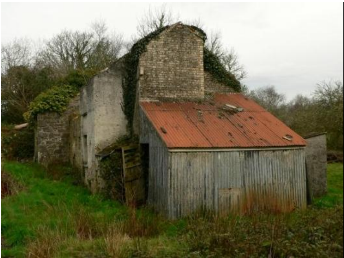
Figure 11: South-east gable elevation of the Cottage in 2014.
