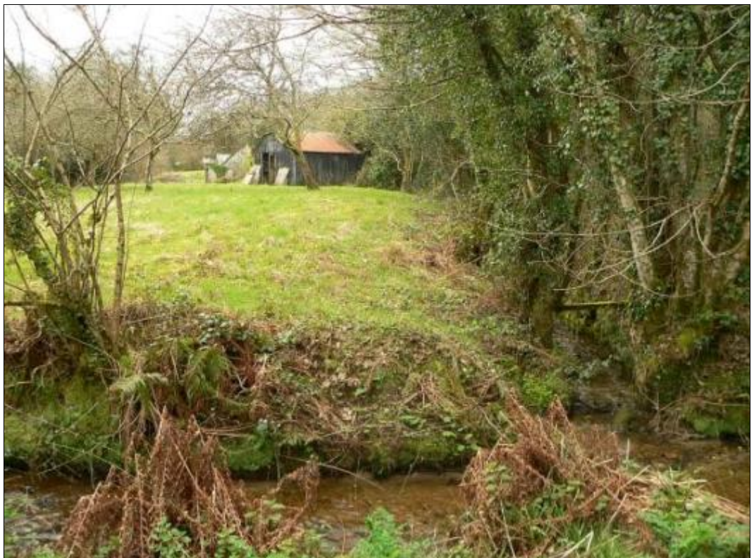
Tailrace (right) rejoining stream below mill
