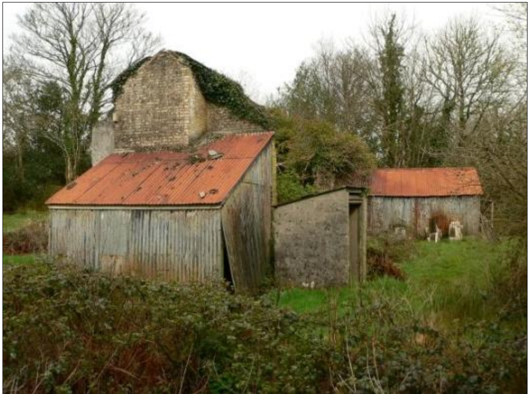
View from south-east, showing the lean-to shed and free-standing concrete block privy.
