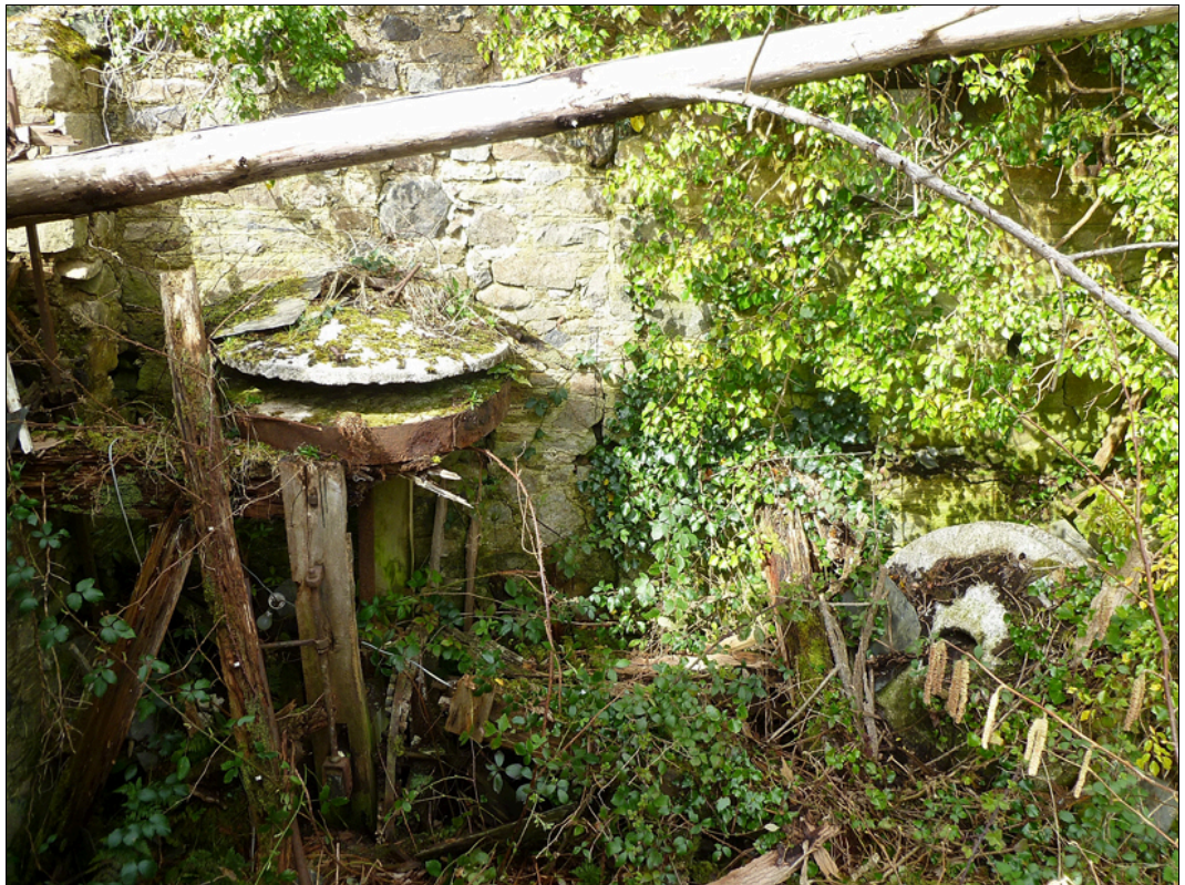
Remains of the hurst, showing the collapsed downstream millstones.
