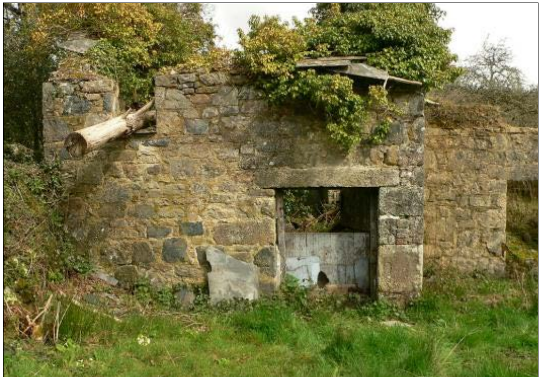
South-west elevation of Mill in 2014.
