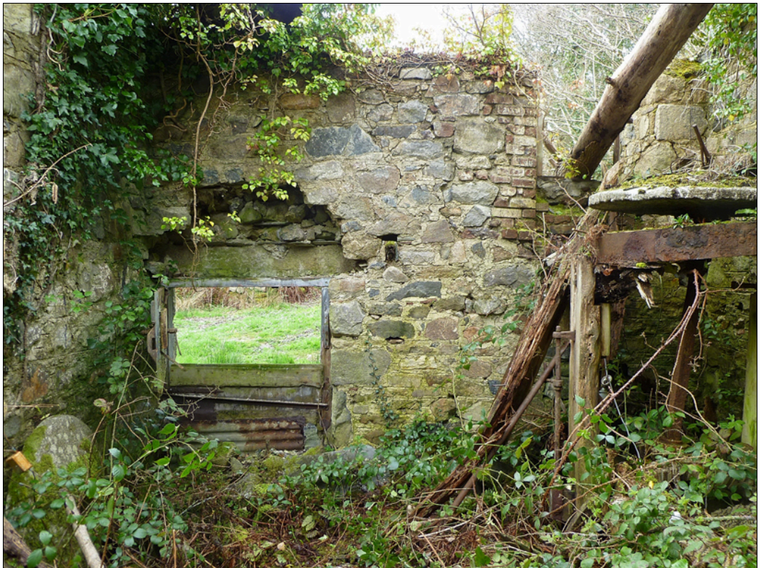
Interior face of the north-west elevation of the Mill.
