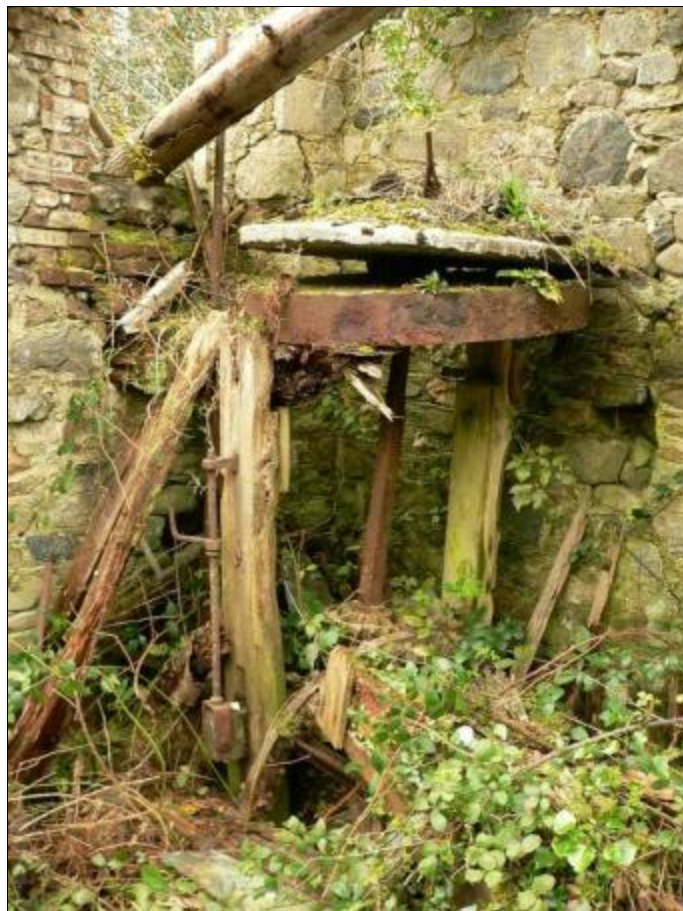
Figure 18: Remains of the hurst and upstream millstones.
