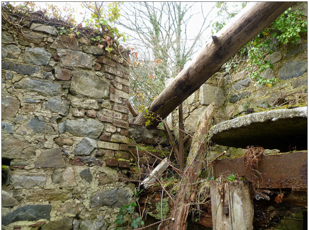
As above, showing the brick reveals to the first-floor window.
