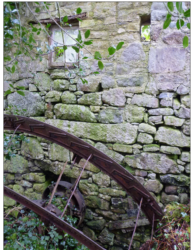
[left] The wheelpit, from above. [right] The wheel in relation to the window and lever slot used to control the flow of water over the wheel.
