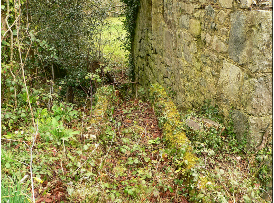
Detail of the granite trough leading to the (vanished) timber launder.
