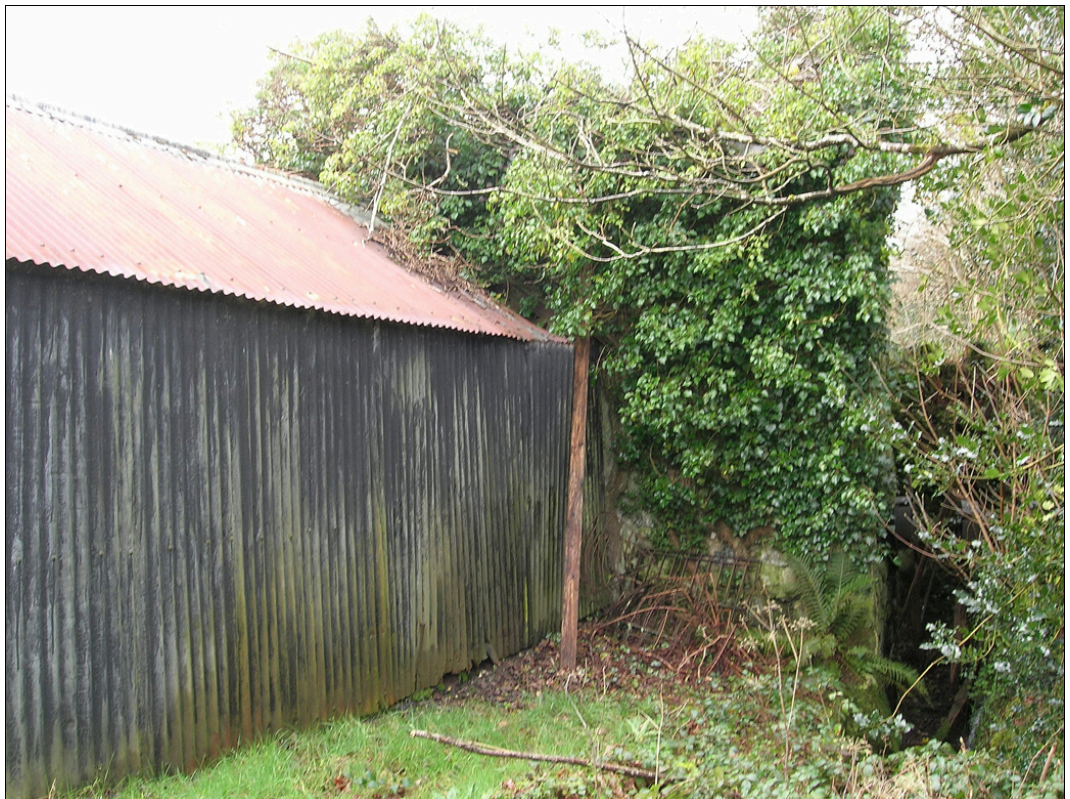
The north-east (rear) elevation of the Mill.
