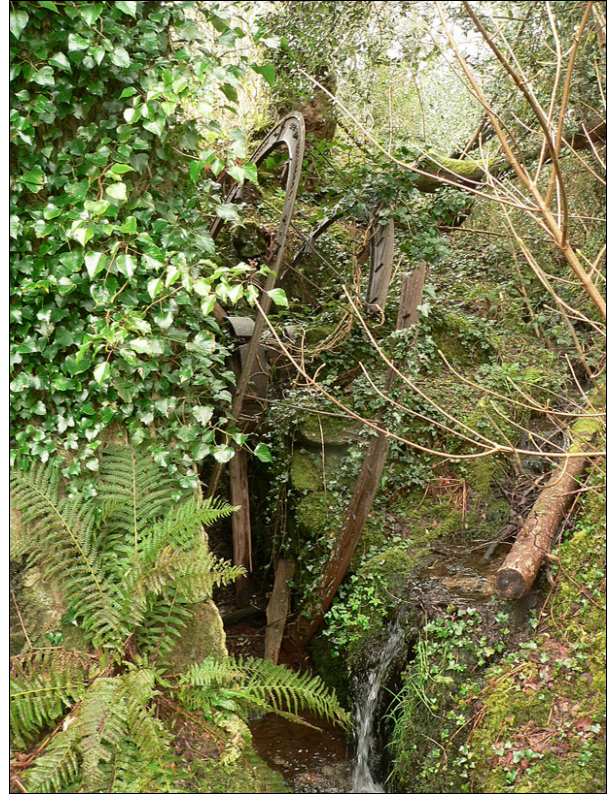
The waterwheel and wheelpit, viewed from the tailrace.
