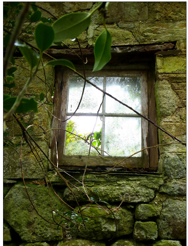
The four-light window in the gable wall of the Mill.
