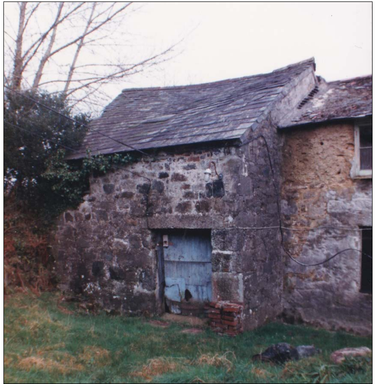
South-west elevation of the Mill in 1988.
