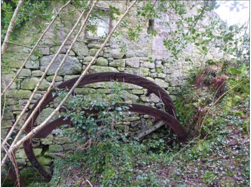
North-west gable end of Mill, wheelpit and waterwheel.
