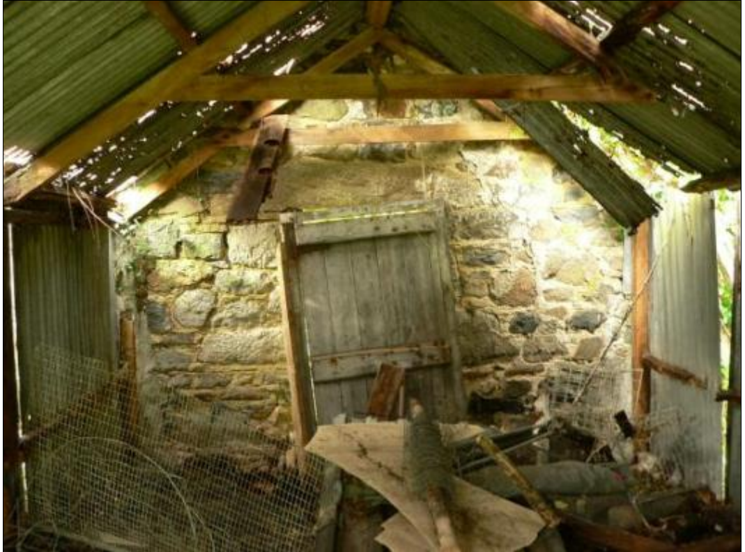
North-east doorway into Mill, from inside the adjoining corrugated iron shed.
