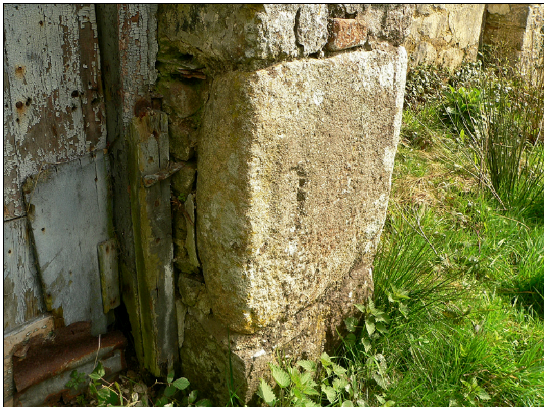
Detail of the possible re-used millstone used as a quoin.
