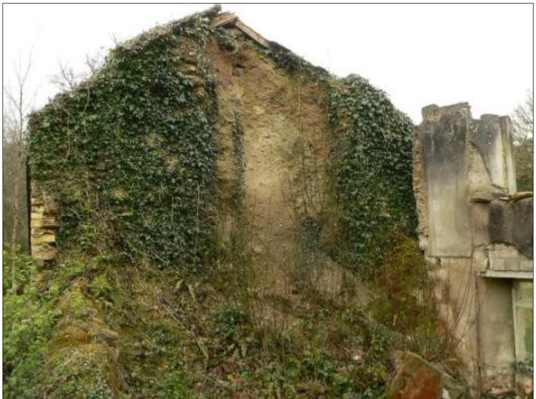
South-eastern gable end of the Cottage, interior view.
