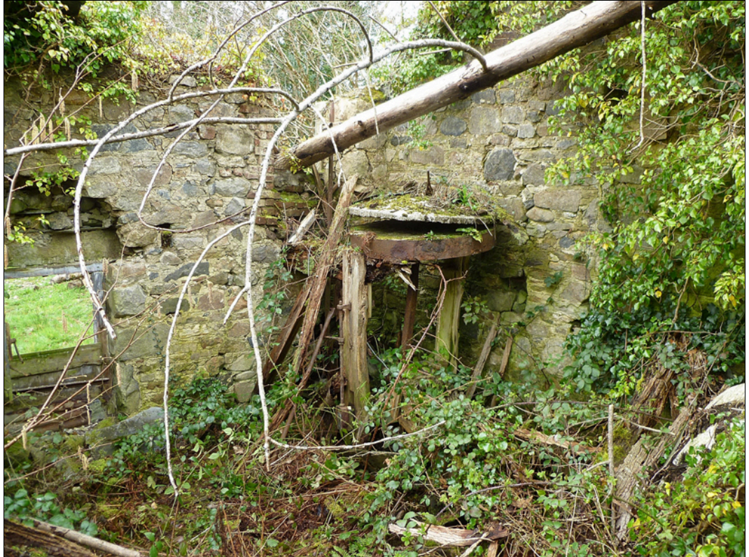
As above, showing the in situ upstream millstones.
