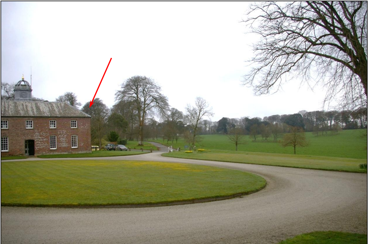
Important designed view from the East Pavilion (formerly the coach house) up the main driveway; the location of the proposed biomass boiler building is indicated. Viewed from the south-east.
