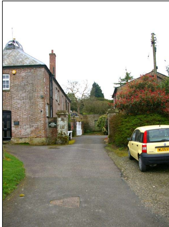
View up the narrow entrance into the service courtyard to the west of the West Pavilion, showing local blocking from the West Pavilion, the stables pavilion building, garden wall and service buildings within the courtyard; from the north.
