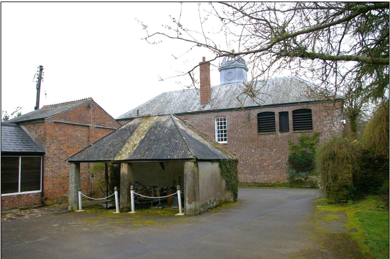
View of the west elevation of the West Pavilion where it overlooks the former stables courtyard; from the south-west.
