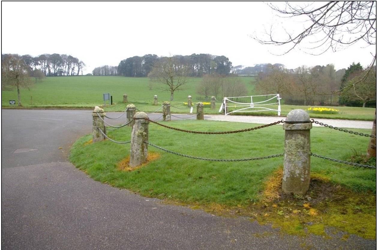
View down and across the bollards and gate, as they frame the gravel driveway; from the south.
