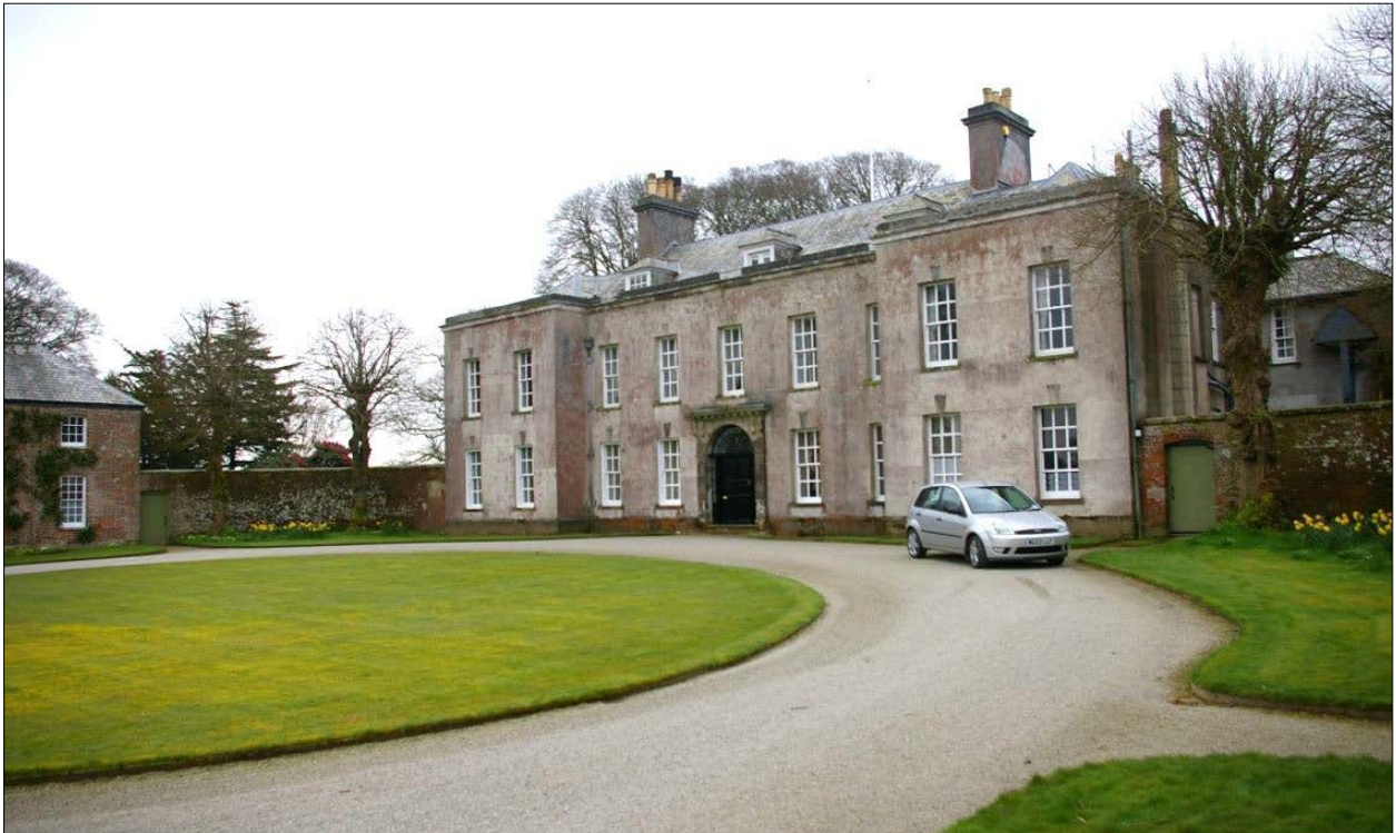
View of the Trewithen House, showing the north elevation, which faces the courtyard; from the north-west.
