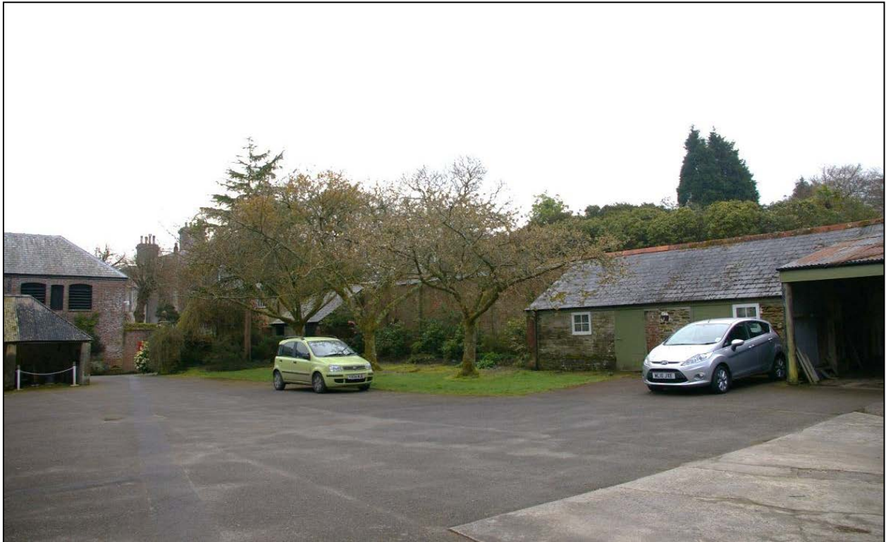
View across the former stables courtyard to the northern kitchen garden walls, abutted with small outhouses and partly shielded by some mature fruit trees; from the north-west.
