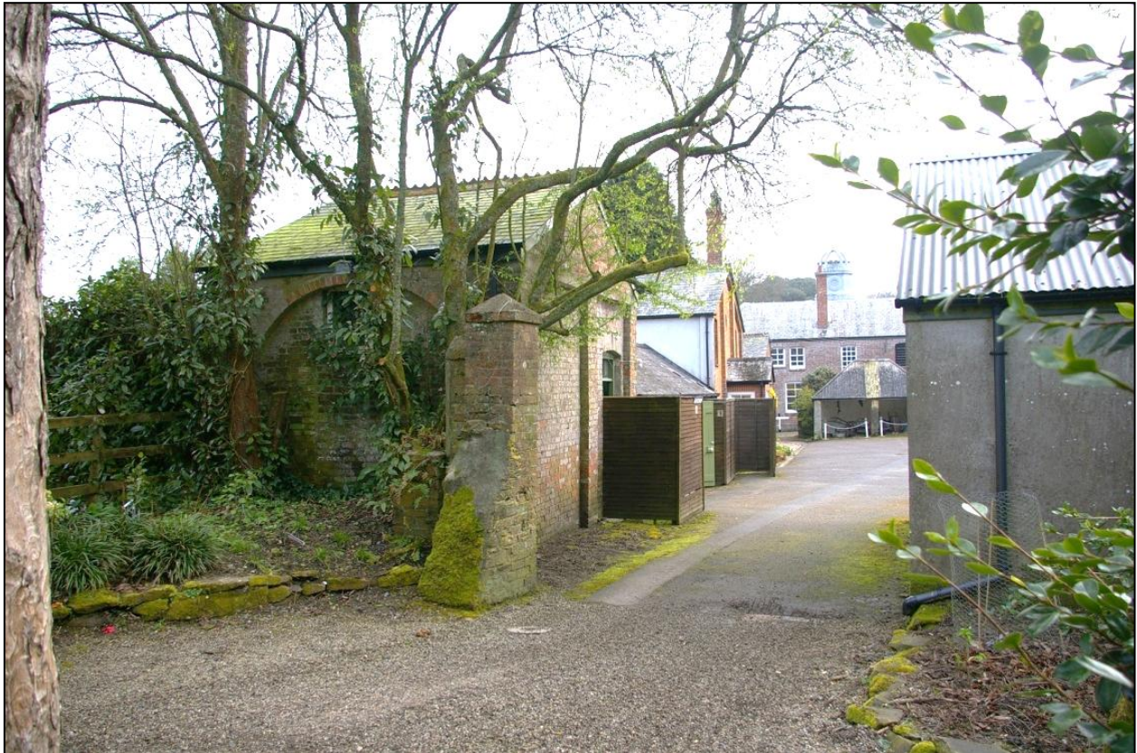
The corner where the trenching will turn and run east into the former stables courtyard; from the south-west.
