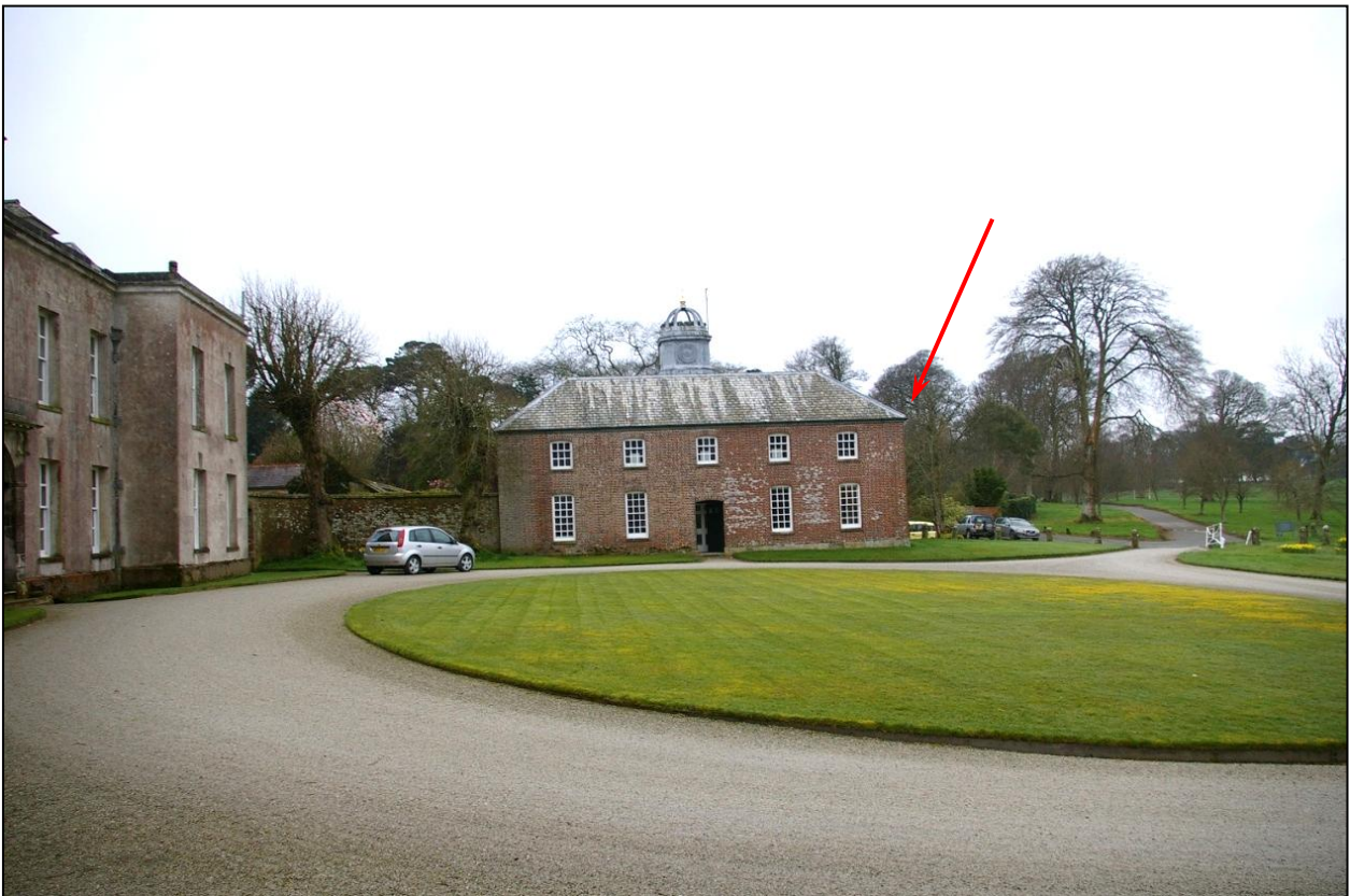
Important designed view from the East Pavilion across the courtyard to the West Pavilion. The location of the proposed biomass boiler building is indicated. Viewed from the east.
