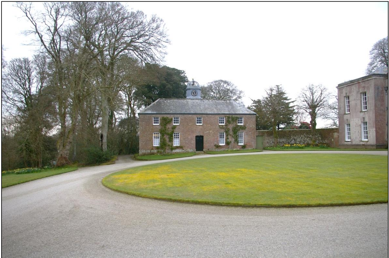
View back across the formal courtyard to the East Pavilion, with its clock tower and symmetrical western facade; from the north-west.
