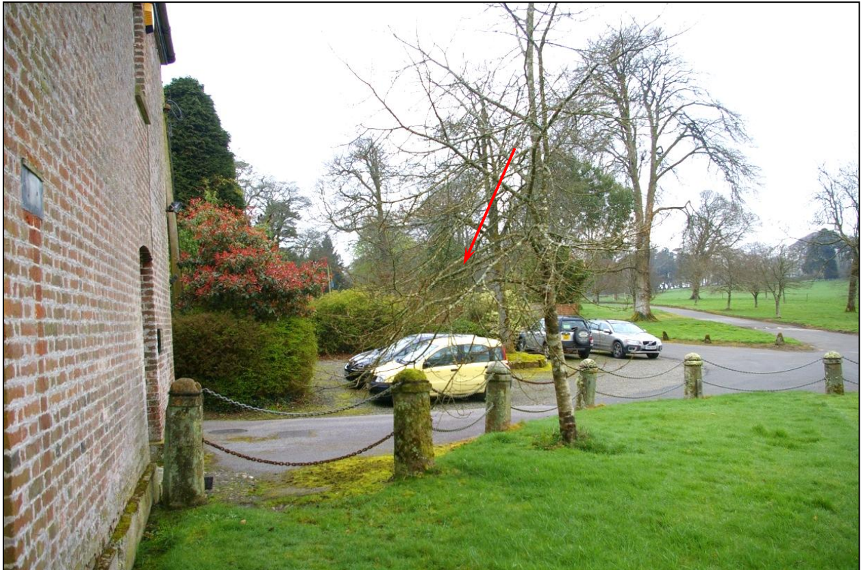
View showing the local blocking at the southern end of the bollard and chain-link gateway; from the east.
