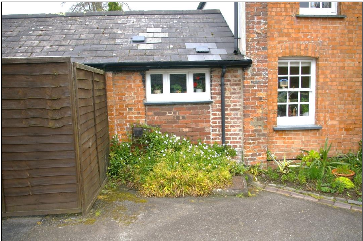
The blocked opening where the trenching will enter the building to provide heating to Garden Cottage; there is a manhole cover, indicating the present of extant services. Viewed from the south.
