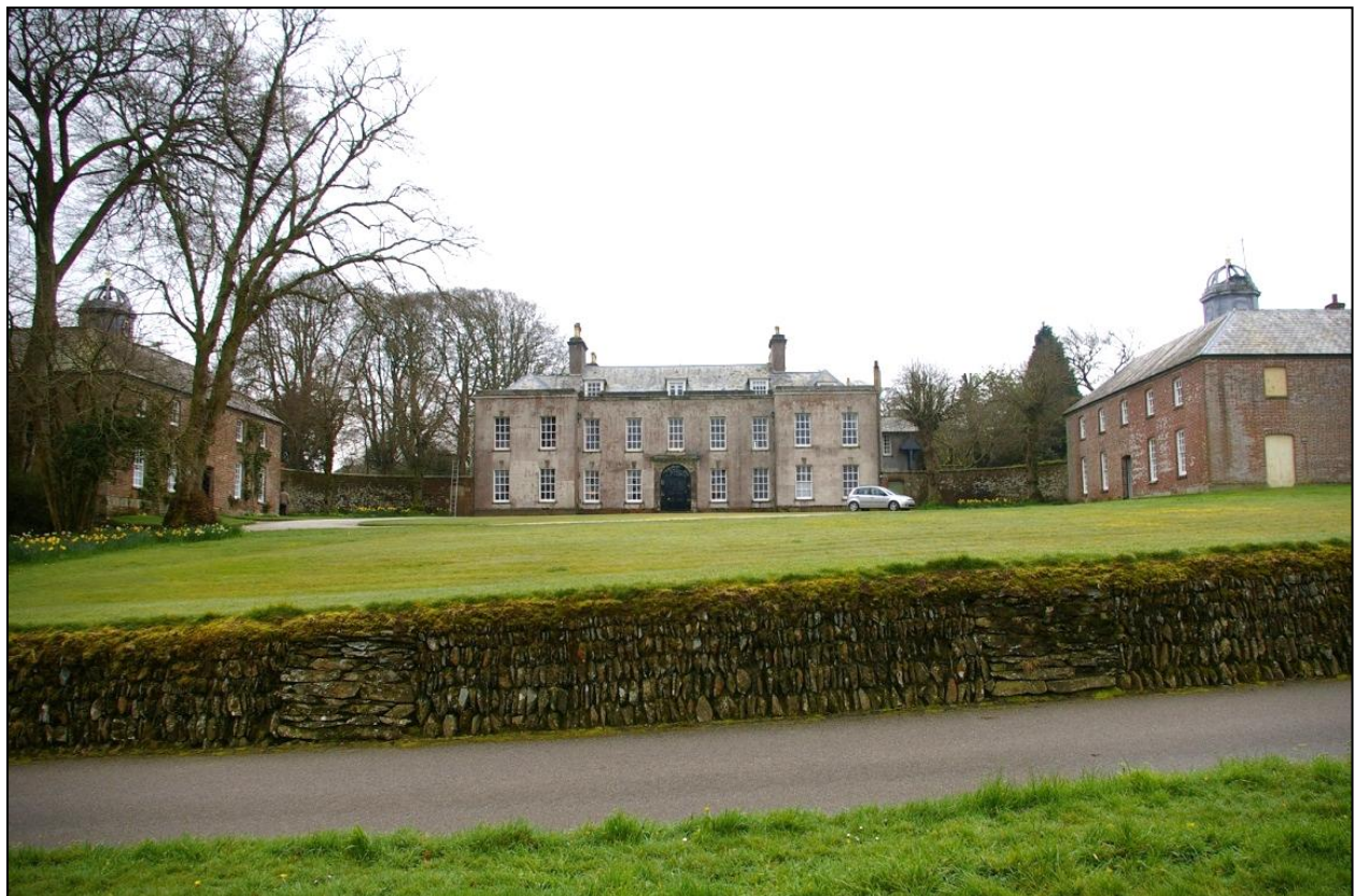
View of the ha-ha/retaining wall of the raised lawn in front of the courtyard, where it drops to the parkland. This photograph shows the layout and key relationships between the House and its Pavilions; from the north.
