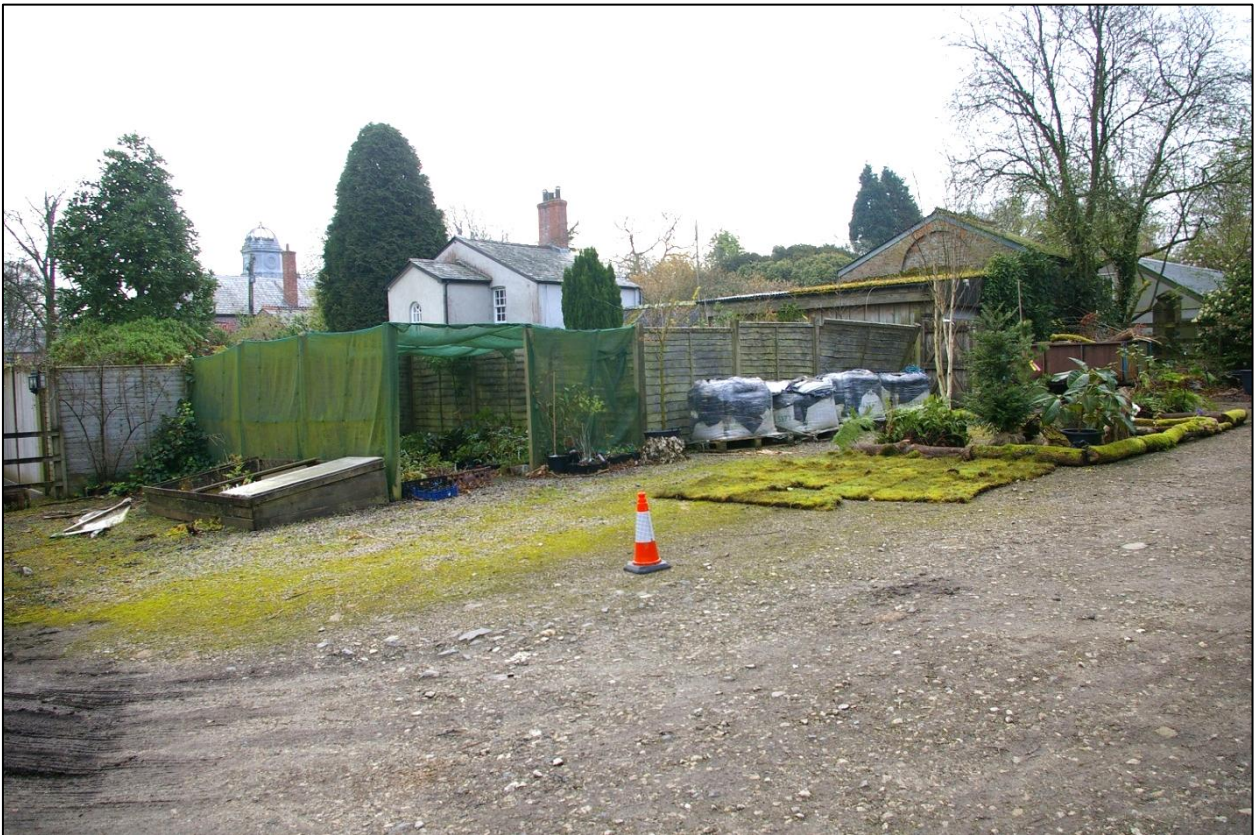
View of the site of the proposed biomass boiler building, showing the current temporary structures and fenced enclosure, with Garden Cottage and former stables pavilions beyond; from the north-west.
