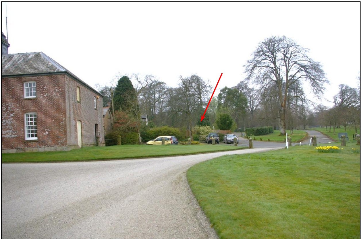
General view back across the bollards from the northern end of the formal courtyard, with the site of the proposed biomass boiler indicated beyond; from the east.
