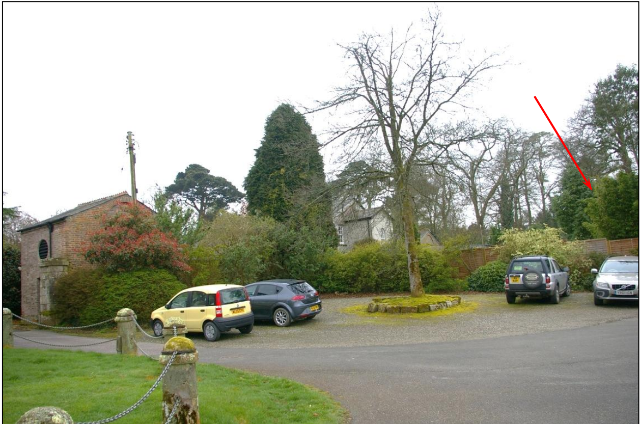
View from the bollards to Garden Cottage and the parking area which has been created for the estate office adjacent to the timber fencing; the location of the proposed biomass boiler building is indicated. Viewed from the north-east.
