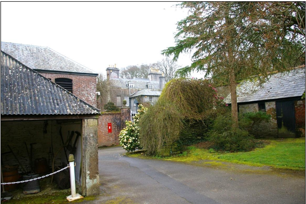
View of the eastern end of the kitchen garden walls where they exit the courtyard and run up to the service courtyard and service wing of the House; from the north-west.
