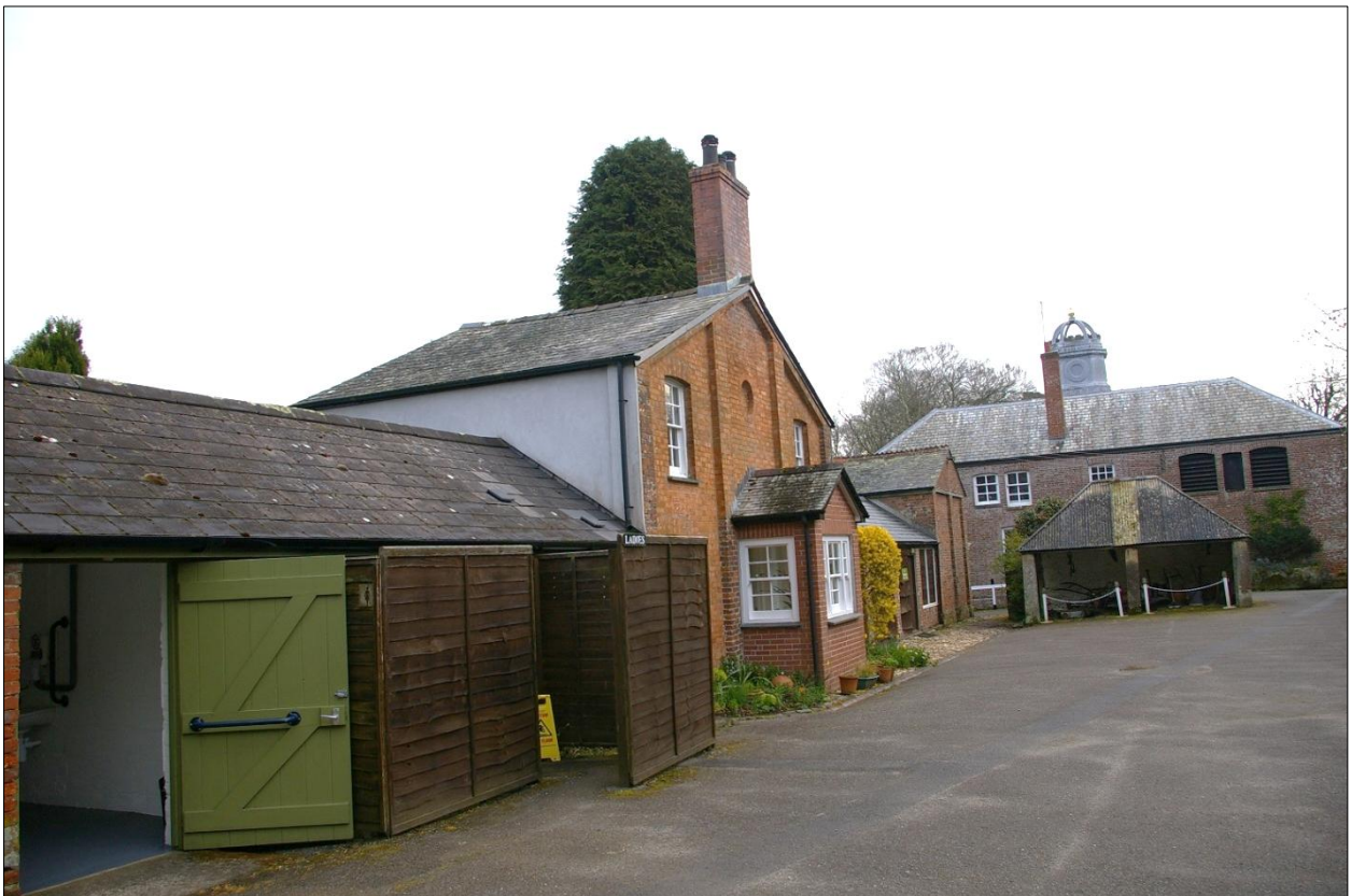
View along the south front of the former stables pavilion building, with the West Pavilion to the east and the small open-fronted store between; from the south-west.
