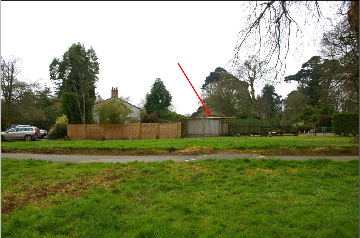
View south from across the main drive to the site of the proposed biomass boiler building, showing Garden Cottage and the roofs of the former stables pavilion building rising above the garden fencing; from the north.
