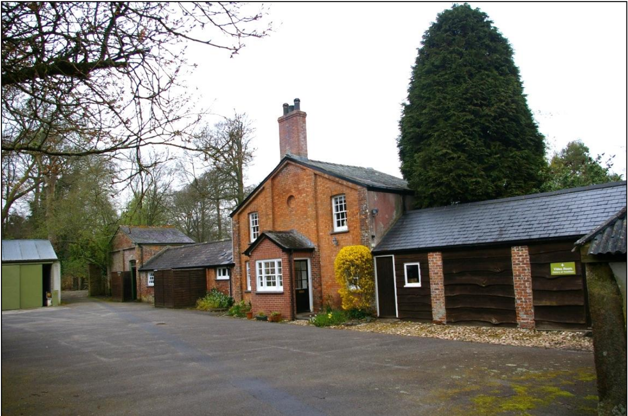
View across the courtyard from the eastern end of the kitchen garden walls, showing the local blocking between them and the proposed biomass boiler building; from the south-east.
