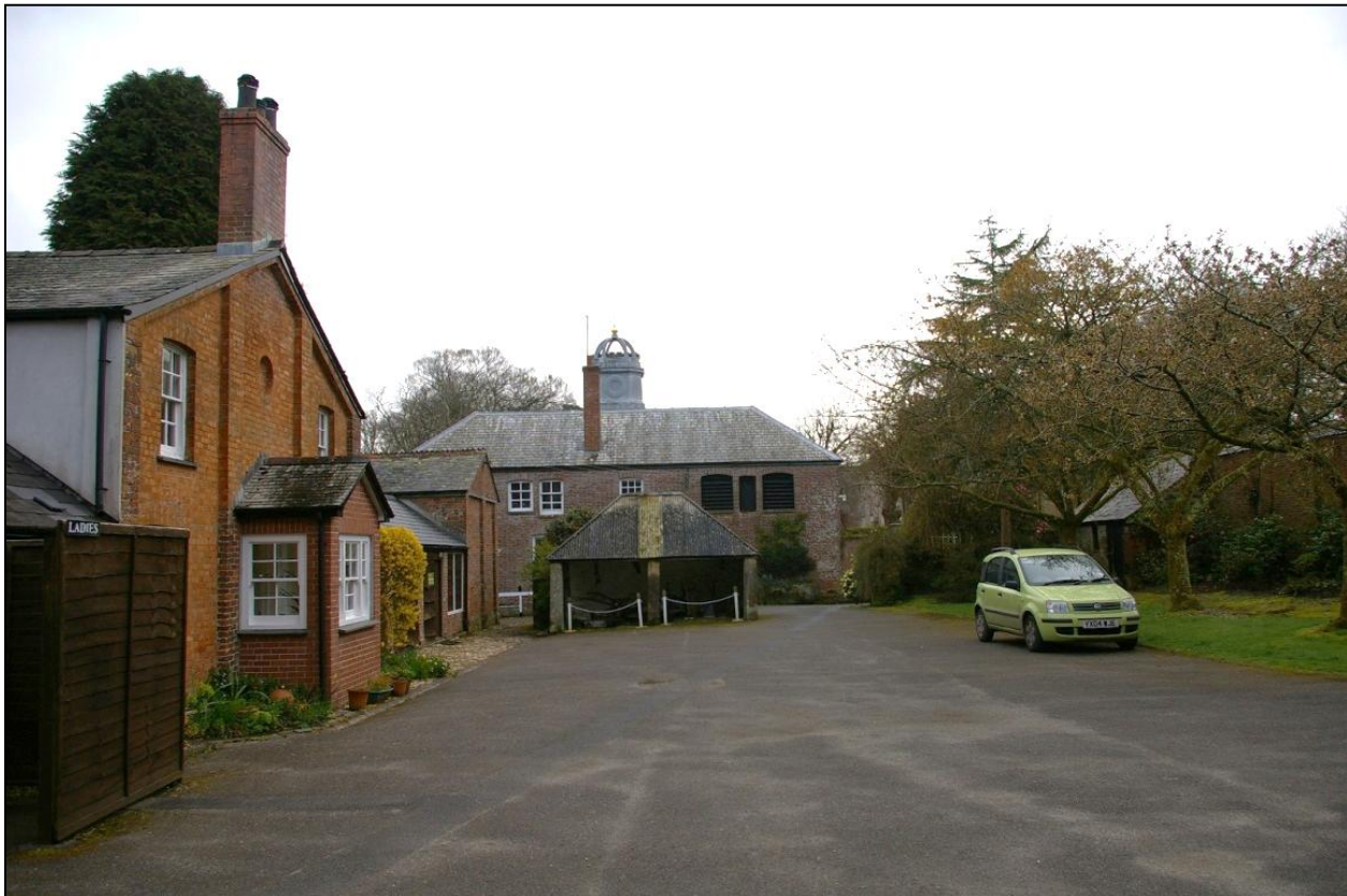
View across the same courtyard, showing the West Pavilion to the east, the former stables (now Garden Cottage) to the north and the kitchen garden walls to the south; from the west.
