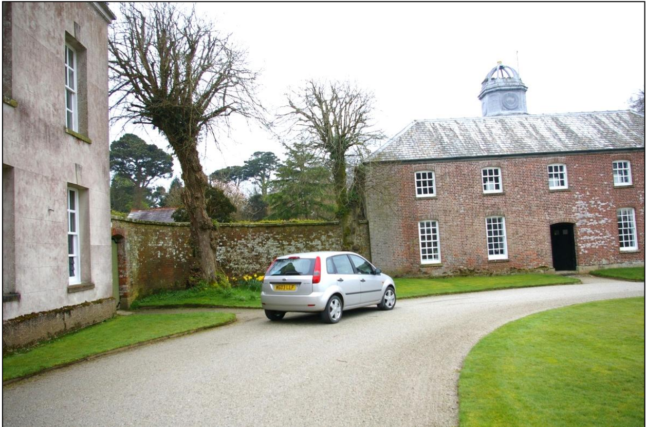
View of the west flanking wall which links the House and West Pavilion. This demonstrates local blocking at ground floor level, with no views to the service courtyards beyond. Viewed from the east.
