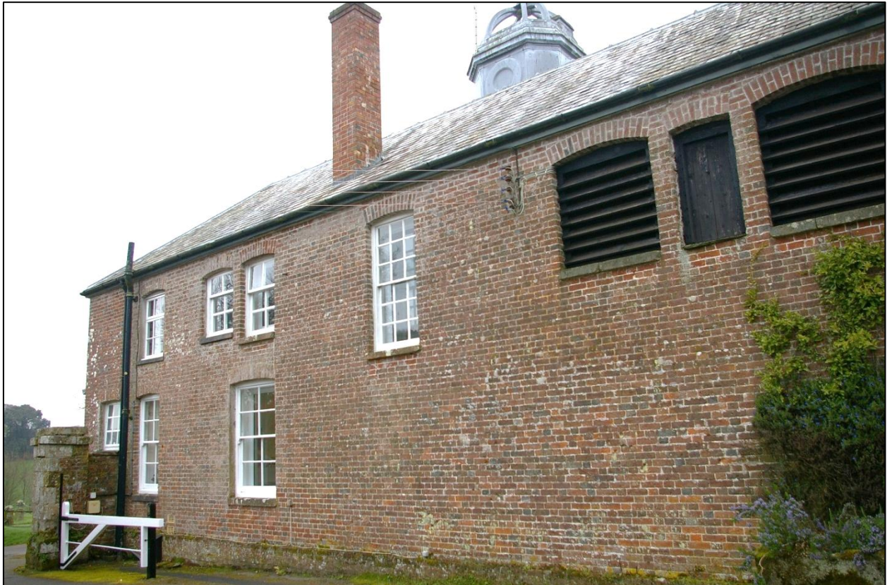
The northern end of the west elevation of the West Pavilion, showing the first-floor windows that may enjoy some very limited views past the former stables pavilion to the proposed biomass boiler building; from the south-west.
