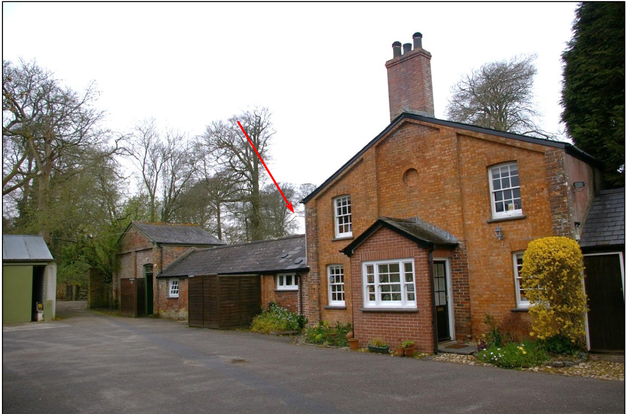
View of Garden Cottage and the West Pavilion, showing where the proposed biomass boiler building may just be visible over the central single-storey section of the building. This photograph also shows the extensive rebuilding of Garden Cottage, with different periods of brickwork; from the south-east.
