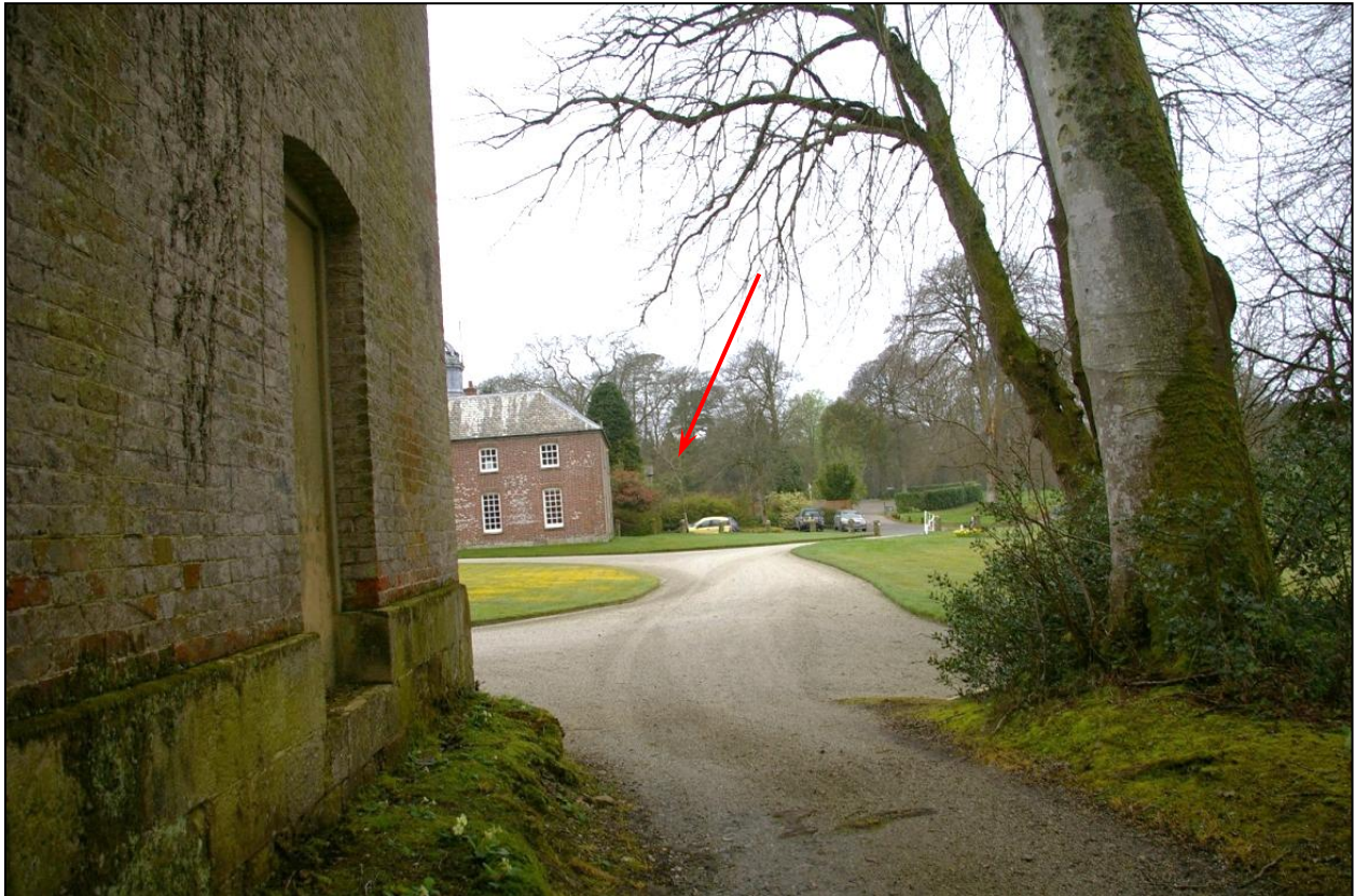
View past the north wall of the East Pavilion, across to the entrance to the courtyard, and towards the location of the proposed biomass boiler building beyond; from the east.
