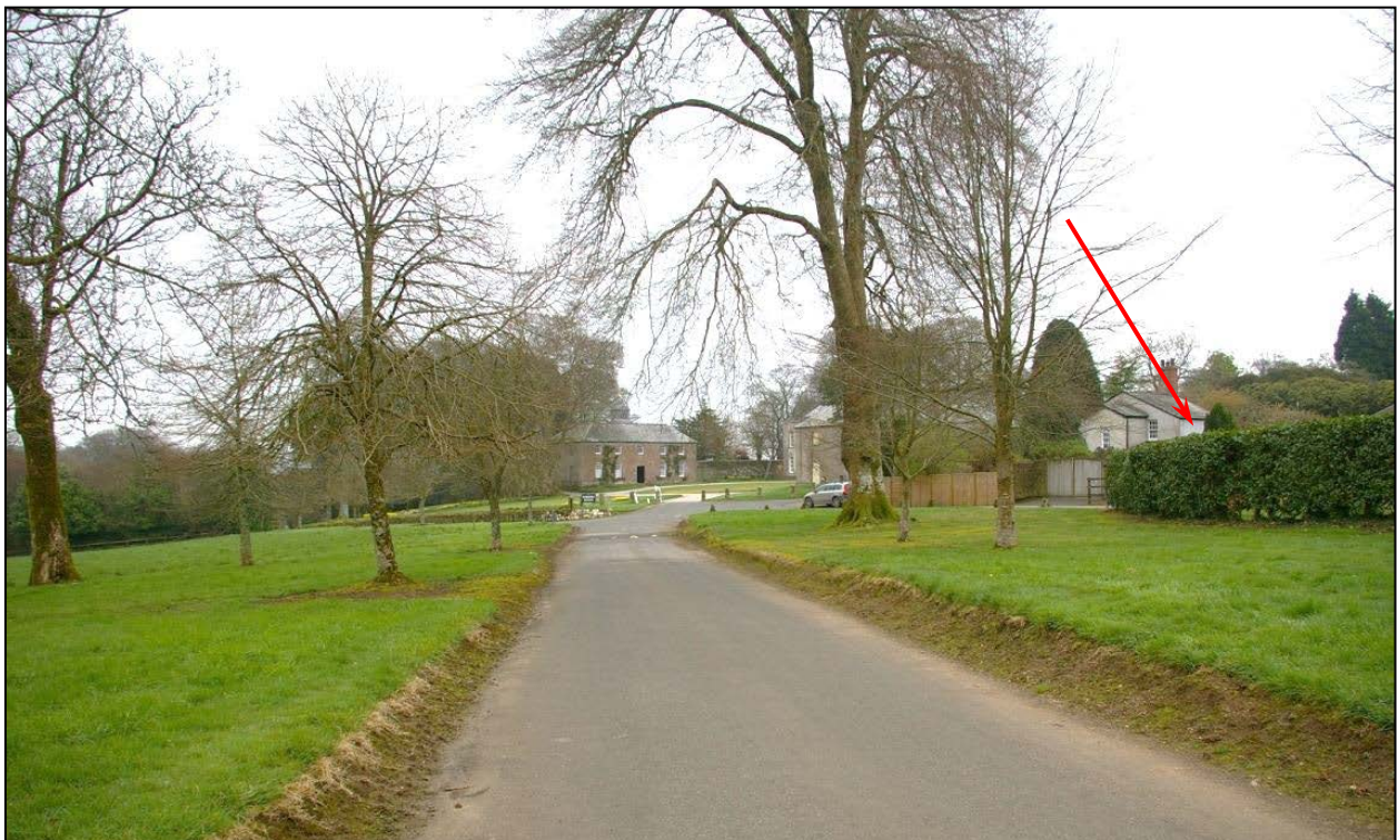
View down the main drive towards the bollards as they frame the entrance into the formal courtyard and visually guide the eye into the courtyard, towards the East Pavilion and the north-east corner of the House; the location of the proposed biomass boiler building is indicated. Viewed from the north-west.
