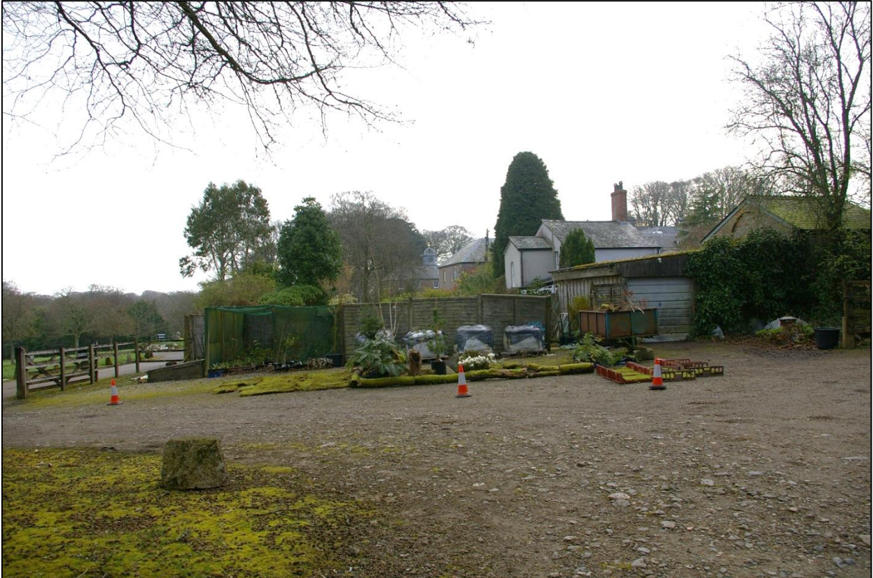
View of the site, showing the slope to the north and the local blocking provided by the enclosed gardens of Garden Cottage. The East and West Pavilions are visible in the background; viewed from the west.
