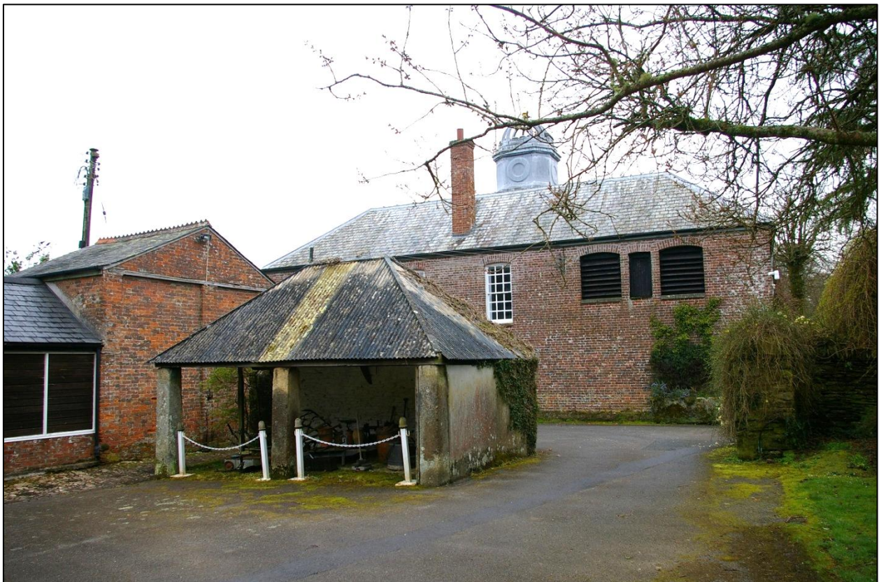
View of the eastern end of the former stables pavilion and the West Pavilion and store, showing the various levels of local blocking between the buildings; from the south-west.
