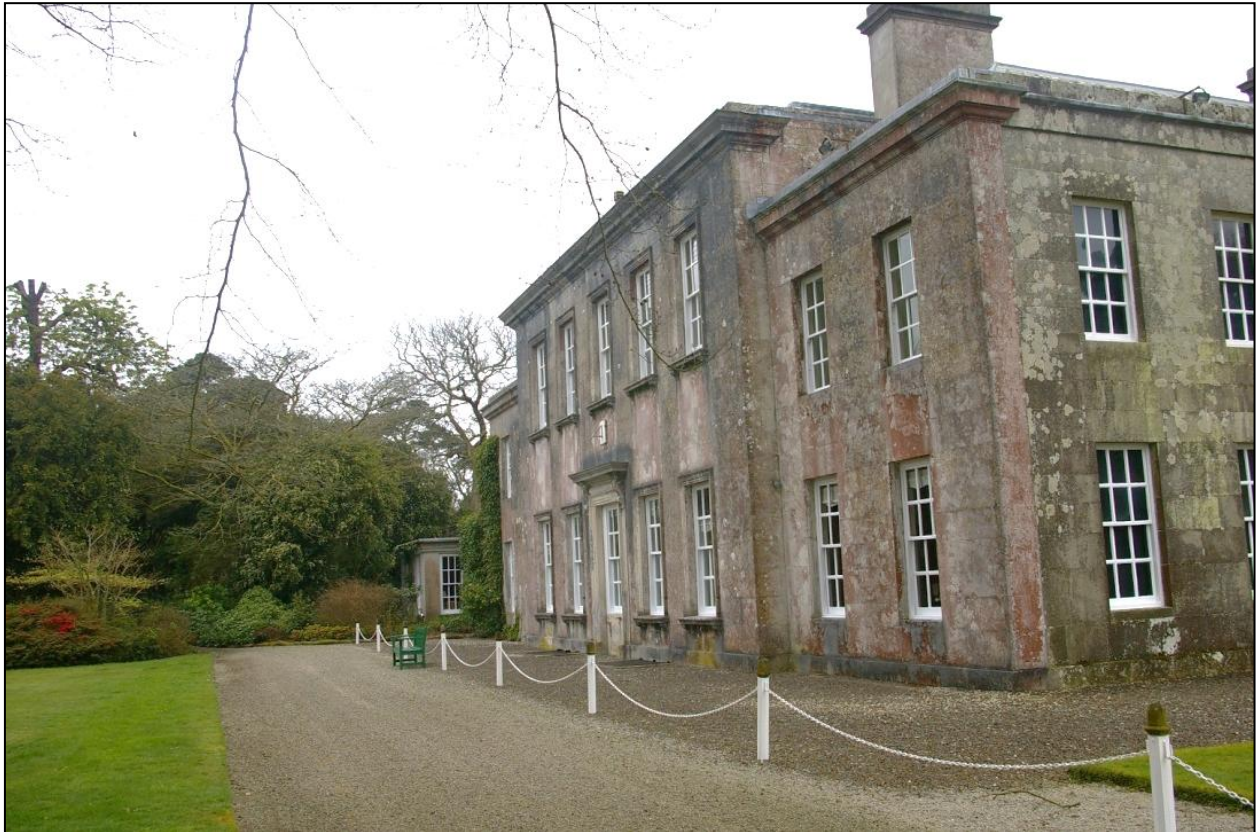
View down the south elevation of the House; from the east.
