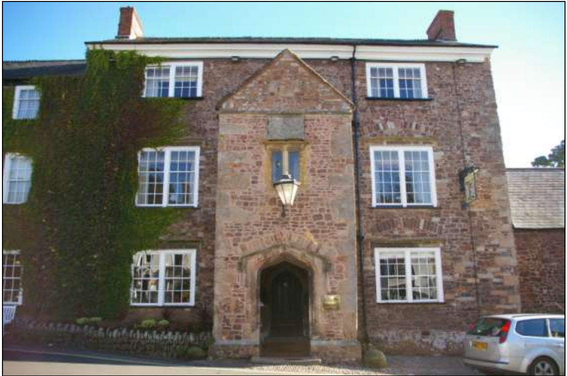
Figure 13: West elevation of main block with projecting porch; from the west.
