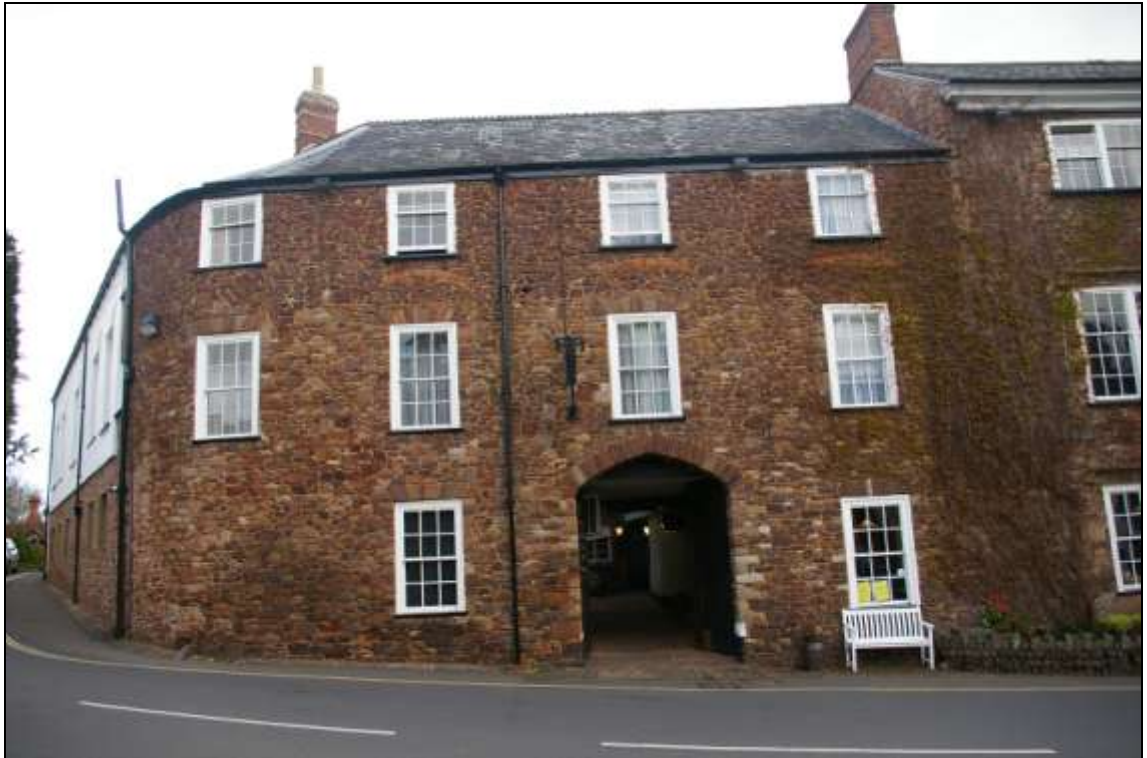
Figure 8: View of the west front of the 18th century or early 19th century section of the buildings to the north, with earlier segmental stone arch over the entrance to the service courtyard; from the west.
