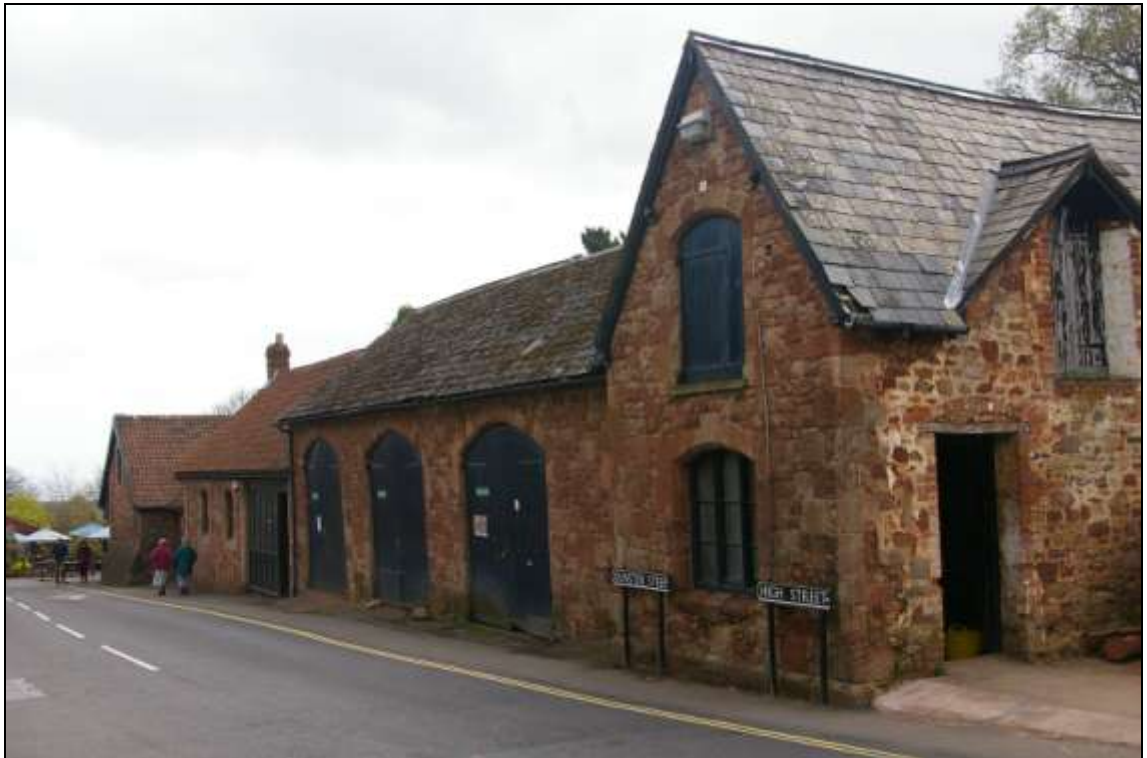
Figure 10: View down the main presentation front of the coach house range as it faces onto Dunster Steep; from the north-west.
