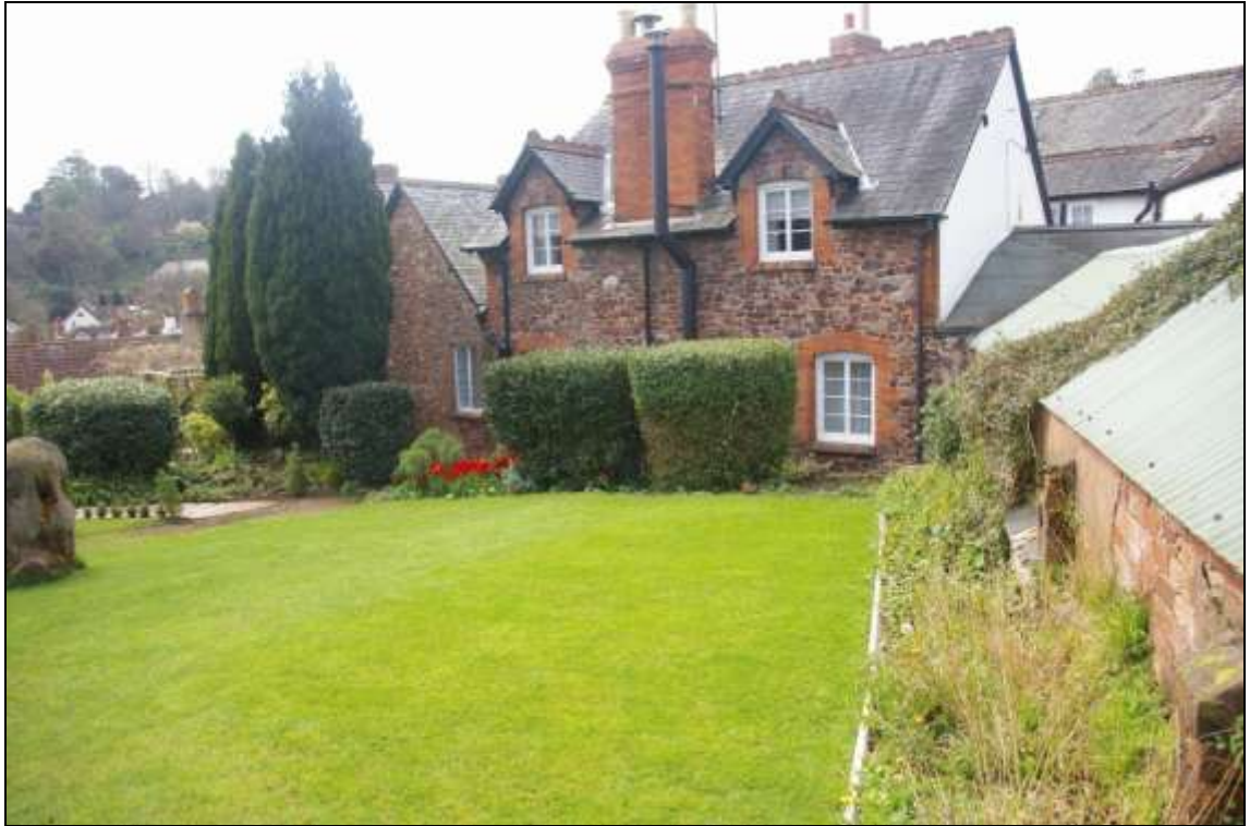
Figure 14: View across the garden showing the area to be disturbed by the service tunnel; from the north-east.
