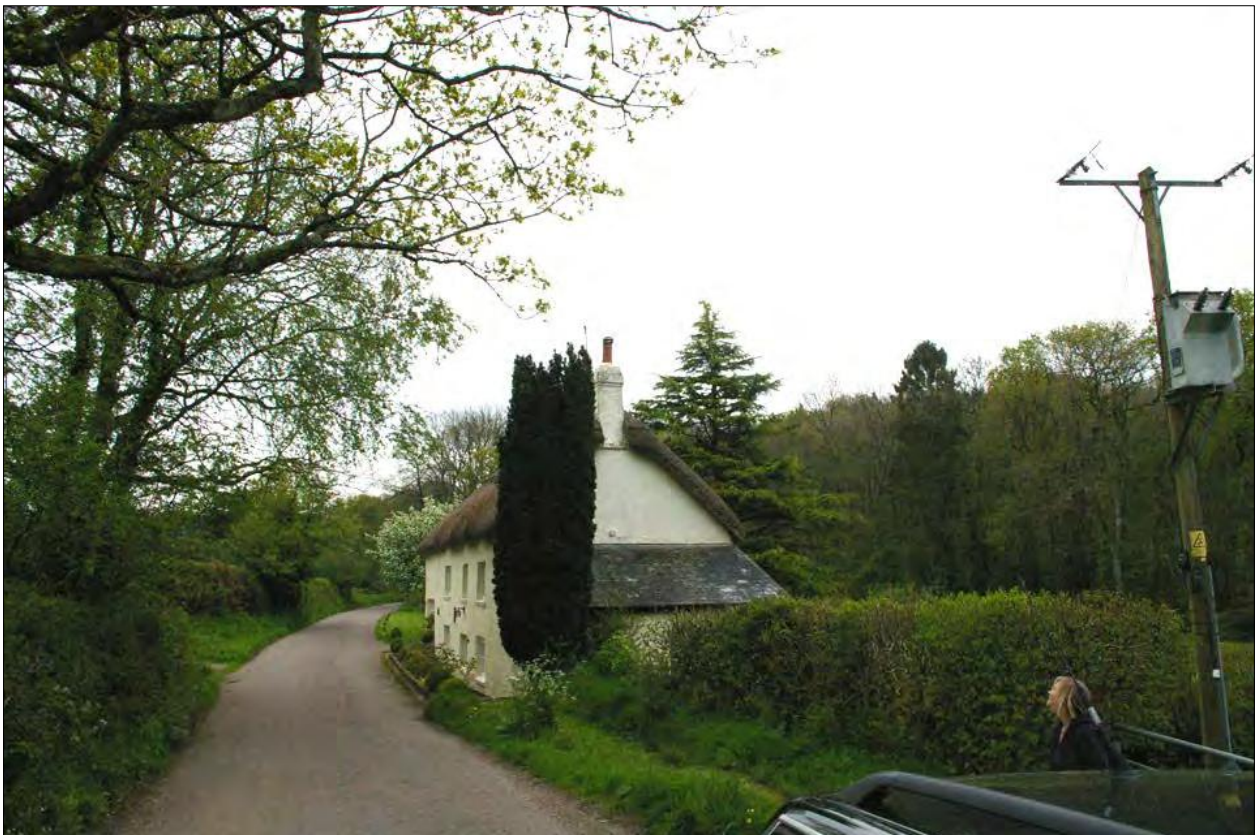
Ham Cottage, viewed from the north-west.
