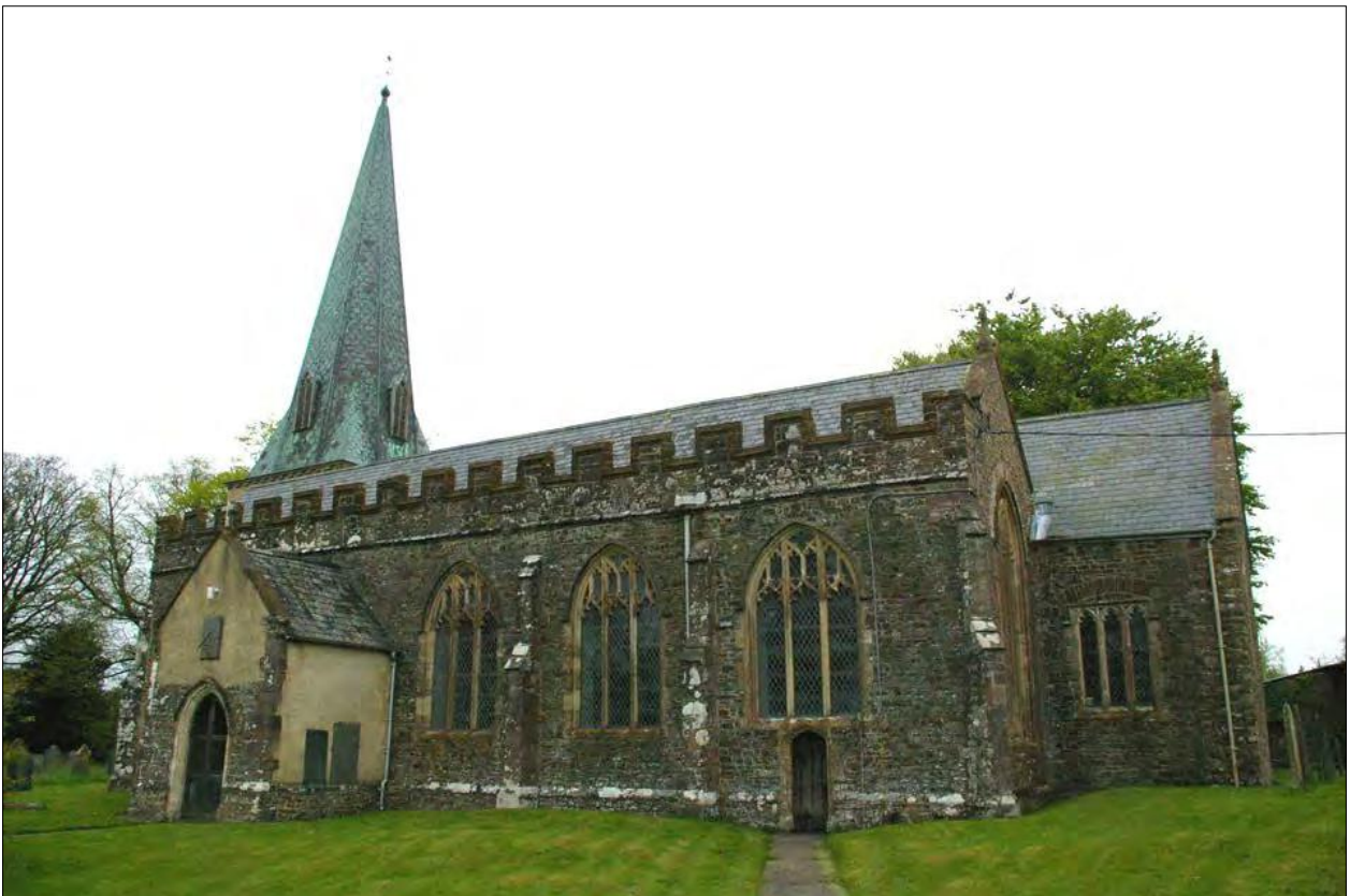
Kings Nympton Church, viewed from the south-east.
