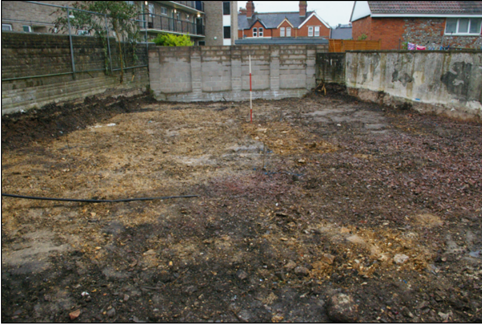
Figure 2: Excavated western half of site, viewed from the east (2m scale).
