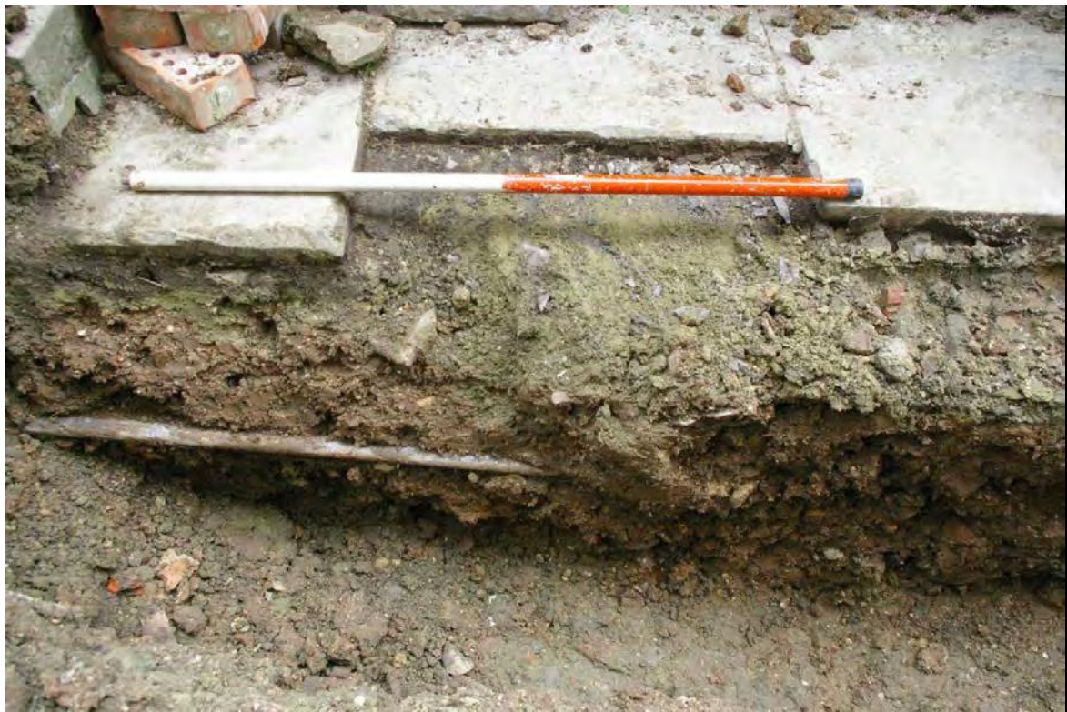
Figure 18: West facing section of Trench 04, showing modern water pipe [256]; looking north-east (1m scale).
