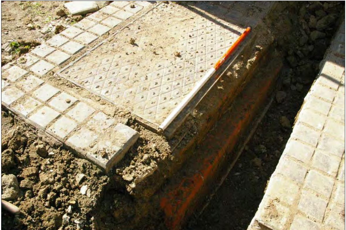
Figure 19: Shot of Trench 04, showing brick manhole chamber; looking north-west (1m scale).
