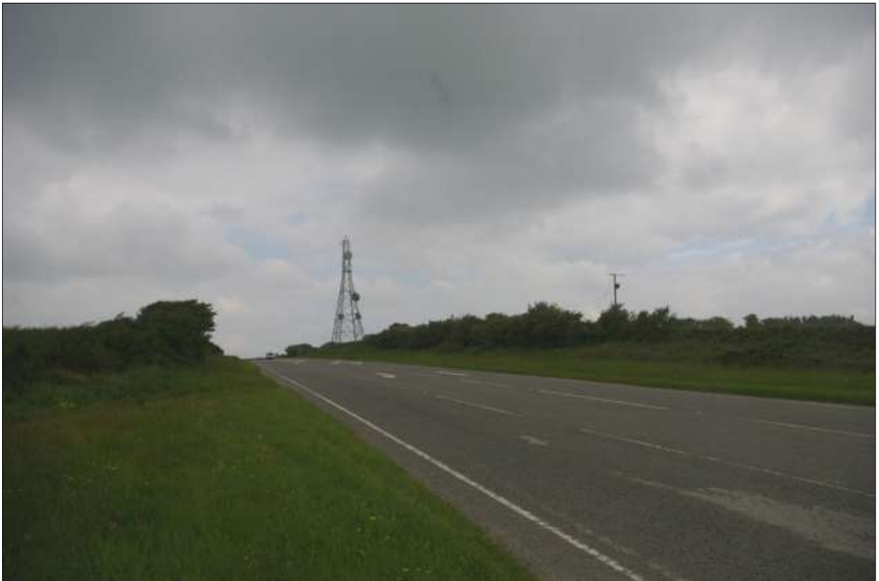
As above, looking back to Tich barrow and the substation immediately adjacent; from the south-west.
