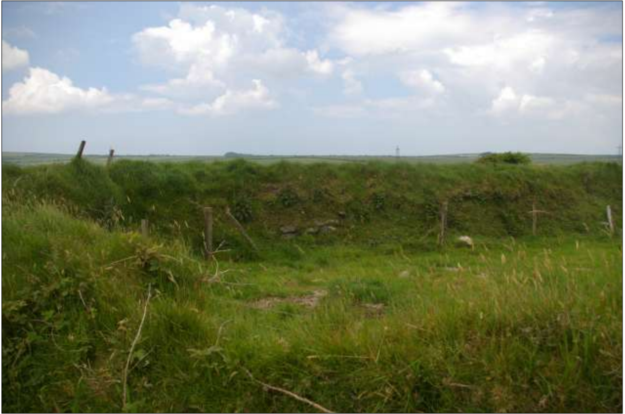
View of the structure of the hedgebank; from the east.
