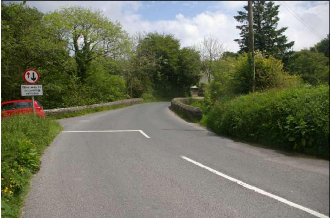
View of Slaughterbridge bridge, from within the base of the valley; from the west.
