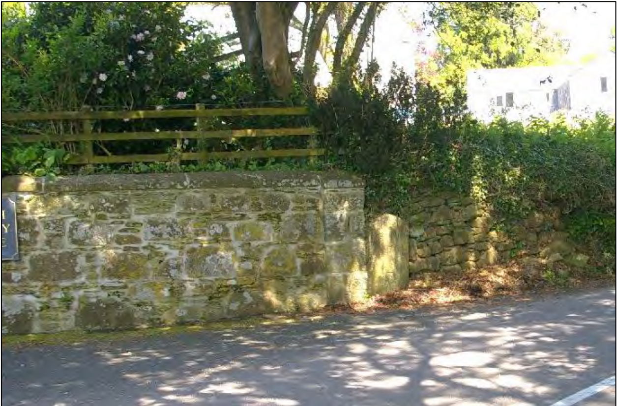
Milestone north of North Darley Farmhouse; an enclosed setting with tall hedgebanks. Viewed from the south-east.
