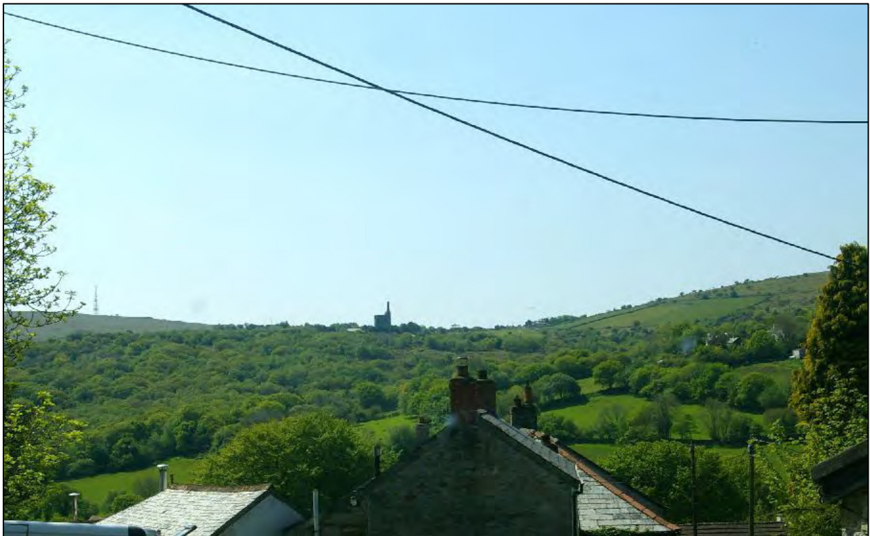
The Prince of Wales Engine House at the former Phoenix United Mine, showing how it dominates the landscape; from the north.
