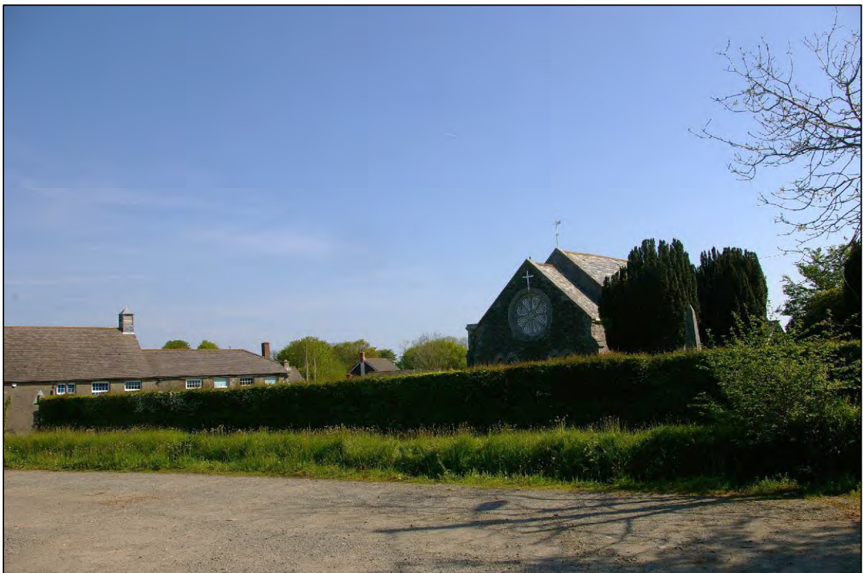
Methodist Chapel and School in Coad's Green, showing the village-based setting; from the south-west.
