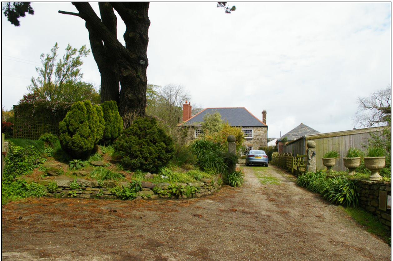
The former farmhouse at Great Pelean, viewed from the south. The proposed turbine would be located directly behind this building.
