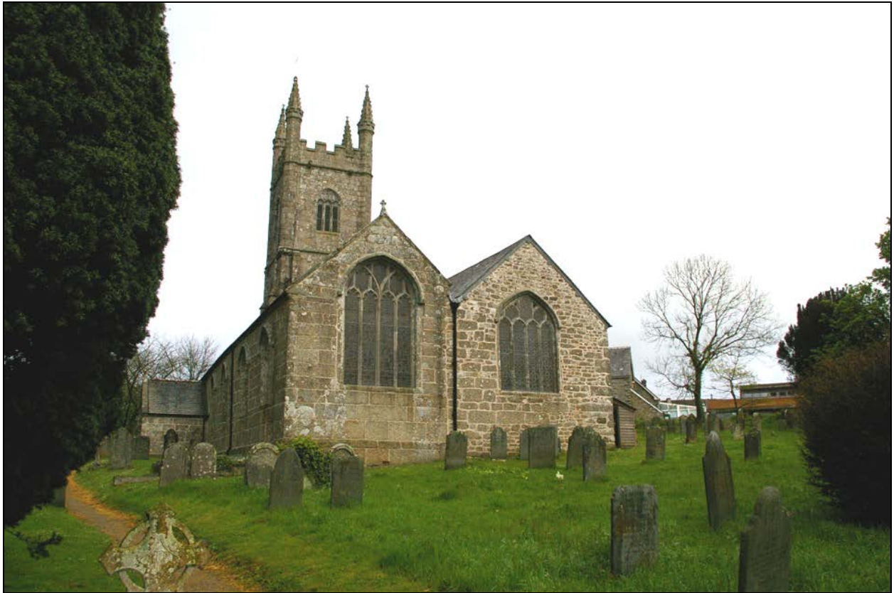
Lanlivery Church, viewed from the south-east.
