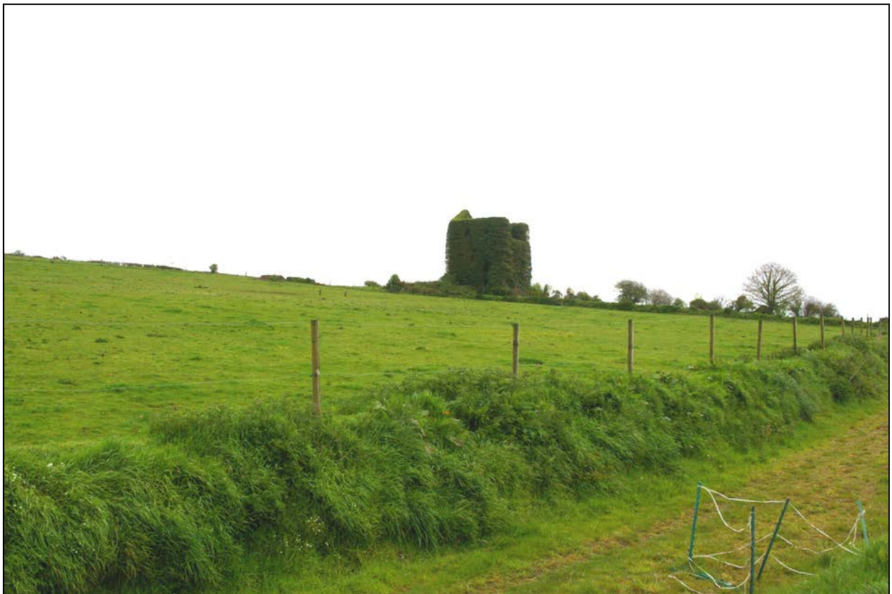
The ivy-covered Fowey Consols engine house, viewed from the south.
