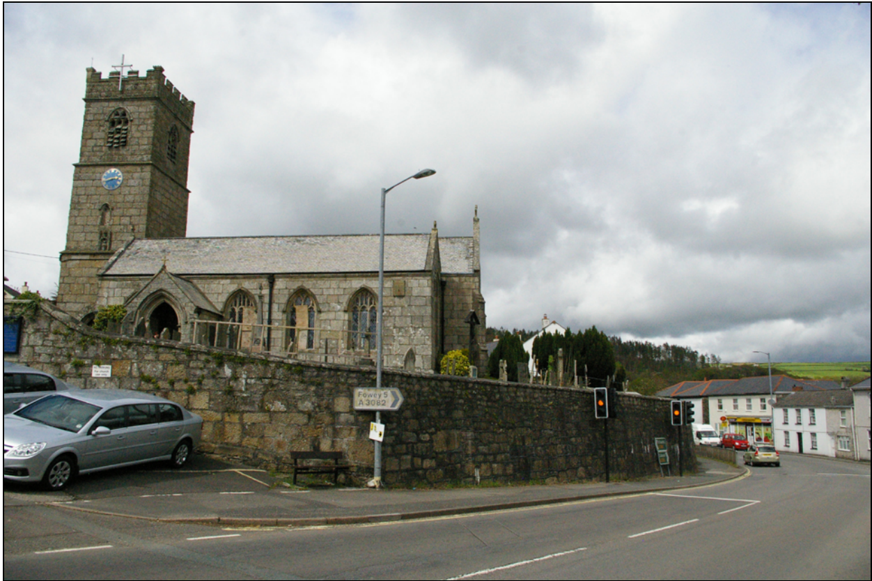
The church at St Blaise, viewed from the south.
