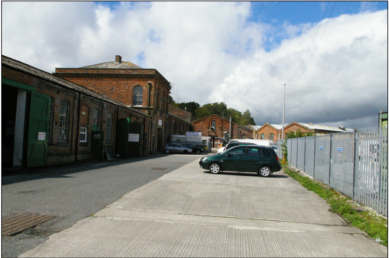
The Listed railway sheds at Par, viewed from the south.
