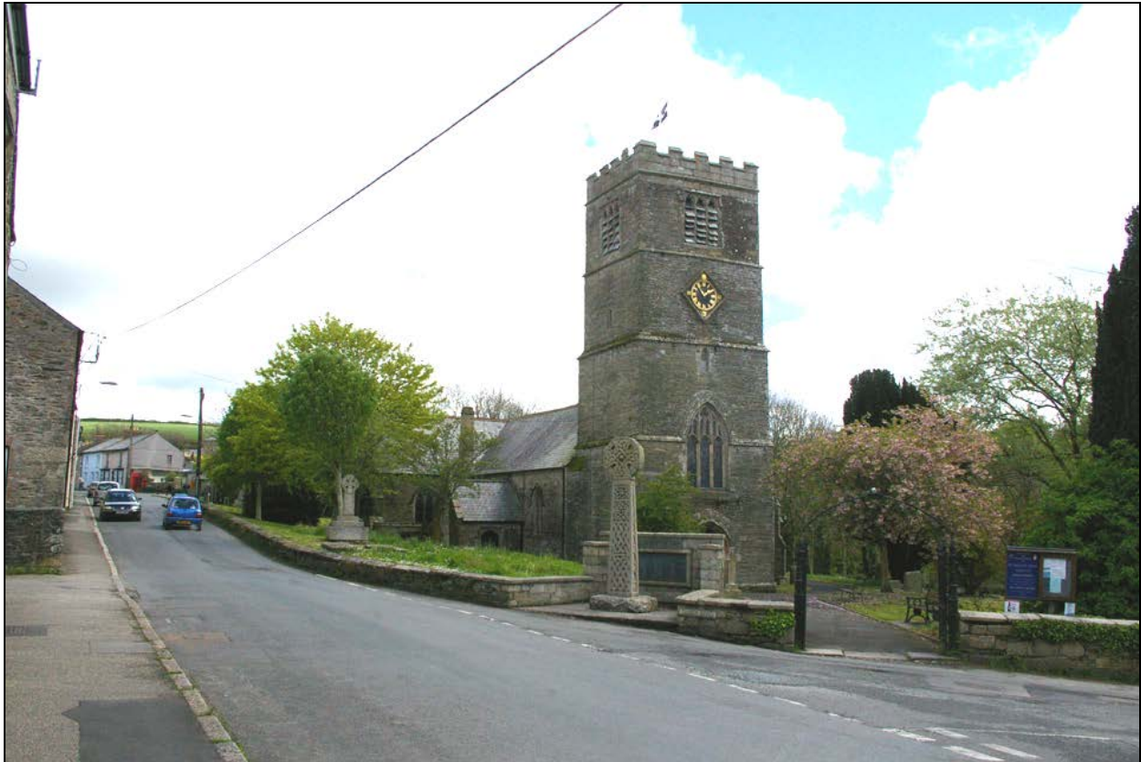
The tower of Tywardreath Church, viewed from the west-north-west.
