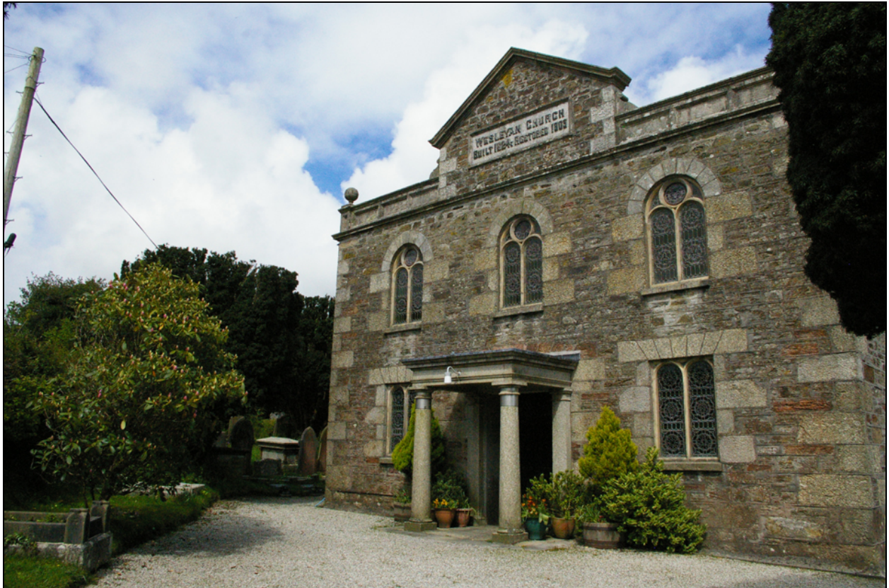
The Grade II* chapel at St Blazey Gate, viewed from the south-west.
