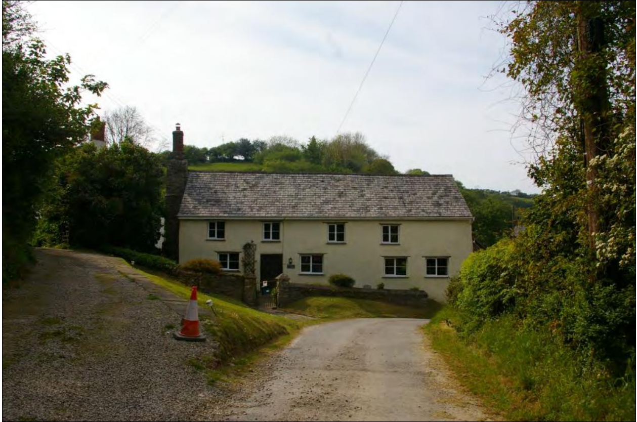
Dyers Farmhouse and Stanburys, set in the trees to the south, on a north-facing slope; from the east.
