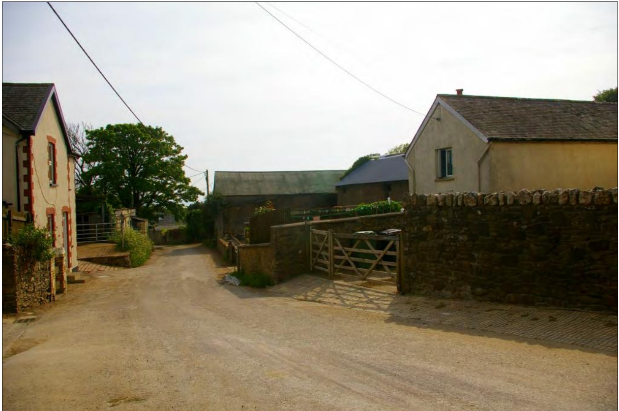
Boode Farmhouse and barns within the hamlet; from the north.
