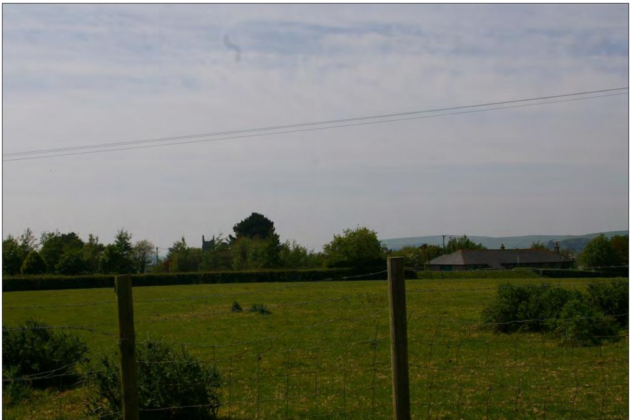
Landscape view of Heanton Punchardon church, set amongst the trees showing local blocking; from the east.
