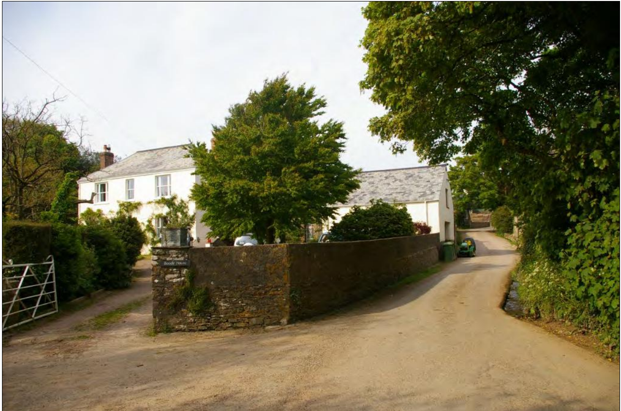
Boode House, set in the small hamlet; from the south-west.
