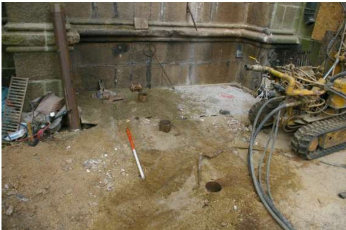
Figure 7: Post excavation plan view of piles 2-4
