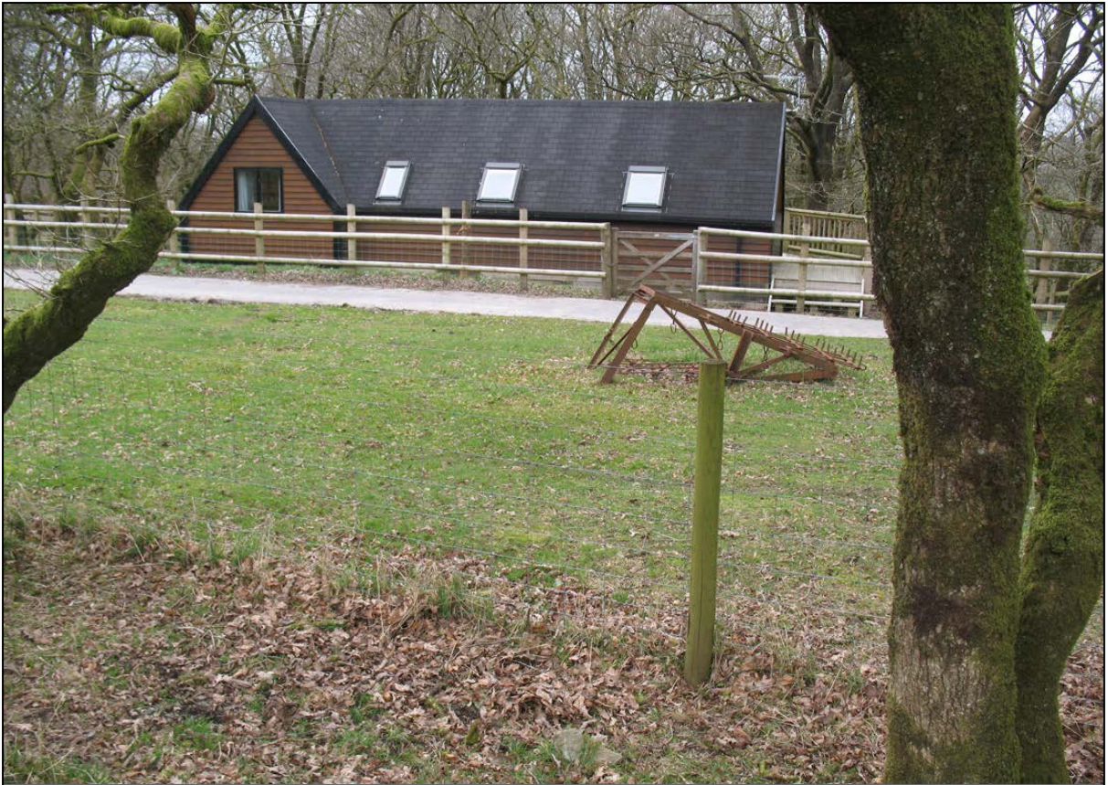
Figure 13: As above, detail of Lodge #1, from the south.
