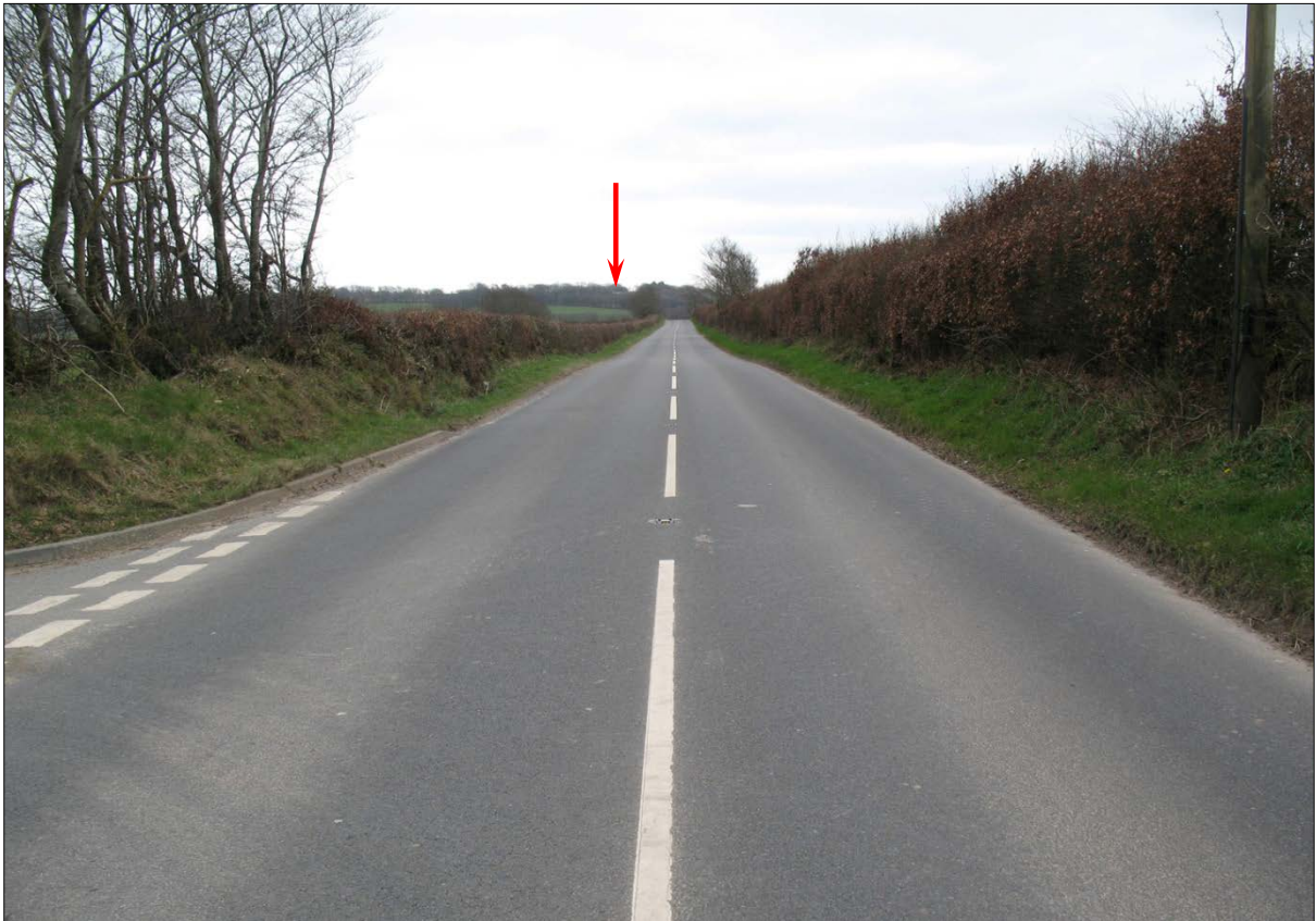
Figure 5: View down the A399 from the north [distance 1.5km] (the site is indicated).
