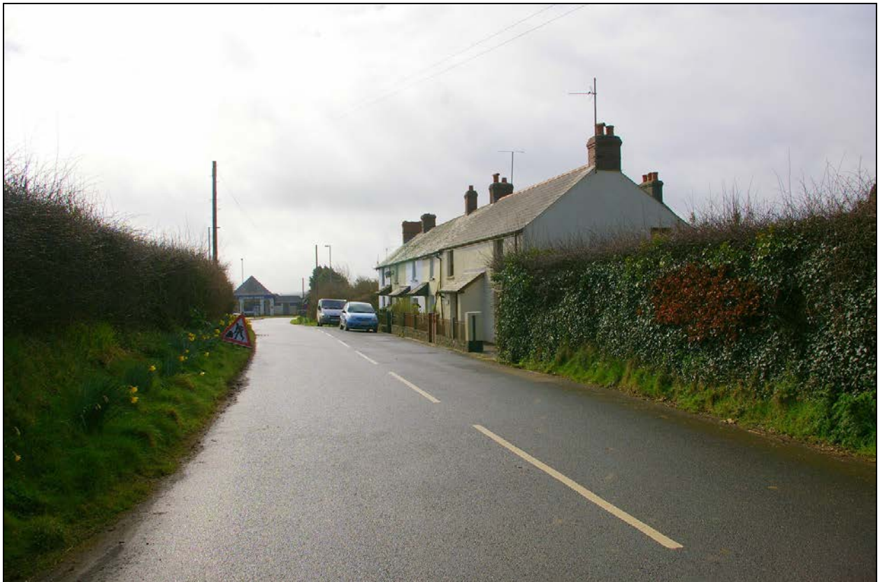
The row of cottages built within a section of the south-eastern outworks; from the north.
