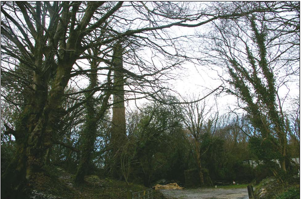
Bilberry kiln chimney and building remains; from the east.
