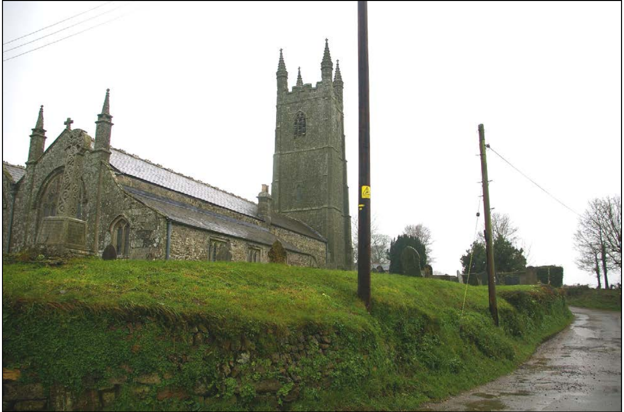
St Clements and additional Withiel medieval church remains in the churchyard at Withiel, showing the tall tower of St Clements; from the north-east.
