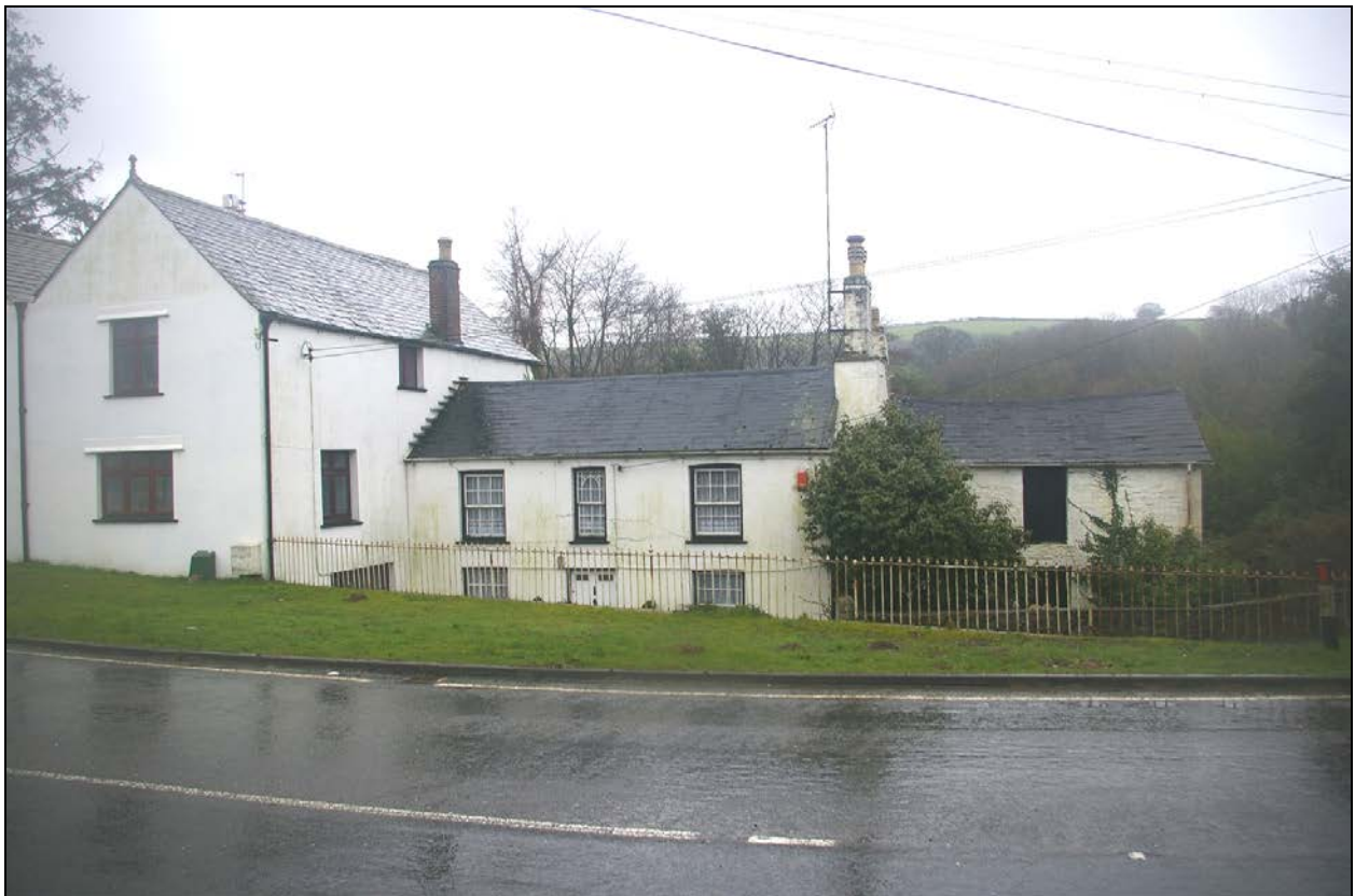
Dunmere Mill, east of Bodmin, on the A389 to Wadebridge; from the west.
