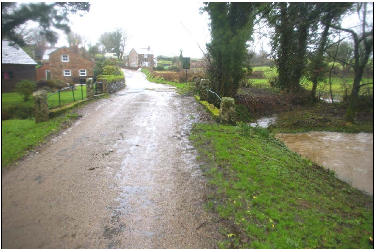
Tremorebridge and Tremore lodge behind, on the west facing lower slopes of the valley; from the west.
