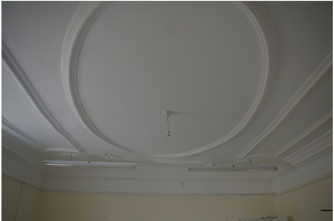
Figure 9: Room 5, the 17th century plaster ceiling; from the east.
