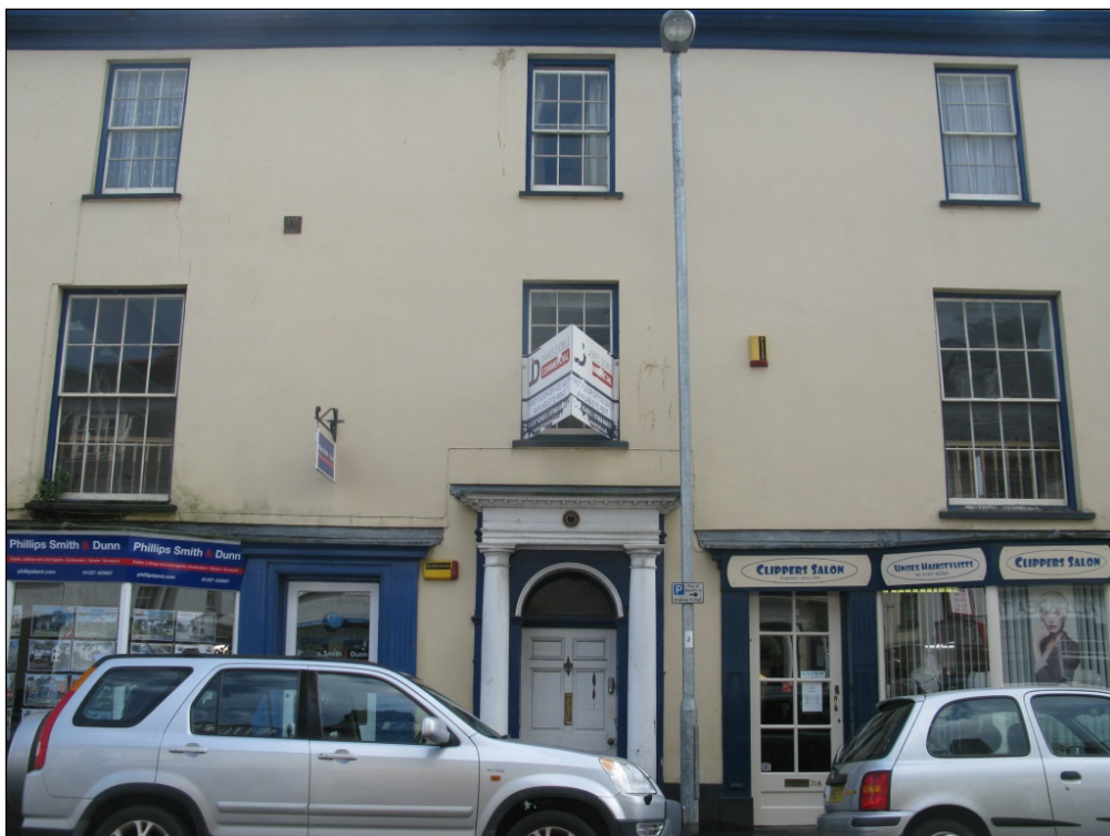
Figure 4: View from Bridgeland Street
