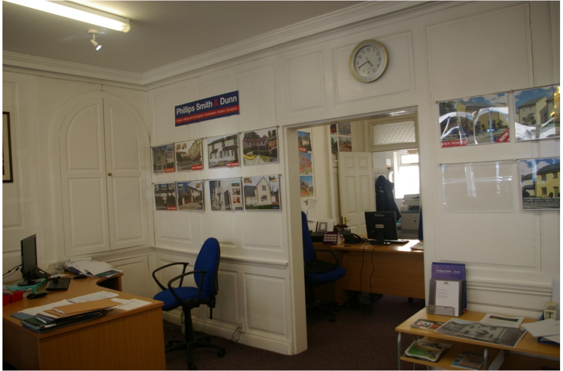
View of the 17th century panelling and alcove cupboard and cornice within the ground floor front reception room to the east, now a retail unit; from the north-west.
