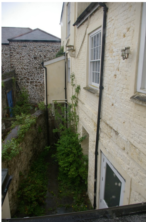
View into the rear yard from Room 3; from the north.
