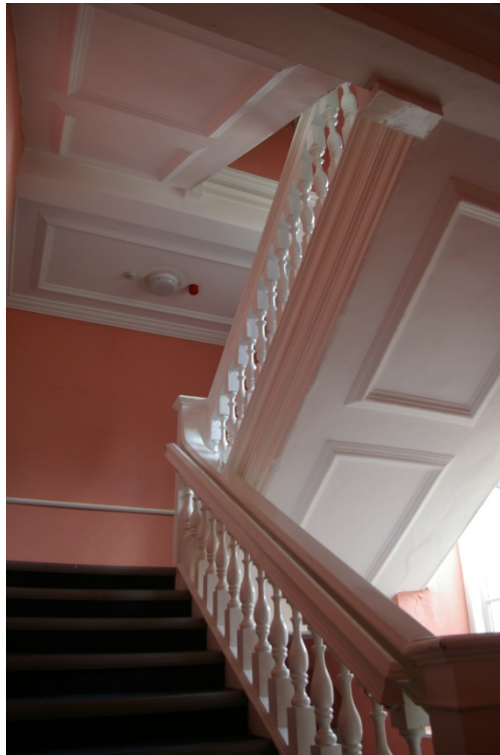
View back up to the first floor landing within the stair; from the half landing between the ground and first floors; from the north-west.
