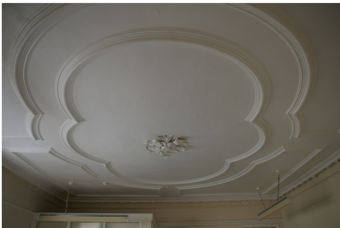
Room 2, the 17th century plaster ceiling; from the west.
