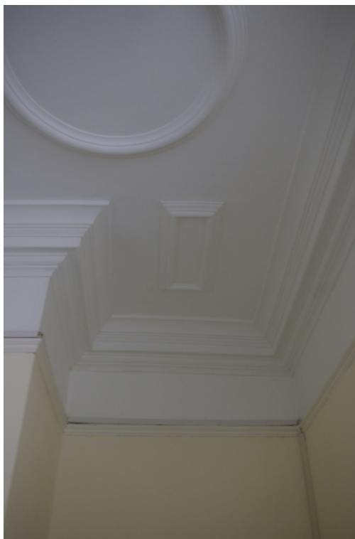
Room 5, the 17th century plaster ceiling; from the east.
