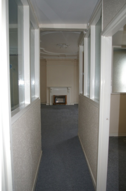
Figure 8: View through the open corridor between rooms 1 and 1A, back into room 2; from the east.
