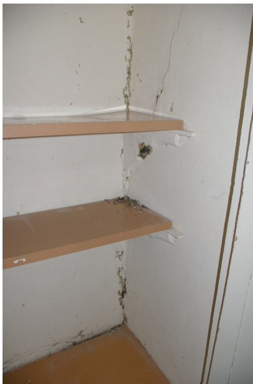
Detail of the decorative shelf stays within the cupboard in room 5; from the north-west.
