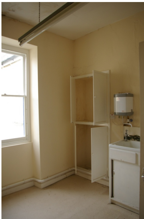
Room 3, showing the cupboard in the west wall and the south wall with large window opening; from the north-east.
