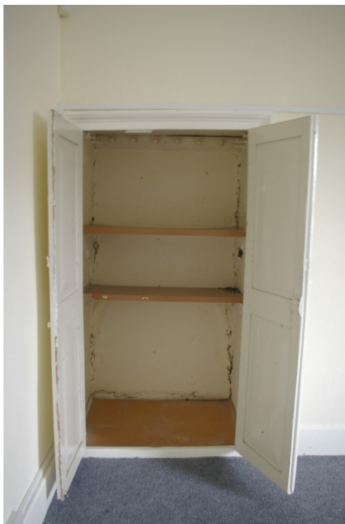
The cupboard in the east wall in room 5; from the west.
