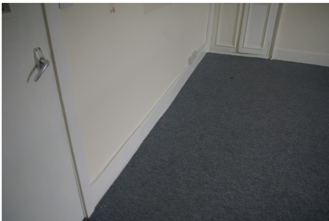
Detail of the deep but very simple skirting in room 5, along the north wall; from the south-west.
