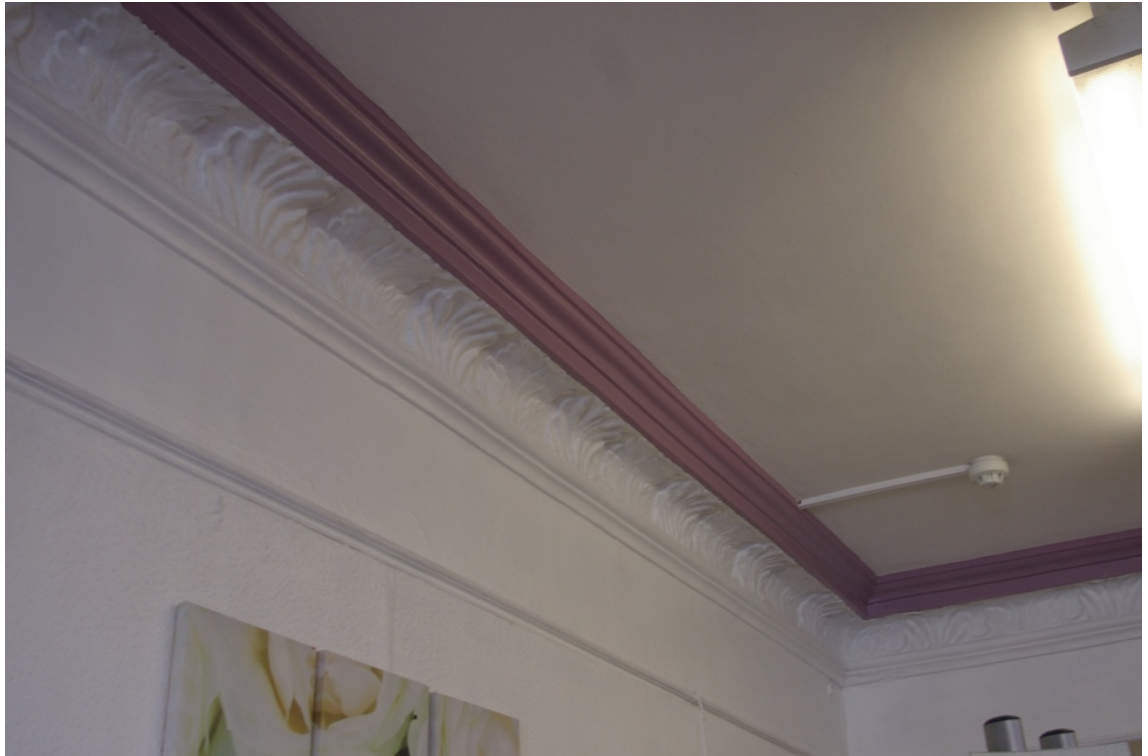
Figure 10: View of the high status 17 th century cornice in the front ground floor room to the west, now a retail unit; from the north-west.
